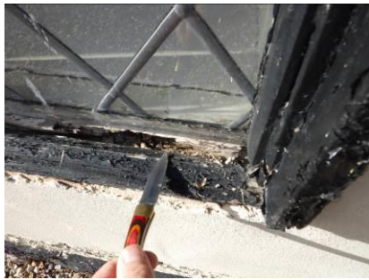
Knife test into timber
