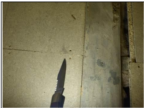
Floorboards screwed down
