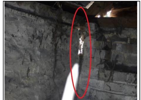
Rear wall opening up
