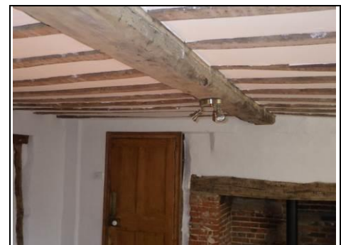
Spine beam in reception room one
