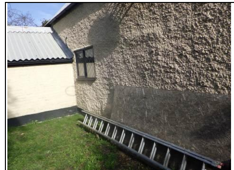
Cement render to right side of ancillary building
