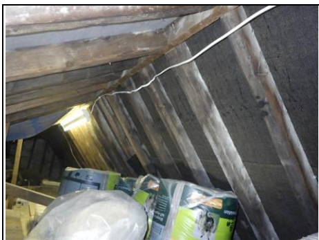
Main roof, mass of stored items
