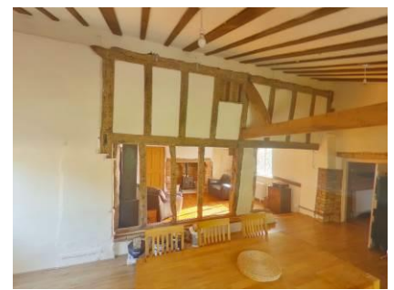
Timber structure in lounge/dining room
