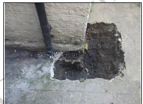
Trial hole to a corner of a property
