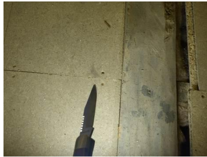
Screwed down floorboards limited our view
