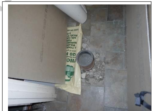
Soil and vent pipe in middle of cloakroom floor
