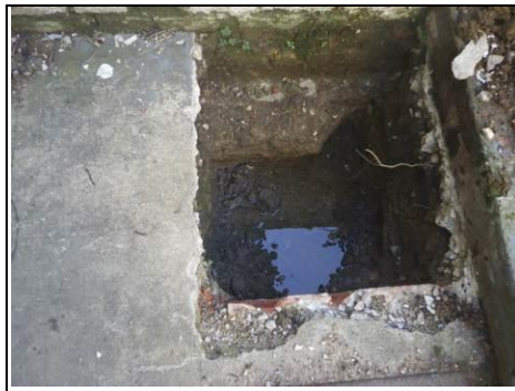
Trial hole showing foundations, water and tree roots
