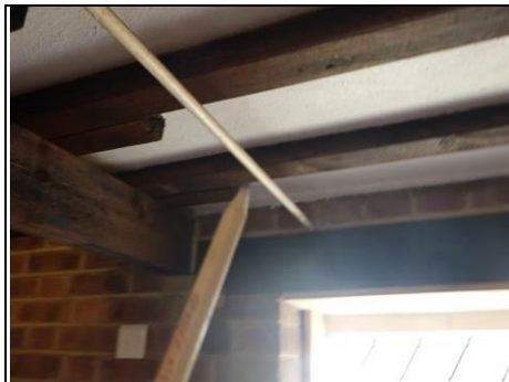
Tie bar running through internally
