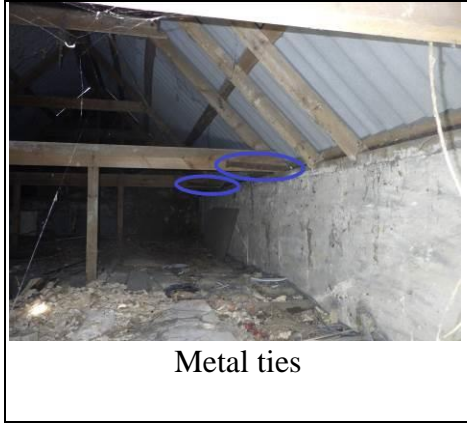
Close up of one of the ties holding the roof together
