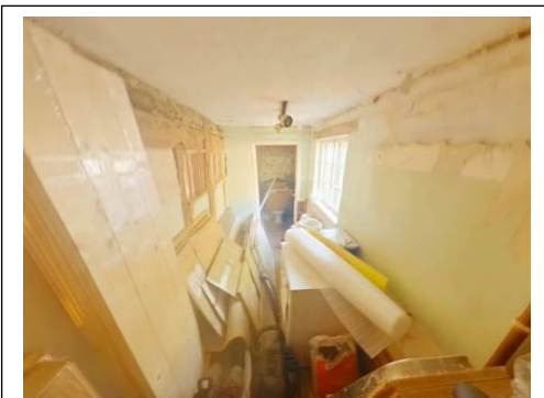
Cloakroom under construction
