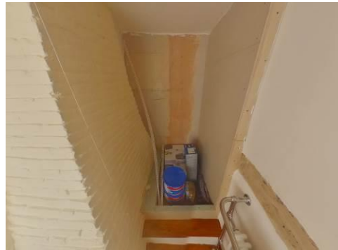
Unfinished en-suite shower room
