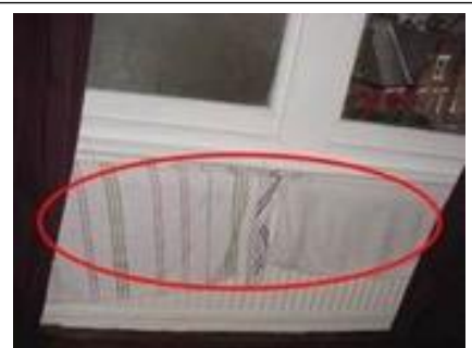
Drying washing on radiators can cause condensation
