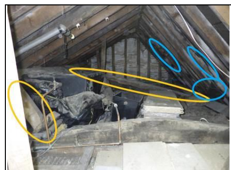
Dampness in roof space (blue ovals) and timbers supports added (yellow)
