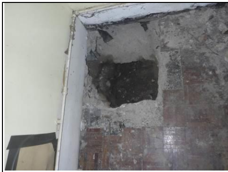
Looking inside a trial hole
