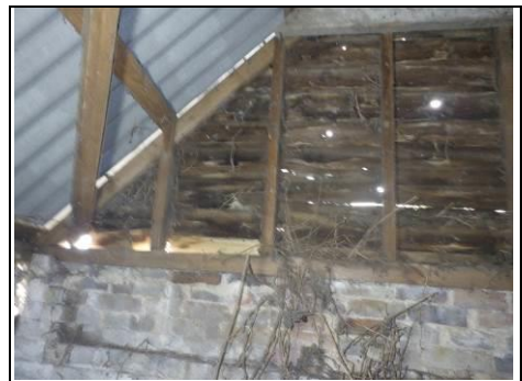
Rear gable end not viewable externally. This is the inside viewed from within roof, where vegetation is growing through
