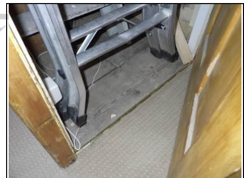
Timber joists run side to side
