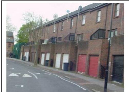
1960s properties built with concrete lintels that cause cold bridging
