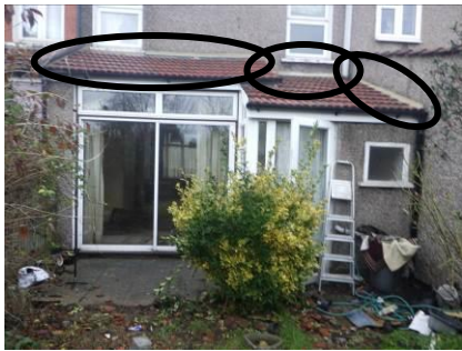
Rear single pitched roof with cement flashing
