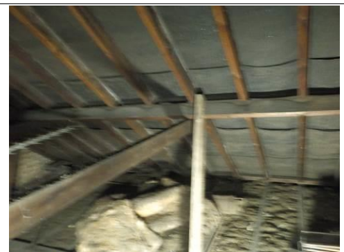
Timber roof purlins and strut support
