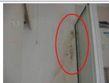
Condensation from a shower where nearby window was never opened
