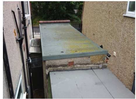
Garage flat roof with cement flashing and flat roofs behind
