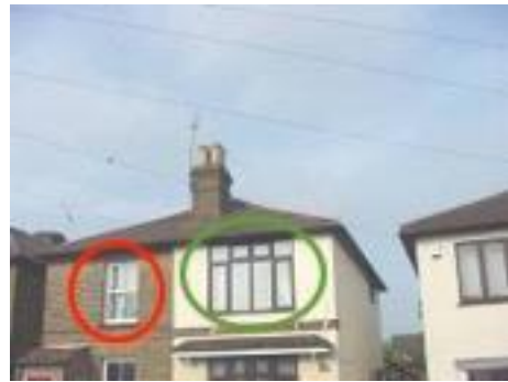
Victorian Property that has been modernised Red circle: original sash window Green oval: new large window that has been added
