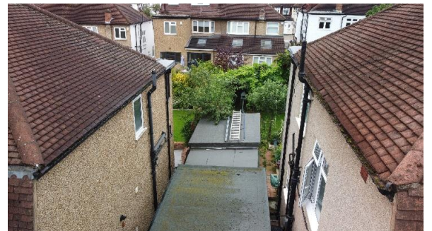
Shed roofs behind garage ~ Aerial View ~
