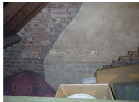
Front chimney viewed within roof space
