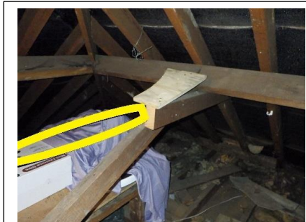
Cut cross brace
