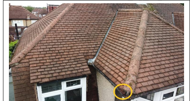
Tile in front gutter ~ Aerial View ~
