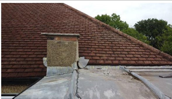
Bitumen repair to flat roof ~ Aerial View ~
