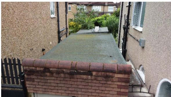
Garage roof ~ Aerial View ~
