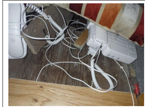
Floorboards visible under the stairs
