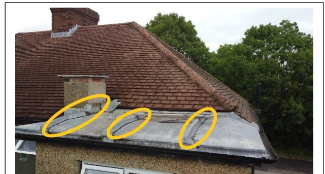
Rear flat roof tarred on rolled joints ~ Aerial View ~
