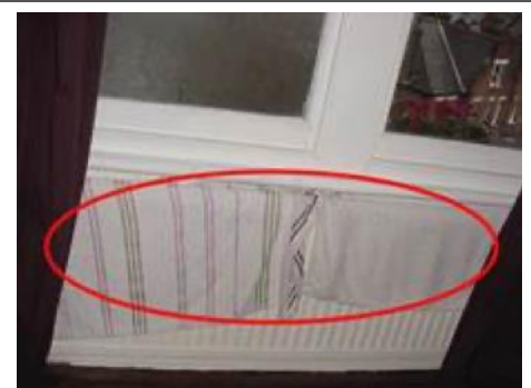
Drying clothes on a radiator can cause condensation
