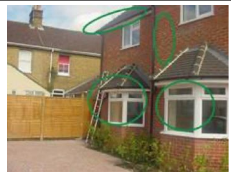
Double glazed windows and loft insulation in a modern property
