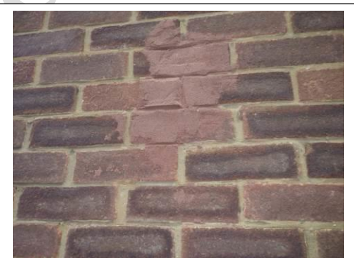
Repairs to the brickwork/blocking up of an opening
