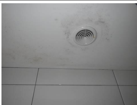
Bathroom extract with black mould around it
