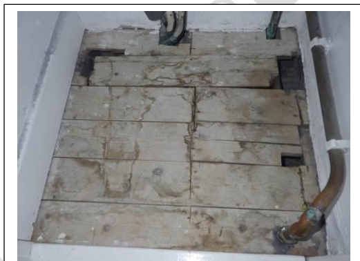
Floorboards in front right bedroom
