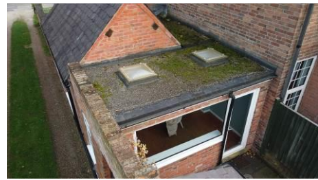
Stretcher bond brickwork to rear kitchen extension
