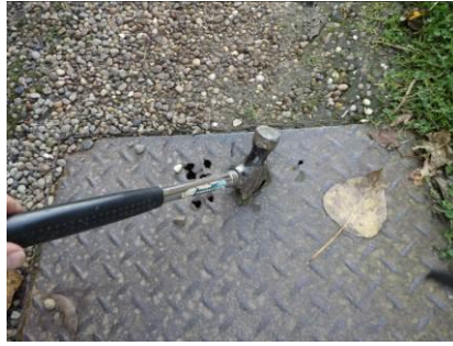
Manhole Two to middle, again we were unable to open
