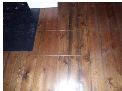
Are of floor in dining room which looks as though it has been opened up before
