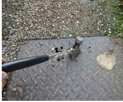
Manhole two to middle
