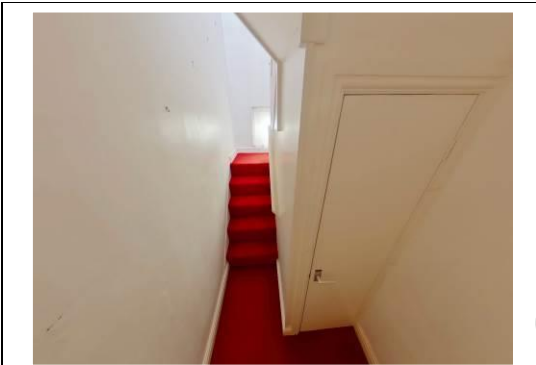
Landing and Stairs to room in roof
