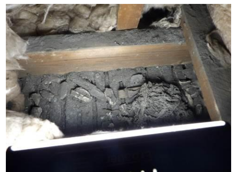
Lath and plaster visible within roof space
