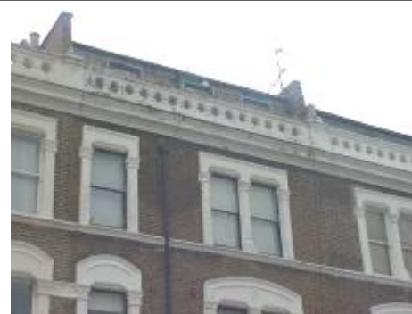
Classic Victorian Sliding sash windows where they have managed to put in one pane of glass
