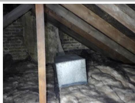
Old cast iron water tank
