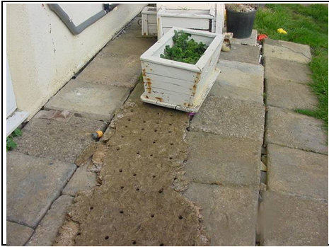
Uneven paving slabs
