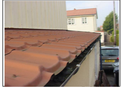
Single storey extension pressed metal tiles
