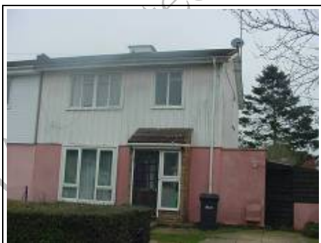
Painted cladding to non-traditional property
