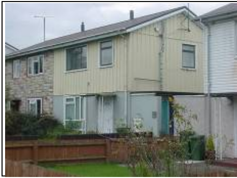
BISF property with metal profile sheet roof (has asbestos roof been removed or has it been overclad?) and metal profile sheet at first floor level and render at ground floor level and older style double glazed windows. .
