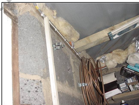
Blockwork to left lean-to
