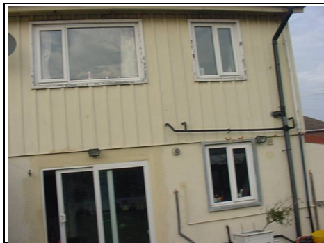
DIY standard pipework
