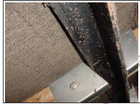
Some fixings replacements/repairs to a non-traditional house
