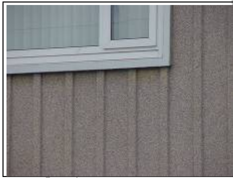
Close up of cladding on non-traditional house
