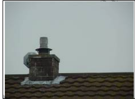
New chimney on a non-traditional house
