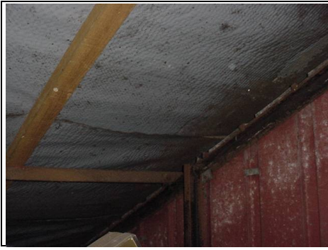
Plastic underlayer to main roof
