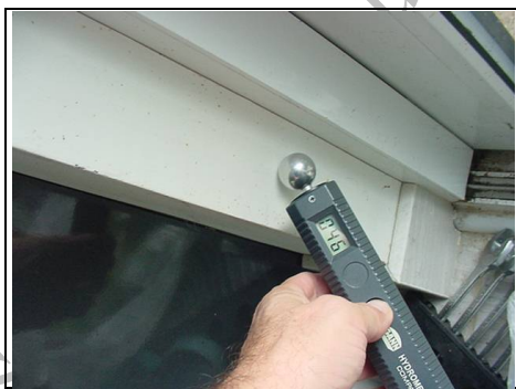
Testing for rising damp
