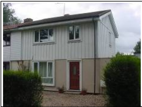
How vertical tiling and new windows can considerably change the look of a property but underneath it is still a metal framed building
