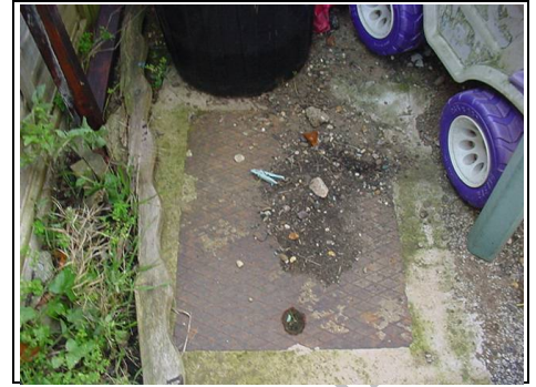
Rear left manhole
