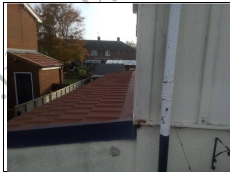
Single storey extension
