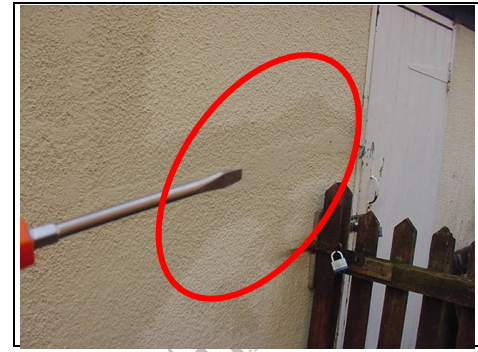
Repaired cracks on left side
