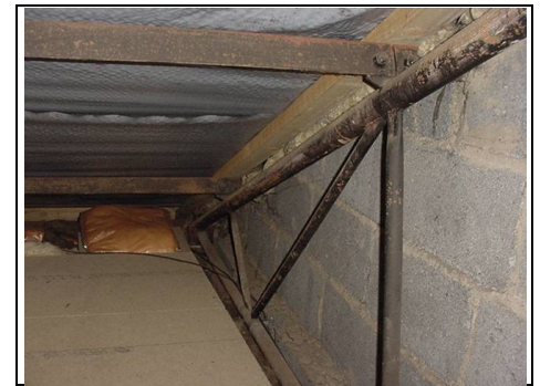
Blockwork fire wall
