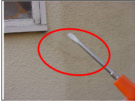
Repaired cracks on left side
