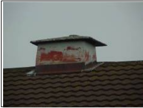
Asbestos original chimney non traditional house
