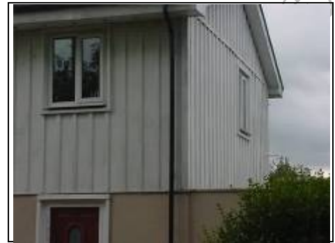
Example of metal cladding on a BISF house (Not your property)
