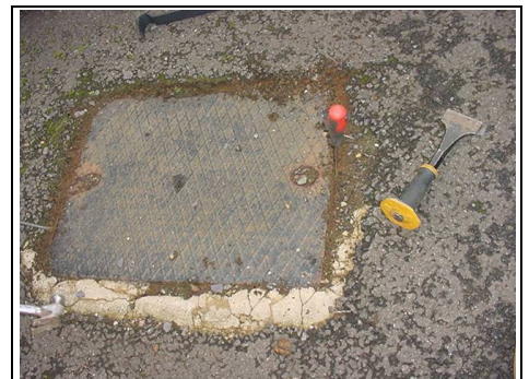
Front left manhole
