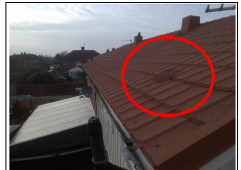
Felt repair where internal soil and vent pipe removed
