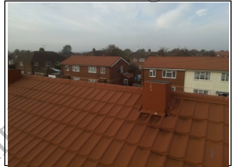
Roof and chimney
