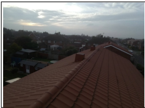
Pressed metal roof
