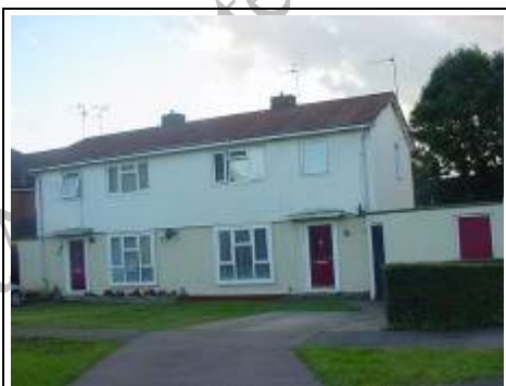
Plastic cladding has been put on top of the property
