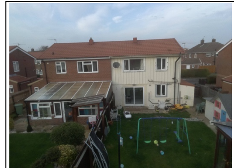
Adjoining semi-detached property brick to rear ~ Aerial View - 360 Photo ~
