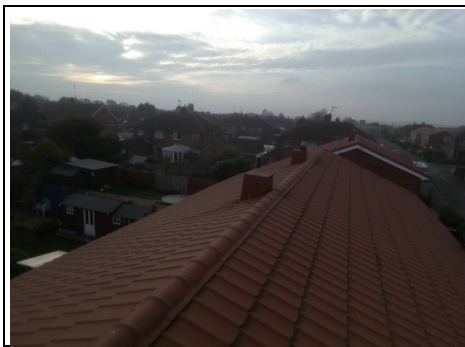
Pressed metal roof
