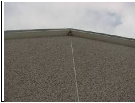
Jointing to a non-traditional house
