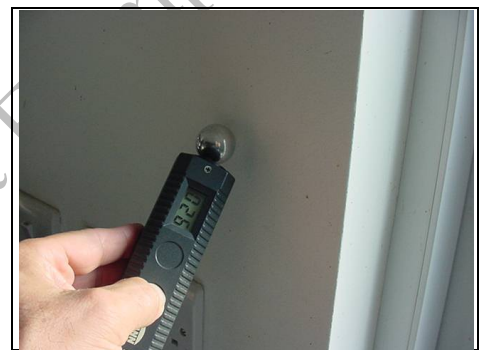
Testing for lateral dampness
