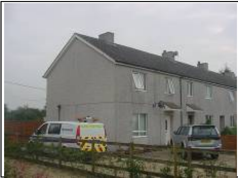
Large panel concrete non-traditional house
