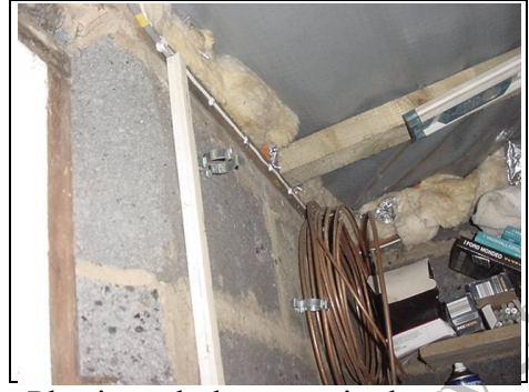
Plastic underlayer to single storey extension roof
