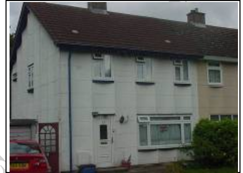
Non traditional house mainly asbestos
