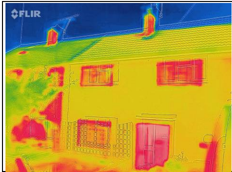
Front of property showing heat coming through windows and door
