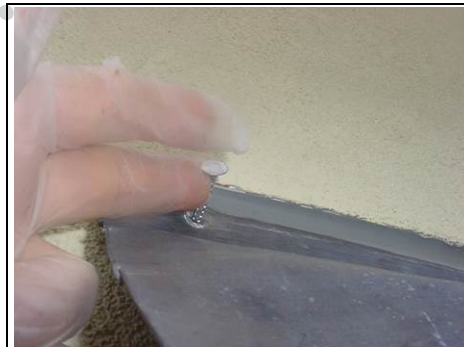
Flashing nailed into the external wall insulation (EWI)
