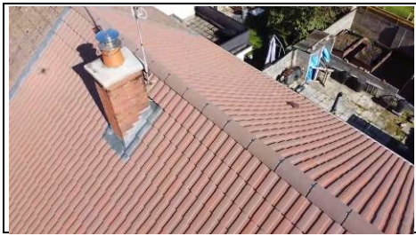
Main roof and chimney ~ Aerial View - 360 Photo ~
