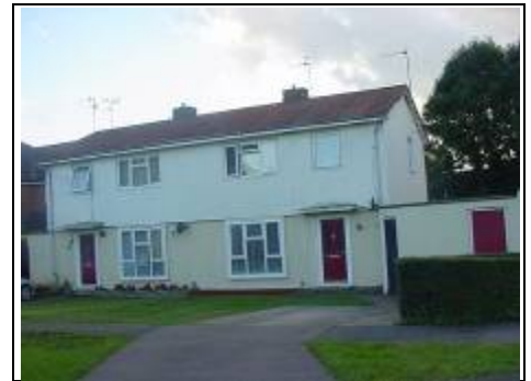
British Steel frame house (BISF)
