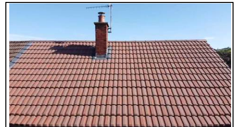
Main roof Aerial view – 360 photo
