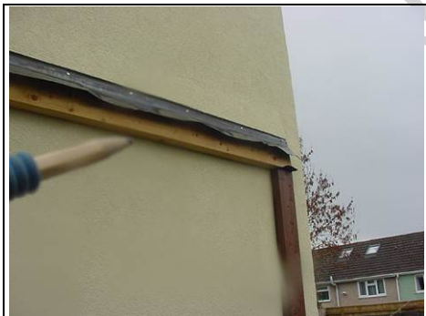
Wall posts for lean-to
