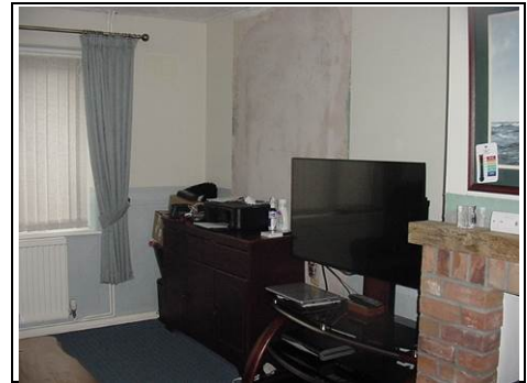
Lounge (where door has been blocked up)
