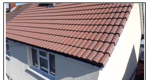
Rear roof ~ Aerial View - 360 Photo ~
