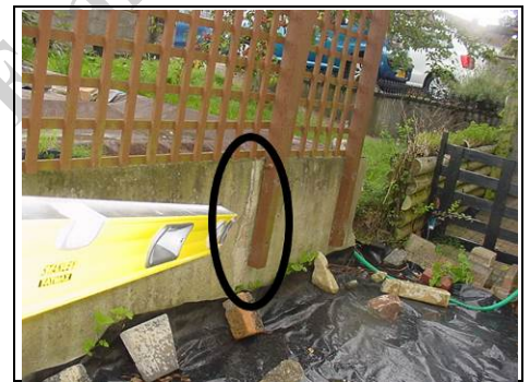
Crack in left side retaining wall
