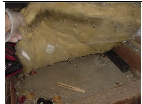
Lifting insulation
