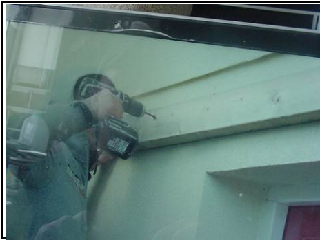
Rate Avon fixing the wall plate
