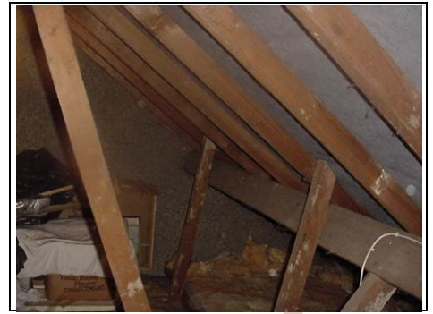
General view of roof
