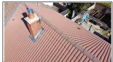
Dry ridge on roof Aerial view – 360- photo
