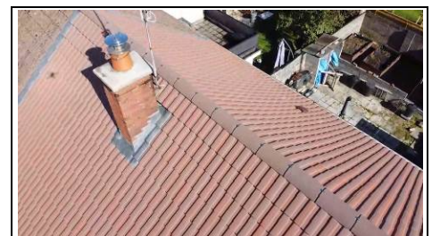
Dry ridge on roof Aerial view – 360- photo
