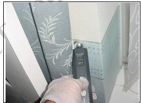
Testing for lateral dampness
