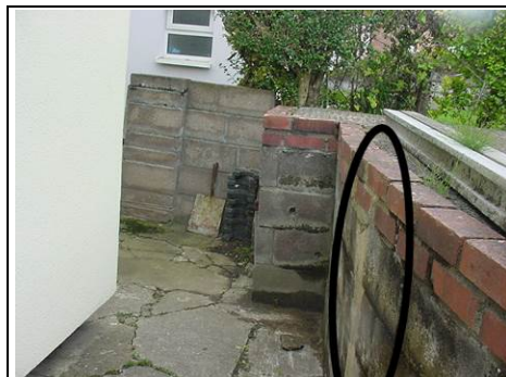
Retaining wall around drop from front driveway
