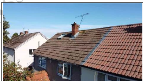
Join with next door's roof ~ Aerial View - 360 Photo ~
