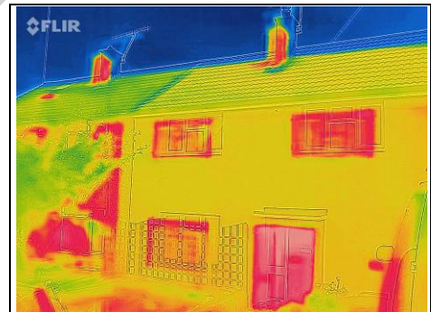
Thermal imaging of front of property
