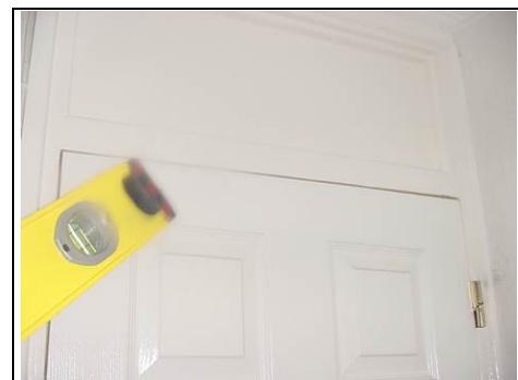
Checking for alignment on door in front left bedroom
