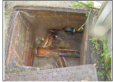
Manhole to right corner of property
