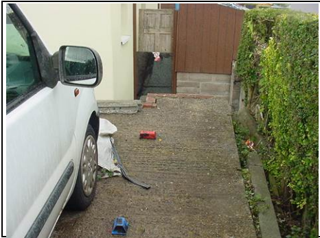
Driveway drops away top right hand side
