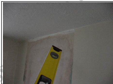
Blocked up door
