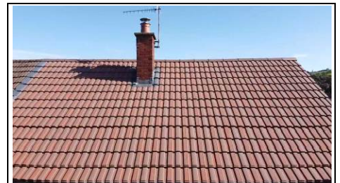
Main roof Aerial view – 360 photo
