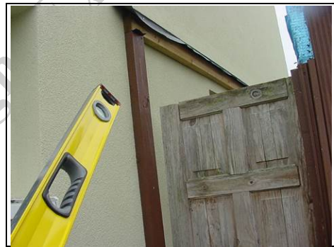
Where the lean-to should be
