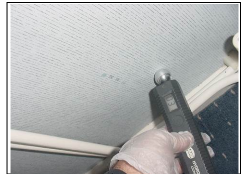
Testing for rising damp
