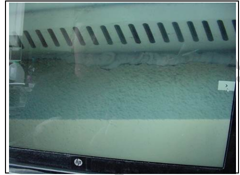
Damaged fascia board where mastic has been added
