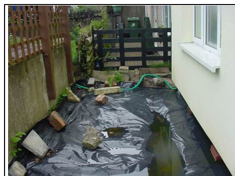
Polythene sheet/tarpaulin at front by base of the wall
