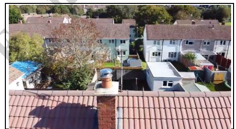
Chimney Aerial view – 360 photo
