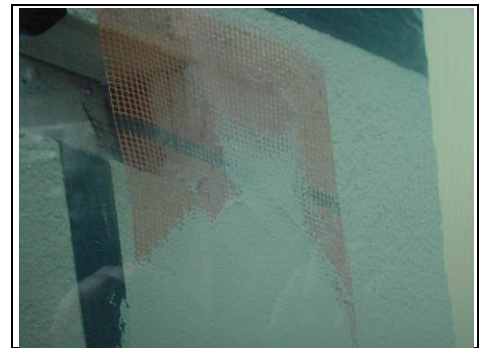
Red reinforced mesh in use with an applied coating on it
