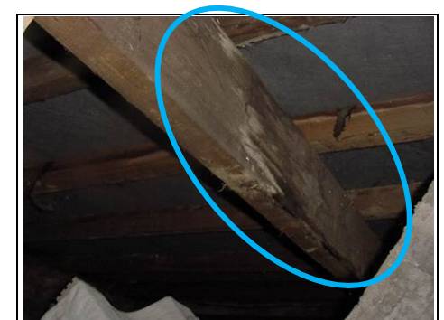
Dampness to is the purlin and common rafters, we believe from the chimney
