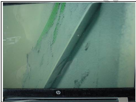
The forming of the drip detail on the side of the property
