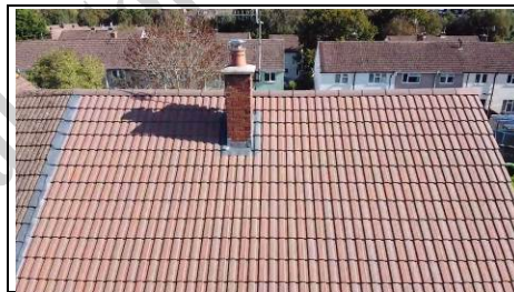
Chimney ~ Aerial View - 360 Photo ~
