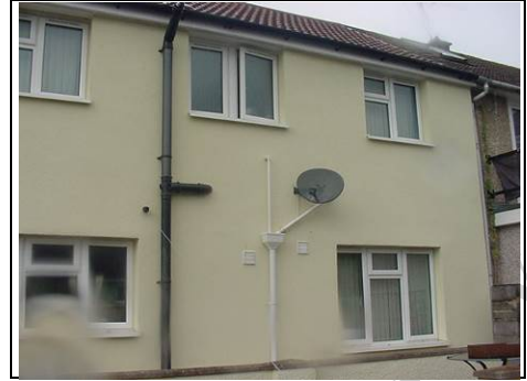
Soil and vent pipe to rear
