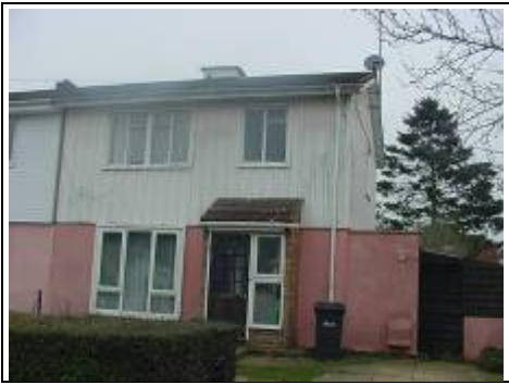
Painted cladding to non-traditional property
