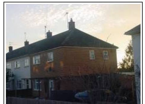
Brick cladding and other alterations make a non traditional house mortgageable
