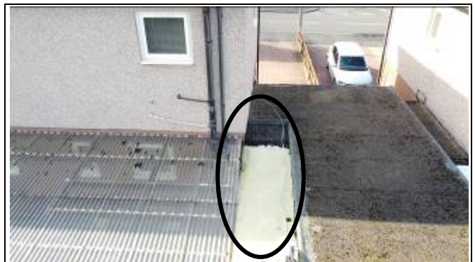
Outbuilding roofs, link corridor roof (black oval) ~ Aerial View - 360 Photo ~
