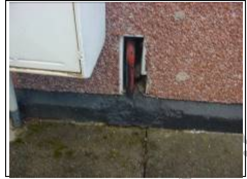
Insulation cut around pipe
