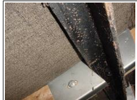
Some fixings replacements/repairs to a non-traditional house
