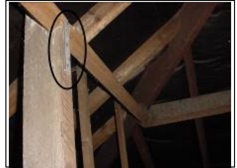
Metal brackets added to roof
