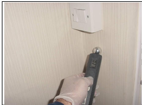
Testing for lateral dampness
