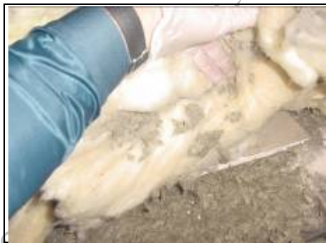
Layers of insulation
