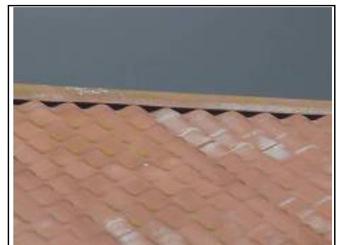
Metal cladding roofs
