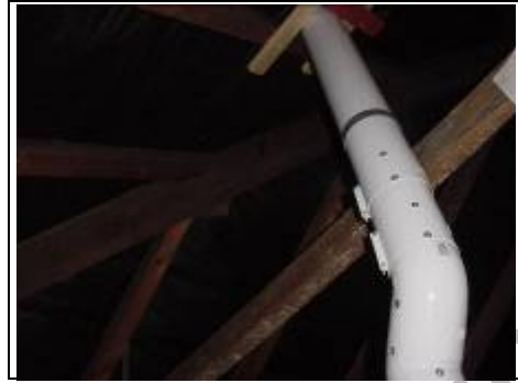
Vent from boiler in roof space
