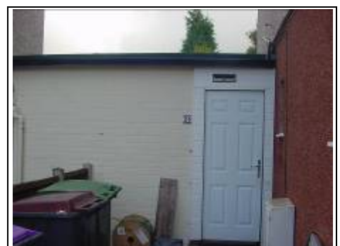
Access to outbuilding
