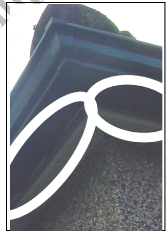
Vent to soffit
