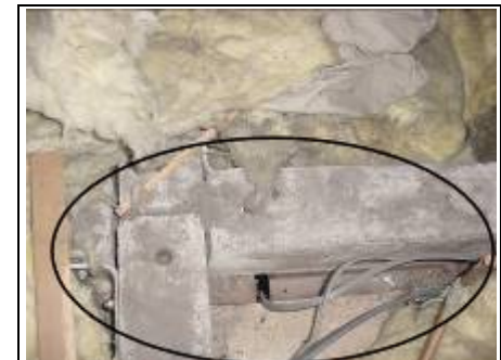
Close up of concrete frame
