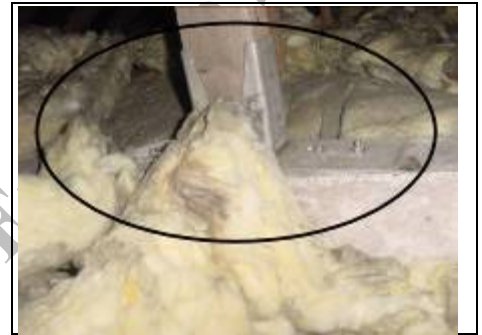
Metal bracket fixing timber to concrete frame
