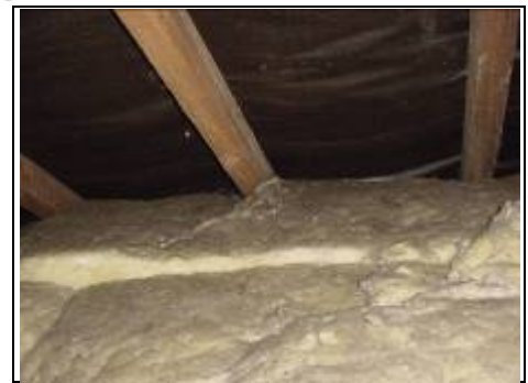
This photo shows the common rafters (the ones that form the pitch of the roof) and the dark area between is the underlayer.
