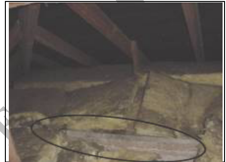
Concrete frame visible within roof
