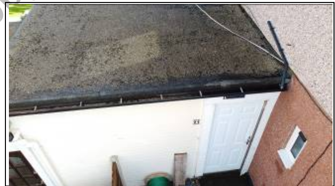
Wastepipe into metal gutter ~ Aerial View - 360 Photo ~
