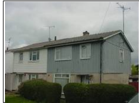
Asbestos roof on BISF house
