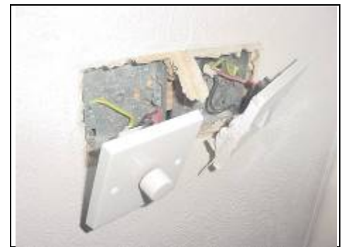
Removing electric points to view construction
