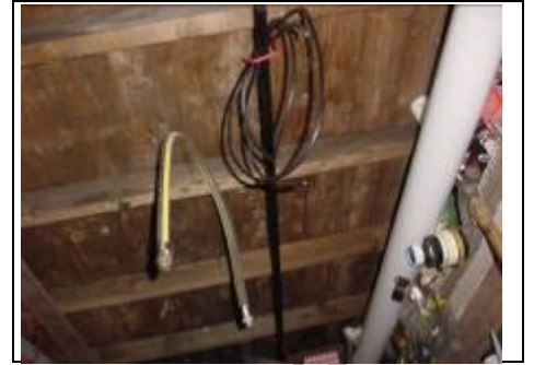
Shed has original boarded roof
