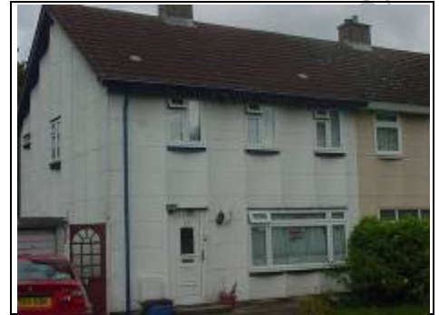
Non traditional house mainly asbestos
