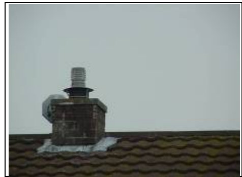
New chimney on a non-traditional house
