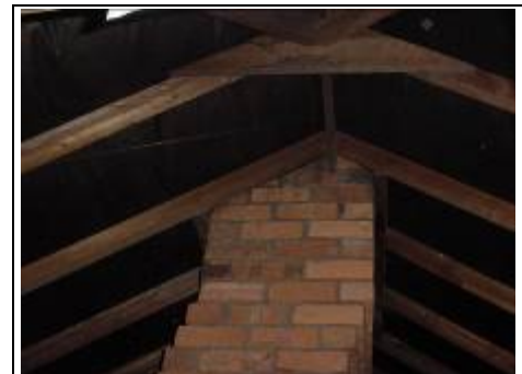
Chimney within roof space
