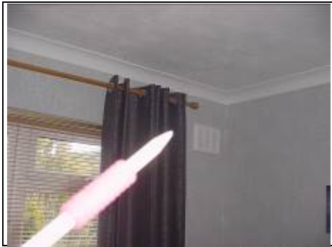
High level airbrick in rear right bedroom
