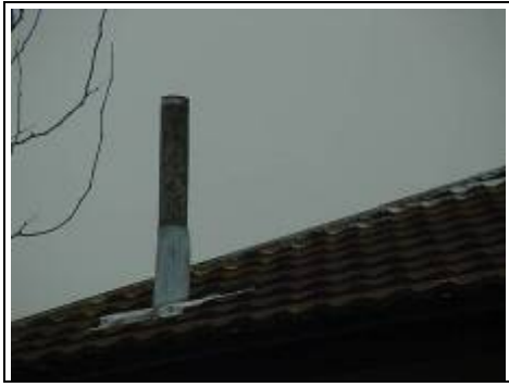
Original asbestos soil and vent pipe on a non-traditional house
