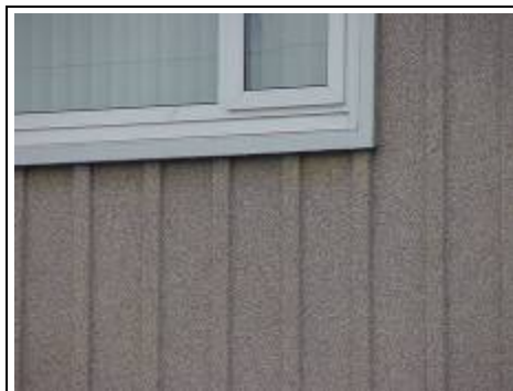
Close up of cladding on non-traditional house
