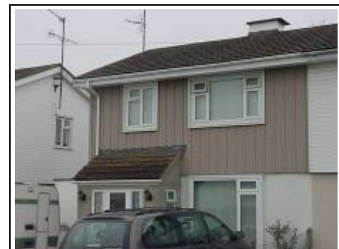
Non-traditional metal frame house
