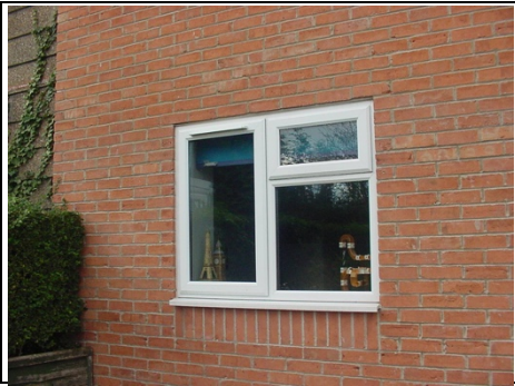
Plastic double glazed window with trickle vent
