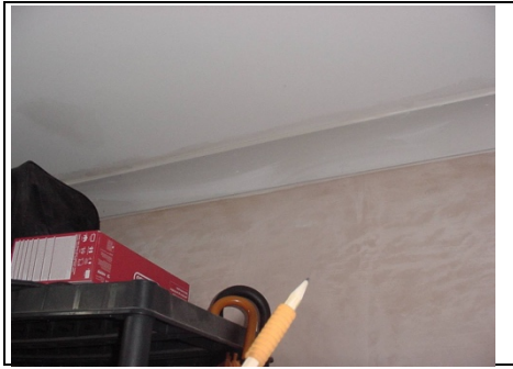
New plaster in storage room
