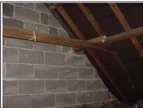
Blockwork to gable
