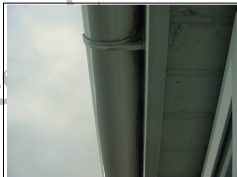
Soffit board
