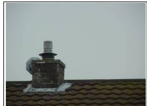
New chimney on a non-traditional house
