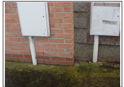
Engineering bricks to base
