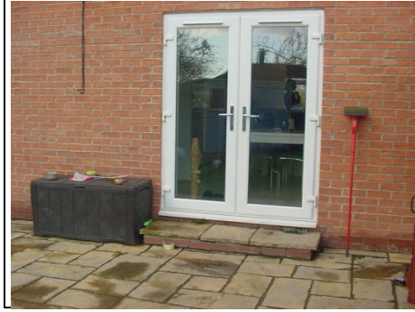
Trickle vent on kitchen door
