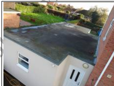
Flat roof ~ Aerial View - 360 Photo ~
