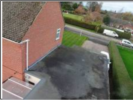
Left flat roof
