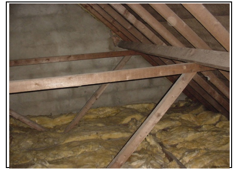
General view of inside of roof
