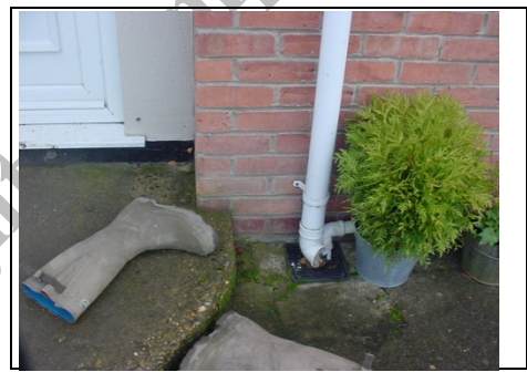
Downpipe discharges into gully
