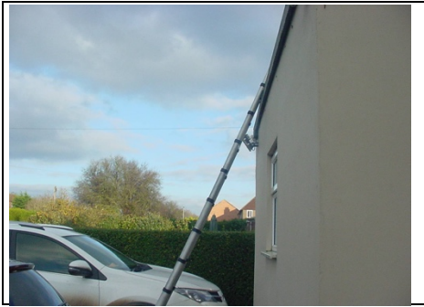
No detailing to roof
