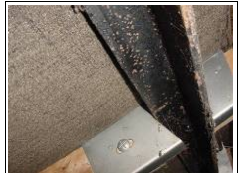
Some fixings replacements/repairs to a non-traditional house
