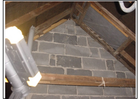
Chimney removed to left
