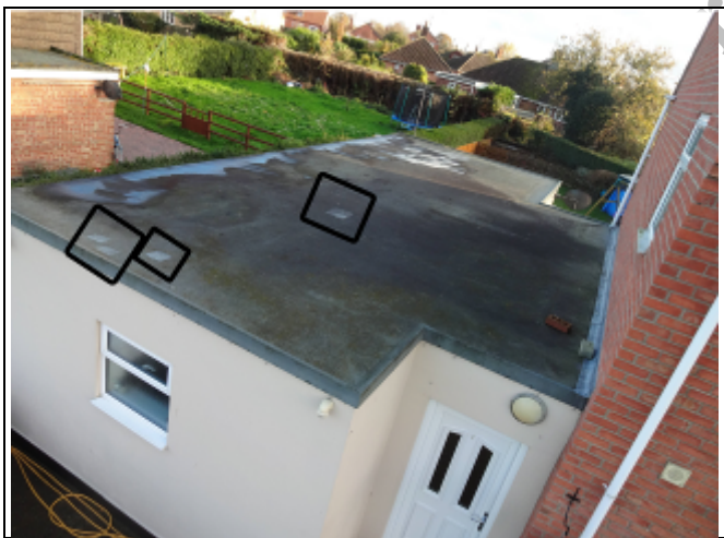
Patch repairs to GRP roof
