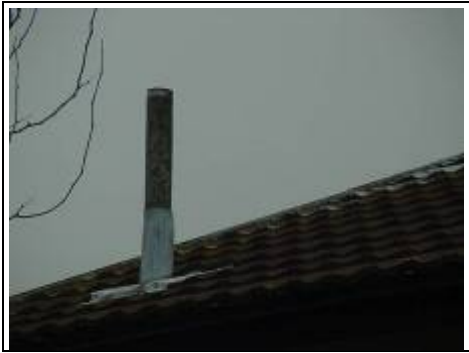
Original asbestos soil and vent pipe on a non-traditional house
