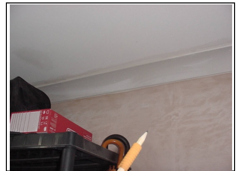
New plaster in store room
