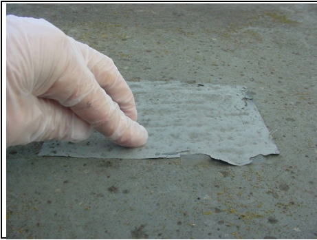
Close up of patch repair
