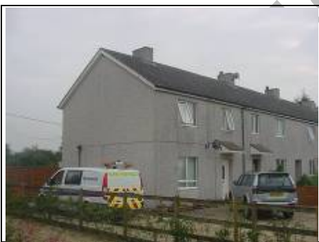
Large panel concrete non-traditional house
