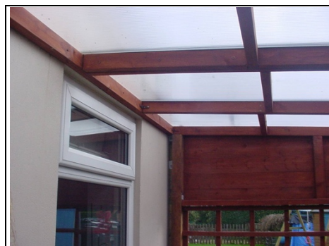
Polycarbonate roof
