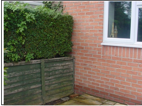
Stretcher bond brickwork with engineering bricks to lower two courses
