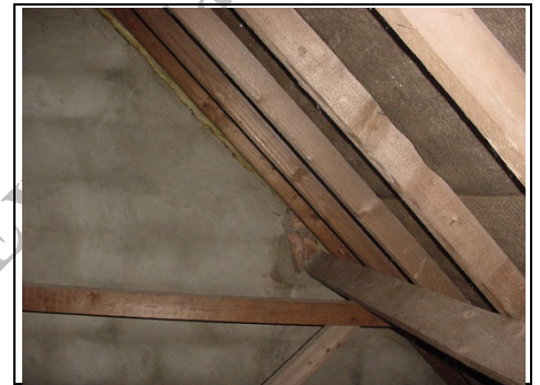
Purlins and common rafters
