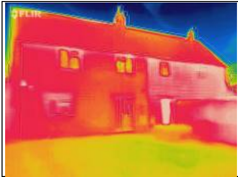
This property and neighbours – Airey house compared with traditional brick
