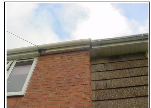
Join at front roof level with next door property
