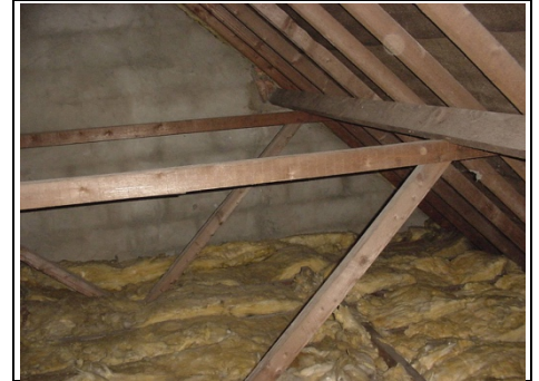
Chimney to right/middle viewed within roof space
