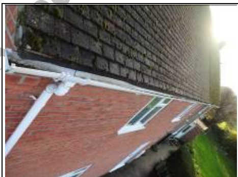
Gutter ~ Aerial View - 360 Photo ~
