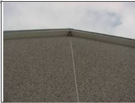
Jointing to a non-traditional house
