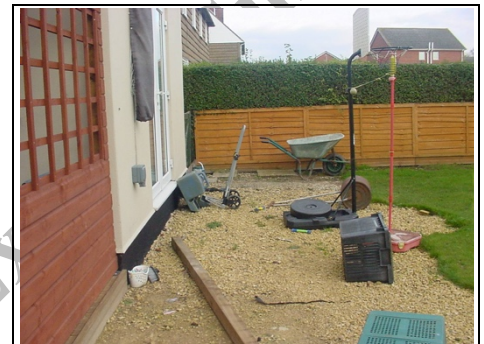
Unmade ground behind outbuilding area
