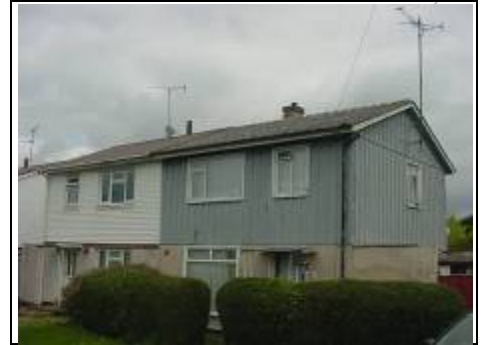
Asbestos roof on BISF house
