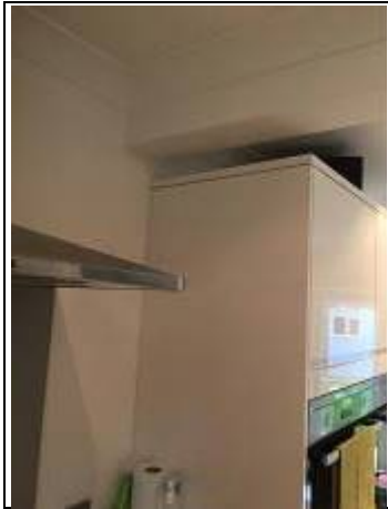
Beam in kitchen
