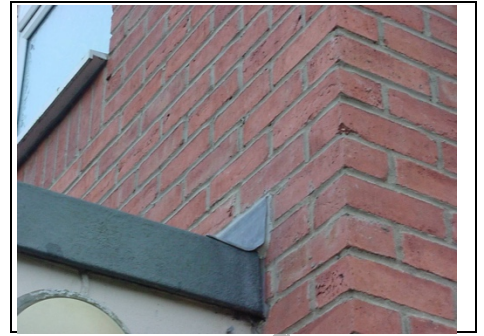
Flat roof meets main building
