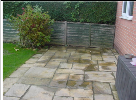
Rear paved area
