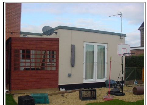
Rear left outbuilding
