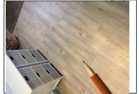
Engineered wood flooring in some areas
