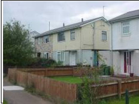
British Iron and Steel Federation House (BISF)
