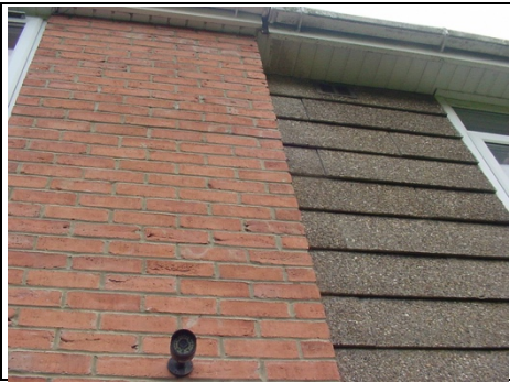
Area where brickwork meets Airey pre-cast concrete panels
