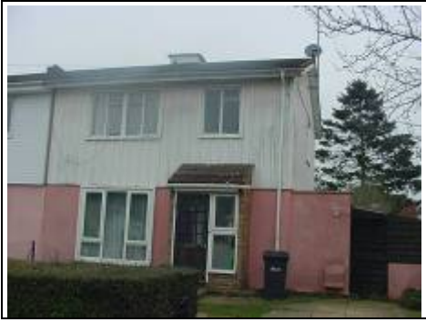
Painted cladding to non-traditional property
