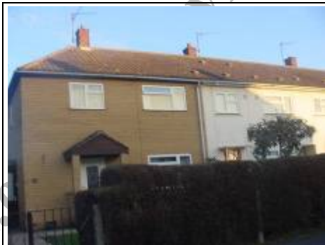
Brick clad modified non traditional house
