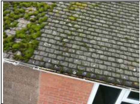
Close up of roof ~ Aerial View - 360 Photo ~
