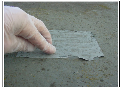
Close up of patch repair
