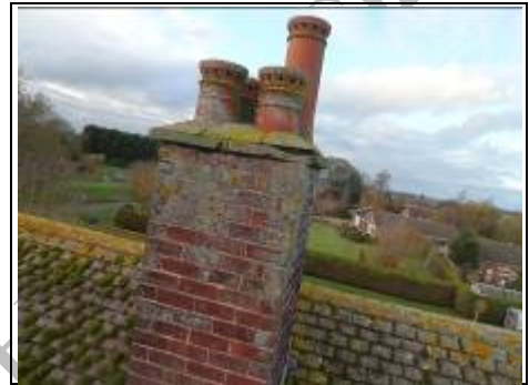
Chimney ~ Aerial View - 360 Photo ~
