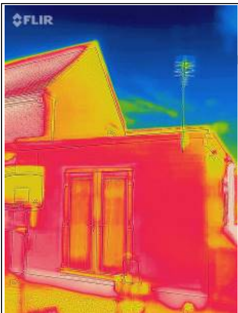
Rear of outbuilding
