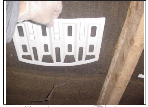
Pulling the vent completely out
