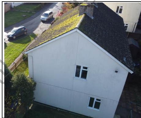
Chimney and right gable end ~ Aerial View - 360 Photo ~
