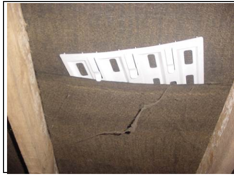
Pulling the vent partially out
