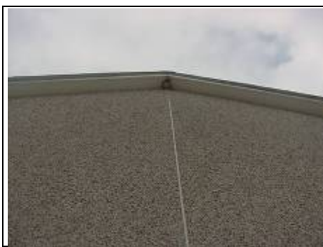
Jointing to a non-traditional house
