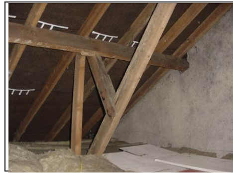
Gable end wall concrete structure
