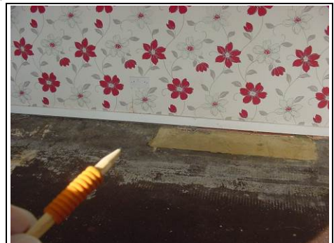
Lounge chimney removed
