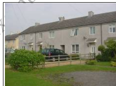
General view of a development of non-traditional houses
