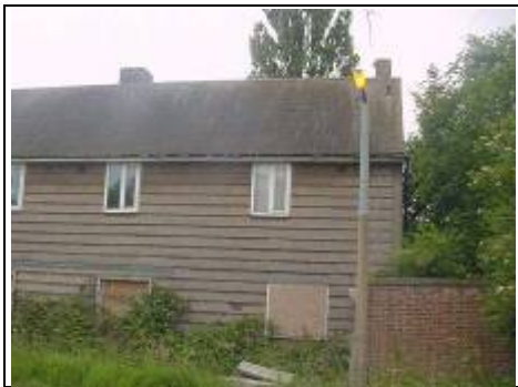
Airey houses were made up of concrete planks and are now generally being knocked down and rebuilt as they are not habitable
