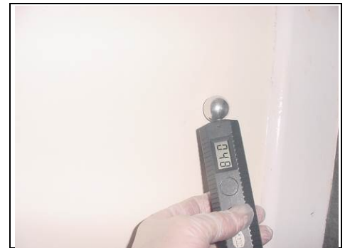
Testing for rising damp
