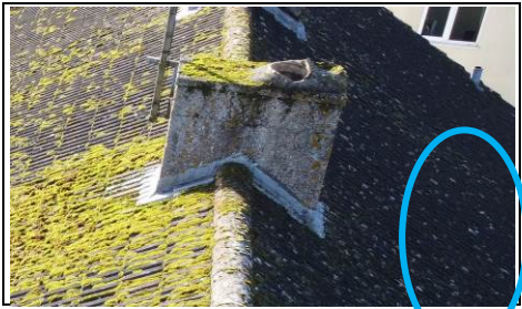
Close up of chimney Aerial view – 360 photo
