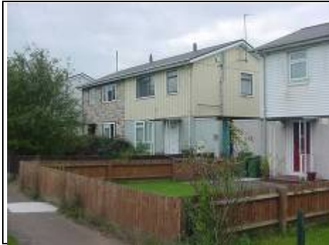
British Iron and Steel Federation House (BISF)
