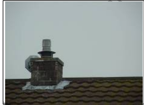
New chimney on a non-traditional house
