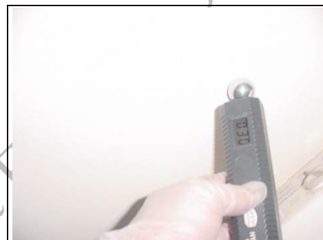
Testing for lateral dampness
