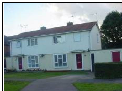
British Steel frame house (BISF)
