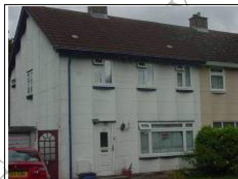
Non traditional house mainly asbestos
