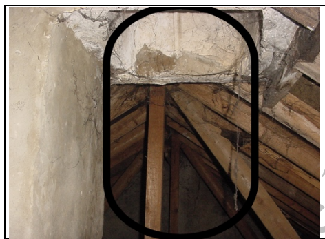
Front of chimney removed
