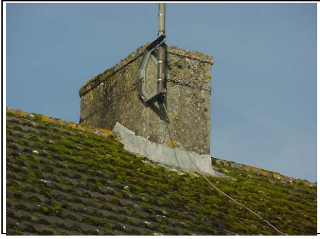
Lead flashing and aerial attached to chimney
