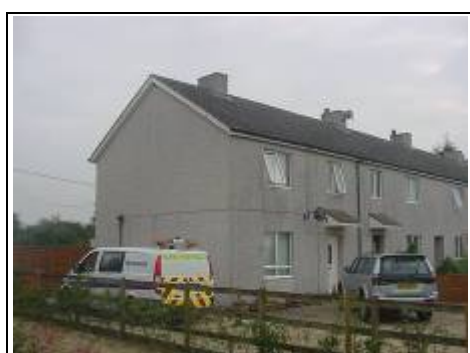
Large panel concrete non-traditional house
