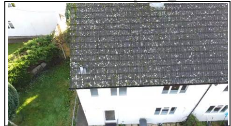
Concrete tile roof ~ Aerial View - 360 Photo ~
