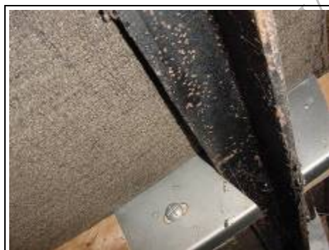
Some fixings replacements/repairs to a non-traditional house
