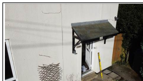
Porch roof Aerial view- 360 photo
