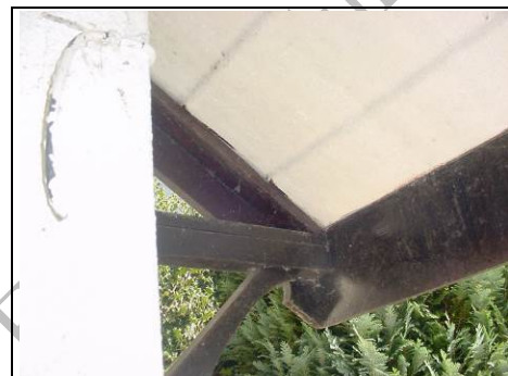
Underside of GRP roof
