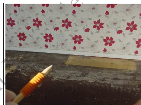
Chimney removed in lounge
