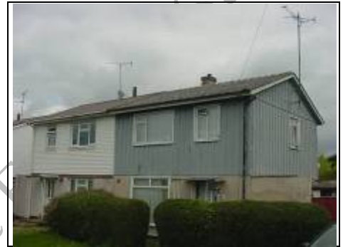
Asbestos roof on BISF house
