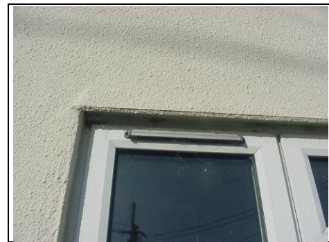
Drip detail over window
