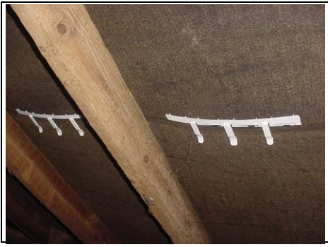
Vents in roof
