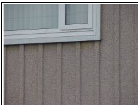
Close up of cladding on non-traditional house
