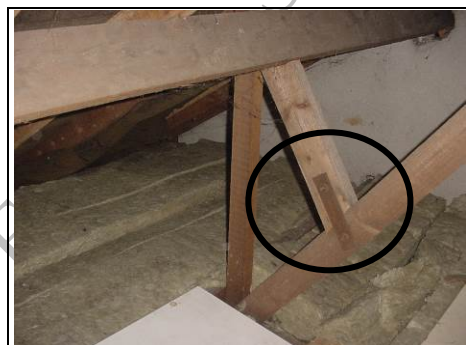
The roof truss has metal fixings
