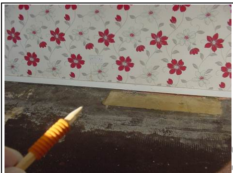
Lounge – chimney removed
