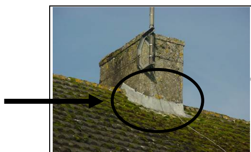
Flashing around chimney
