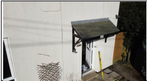
Front entrance GRP roof ~ Aerial View - 360 Photo ~
