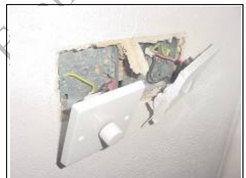
Removing electric points to view construction
