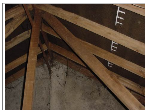
General view of roof with ridge board
