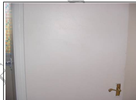
Plain panel door on first floor
