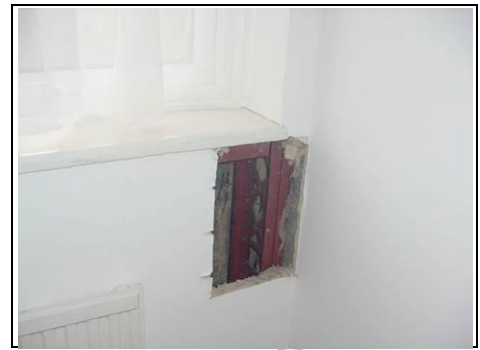
Example of opening up of a property (Not your property)
