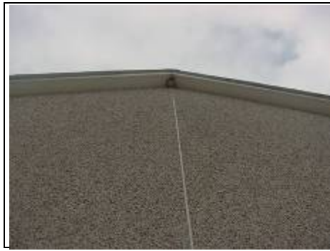
Jointing to a non-traditional house
