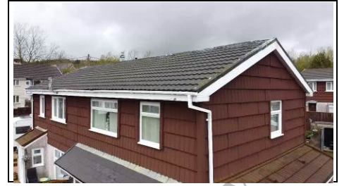
Pressed metal roof Aerial view – 360 photo
