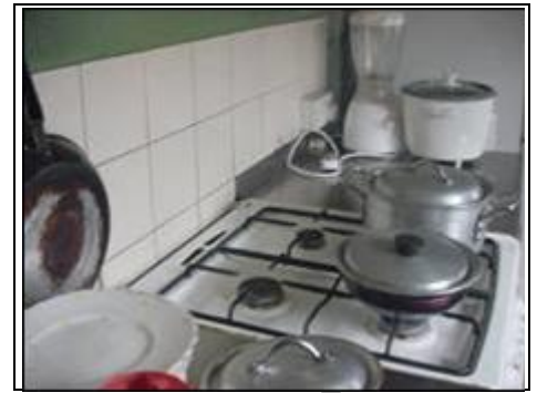
Cooking produces steam and requires ventilation
