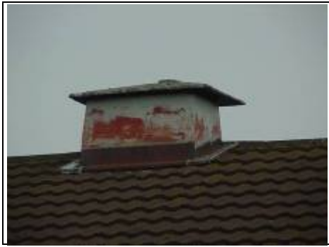
Asbestos original chimney non traditional house
