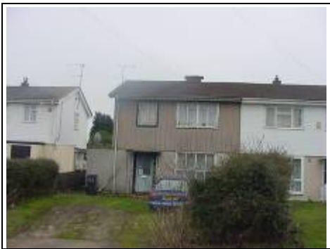
Original condition of non-traditional house with roof replacement
