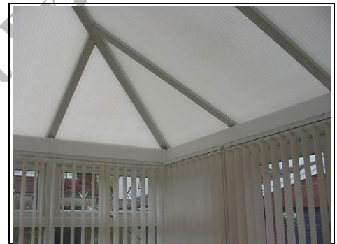
Looking up at the polycarbonate roof
