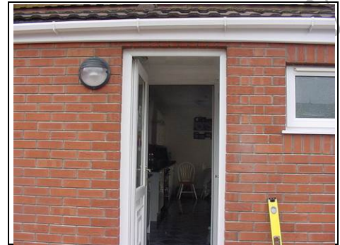
Brickwork to ground floor level
