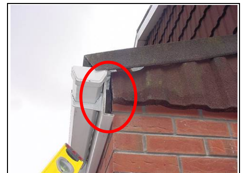
Plastic fascias and soffits over-cladding timber on the single storey roof
