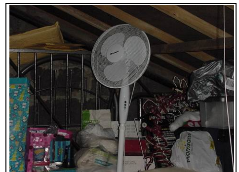
Stored items within the normal roof area
