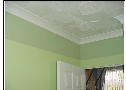
Textured paint in fan pattern
