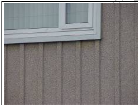
Close up of cladding on non-traditional house
