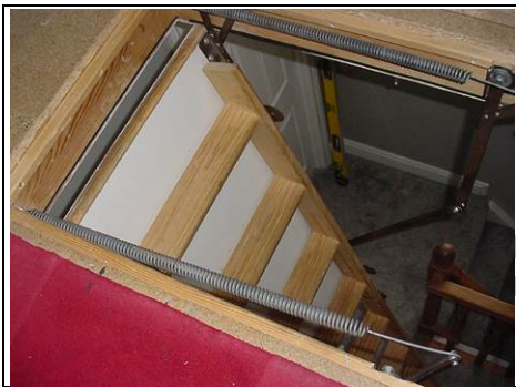
Loft hatch in lined and boarded area
