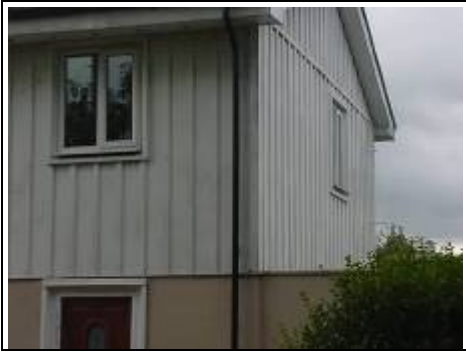
Originally the property would have had profile metal cladding
