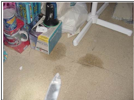
Damp stains in roof space, which we believe have been there a while
