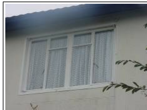
Close up of old metal windows in a non-traditional house
