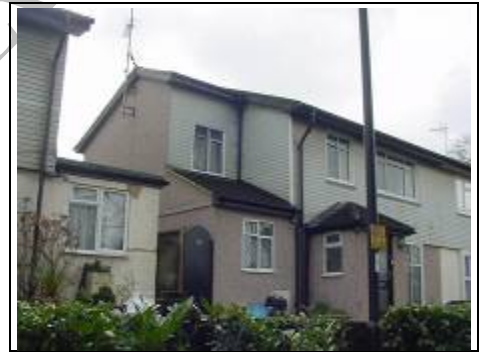
Pebbledash render in parts as well as plastic cladding and extensions but again the main part of the building is still a metal frame
