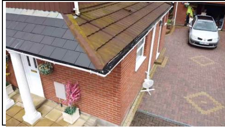
Corner where front and right single storey roofs meet Aerial view – 360 photo
