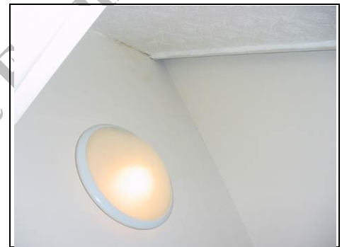
Textured paint under the stairs
