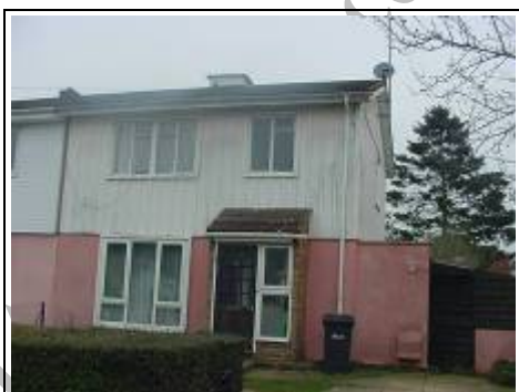
Painted cladding to non-traditional property
