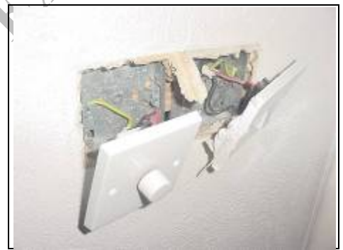
Removing electric points to view construction
