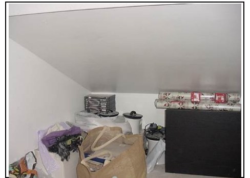
Loft lined/boarded out for storage
