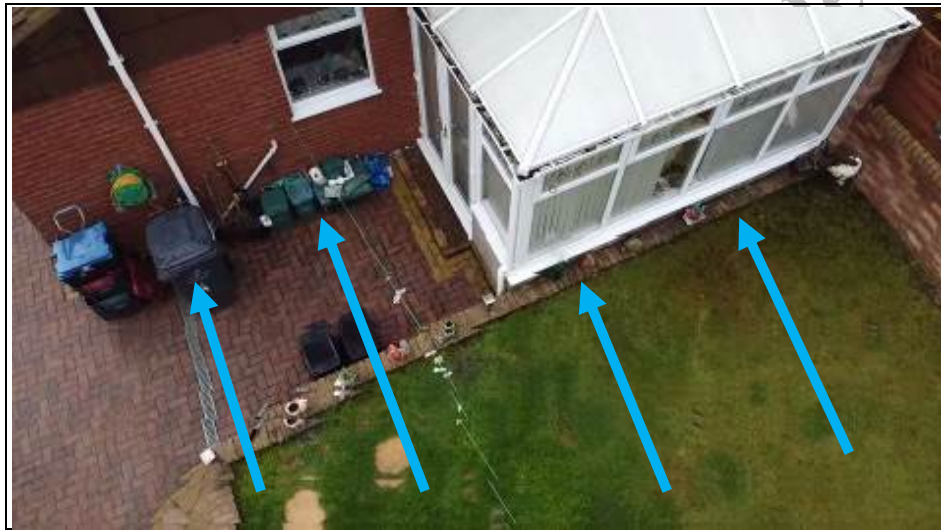
Sloping site running towards rear of property Aerial view – 360 photo
