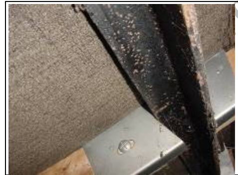
Some fixings replacements/repairs to a non-traditional house
