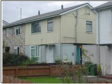
BISF property with metal profile sheet roof (has asbestos roof been removed or has it been overlaid?) and metal profile sheet at first floor level and render at ground floor level and older style double glazed windows. .
