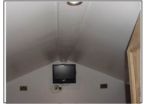
Right side of roof lined
