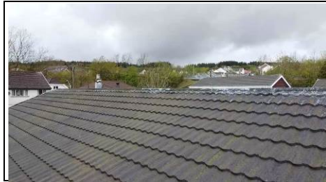
Pressed metal roof Aerial view – 360 photo
