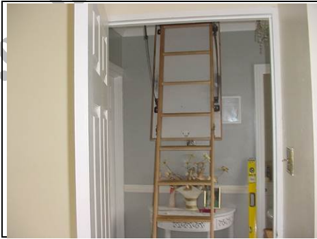
Loft hatch on landing
