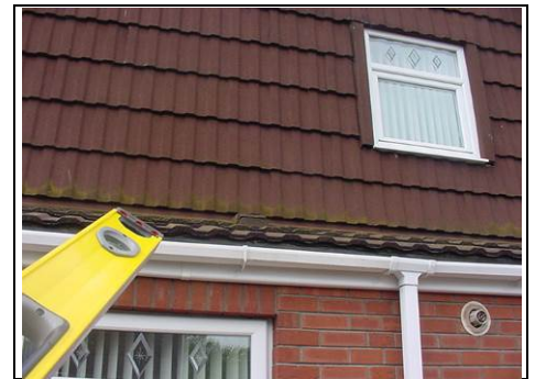
Vertical pressed metal wall tiles
