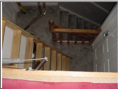
Landing and stairs looking down from loft
