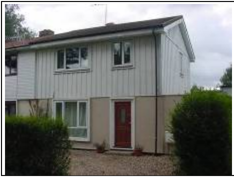
Metal frame house with profile metal sheeting at top and render at bottom. Roof has been changed.
