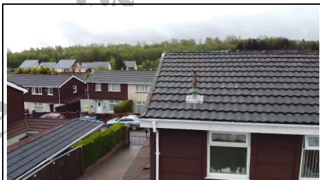
Top of internal soil and vent pipe to rear of property Aerial view - 360 photo
