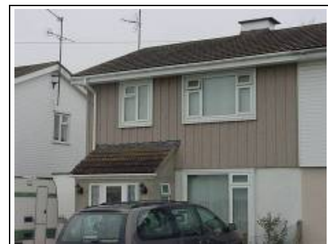
Non-traditional metal frame house
