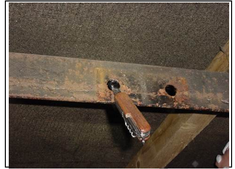
Area of roof space where we believe the chimney once was
