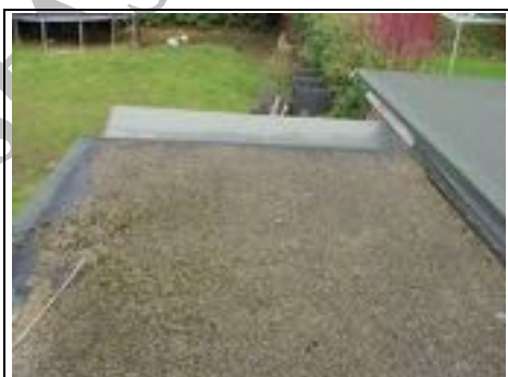
Garage roof ~ Aerial View - 360 Photo ~
