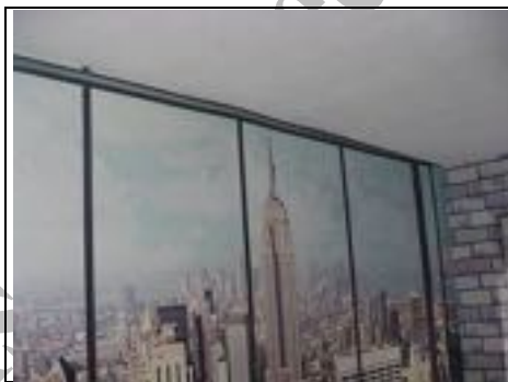
Has there been a lift in the ceiling?
