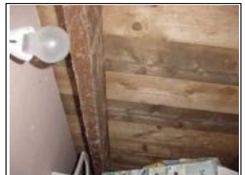
Close boarding to roof
