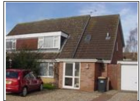
Example of two storey extension nearby
