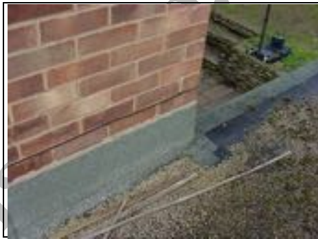
Felt flashing
