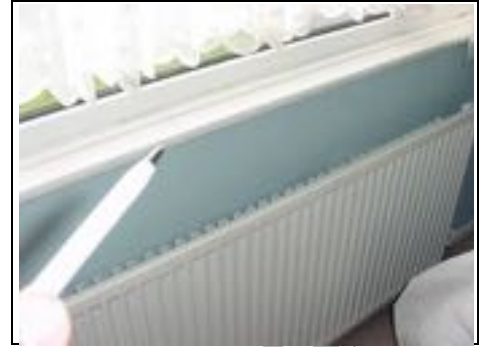
Single panel radiator
