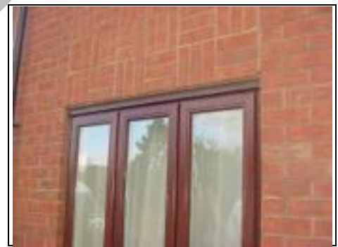
Era when timber (renewable source) windows returned with double glazing
