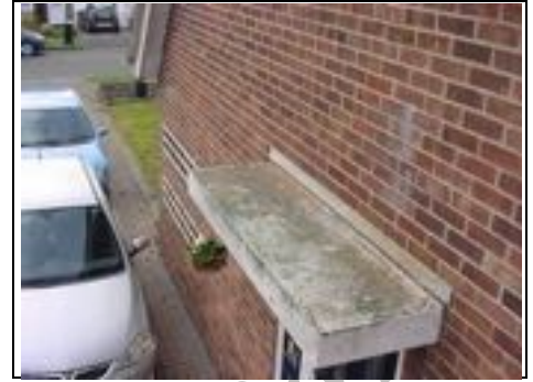
Front entrance roof
