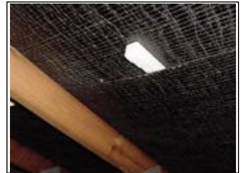
Spacers to help air ventilation
