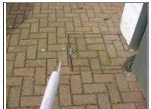
Manhole in front of garage
