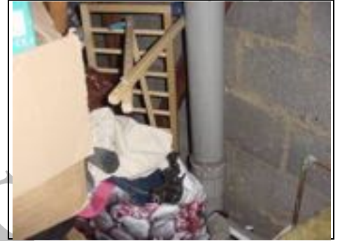
Stored items within roof
