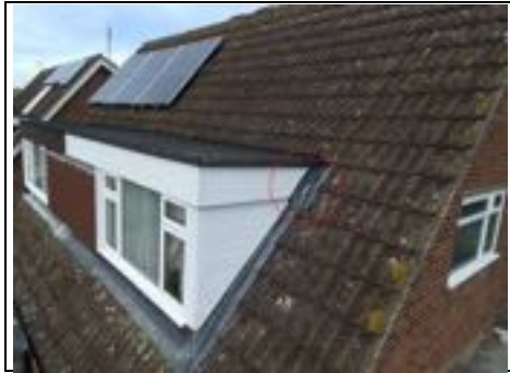
Repair to flashing ~ Aerial View - 360 Photo ~
