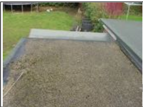
Garage flat roof
