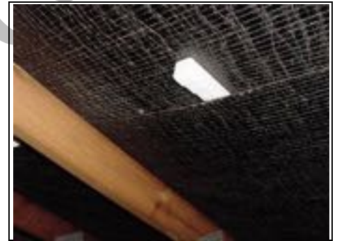
Spacers to help air ventilation
