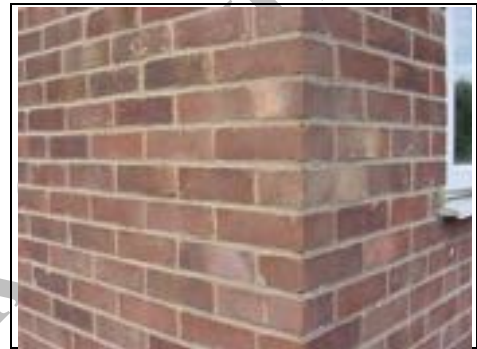
Stretcher bond brickwork
