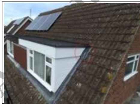
Repair to flashing ~ Aerial View - 360 Photo ~
