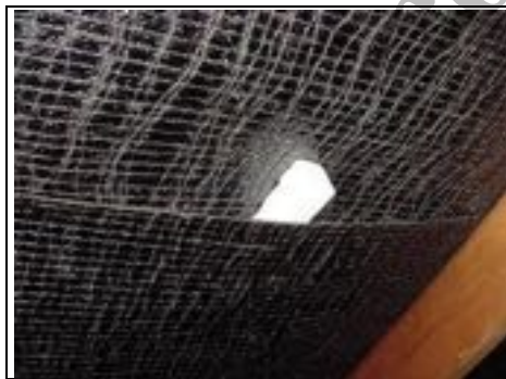
Spacer to protective underlayer
