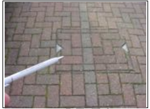
Manhole to middle of driveway
