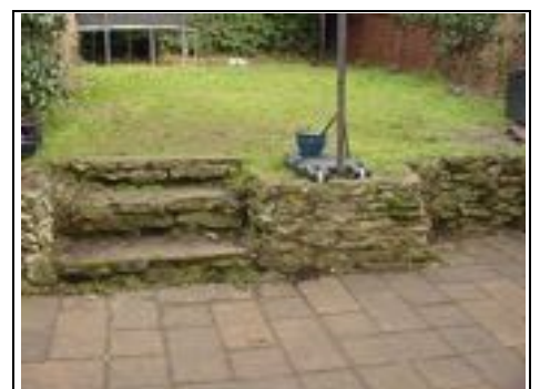
Step in garden due to sloping site
