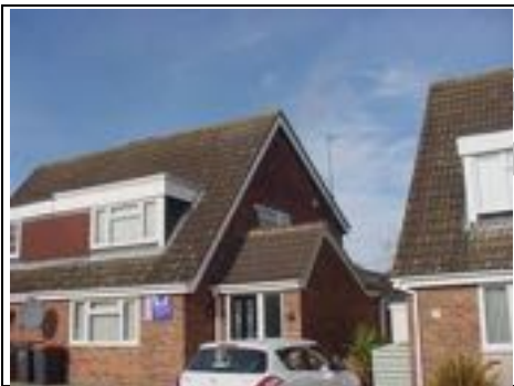
Example of single storey extension nearby
