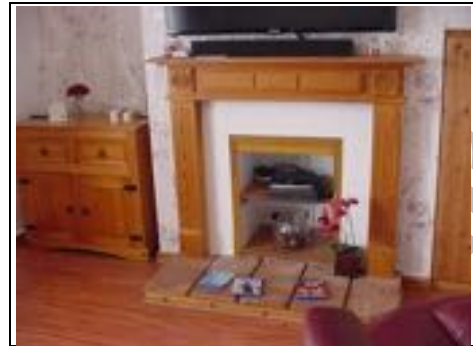
Front fireplace with asbestos flue
