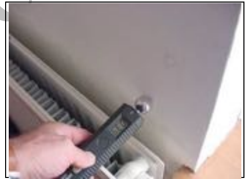
Testing for lateral dampness
