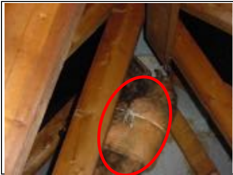
Close up of asbestos flue
