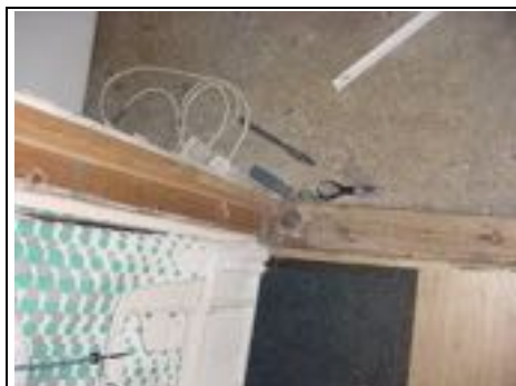
Front concrete floor and rear timber floor
