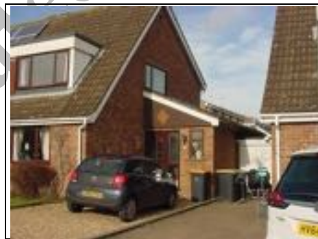
Example of single storey extension nearby
