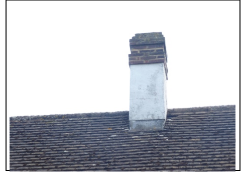
Middle chimney front view ~ Aerial View - 360 Photo ~
