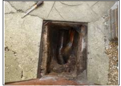
Rear left manhole
