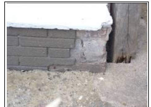
Brick tiles applied over top of brickwork
