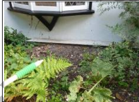
High ground level and render to base
