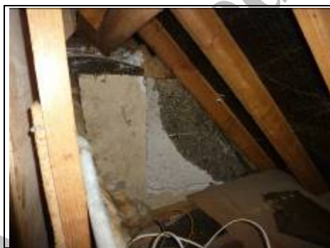
Right roof space
