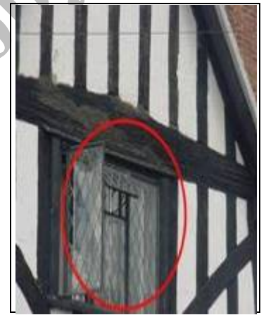
Old style diamond panel lead light in cast iron window opened to air room
