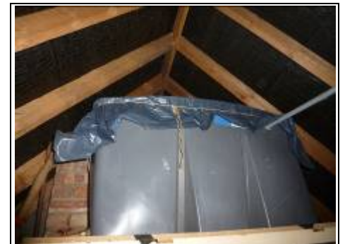
Water tank in newer left roof
