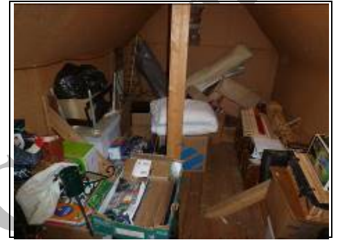
Stored items limited inspection
