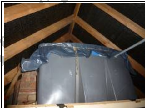
Water tank in newer left roof
