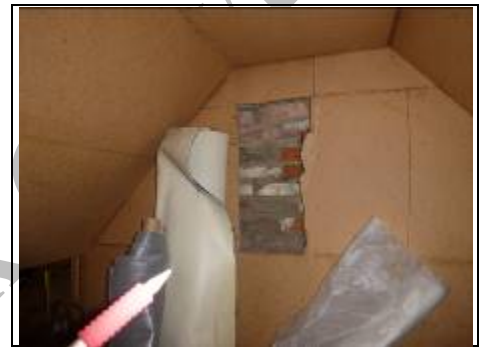
Left side of roof space and gable replaced in modern brick
