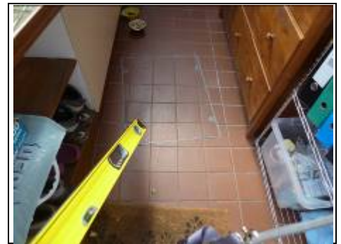
Manhole to rear entrance area
