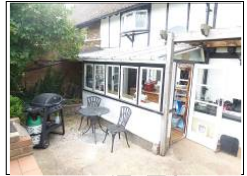
Rear entrance/boot room roof
