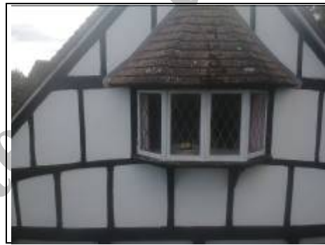
Oriel window on left gable ~ Aerial View - 360 Photo ~
