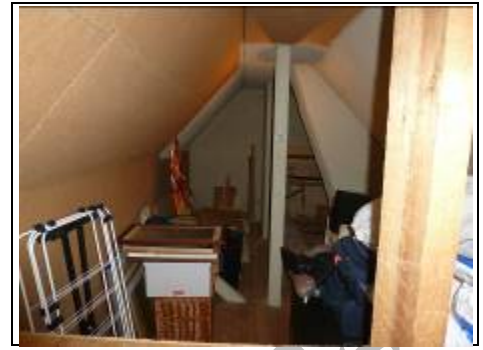
Right side of roof space
