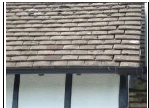
Opening up of tiles
