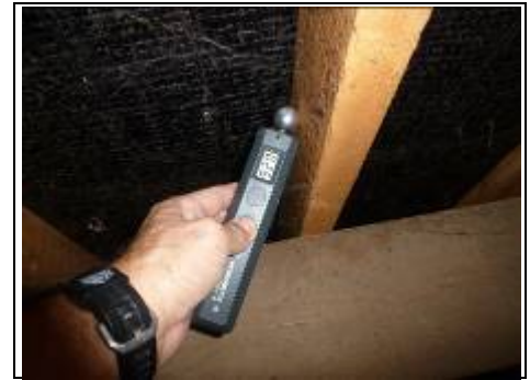
Damp testing common rafter
