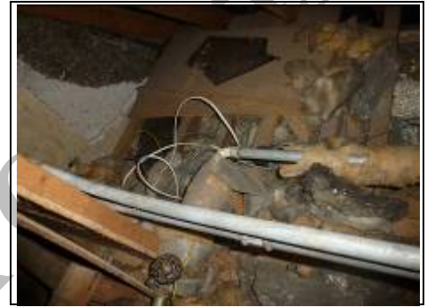
Pipes within roof space
