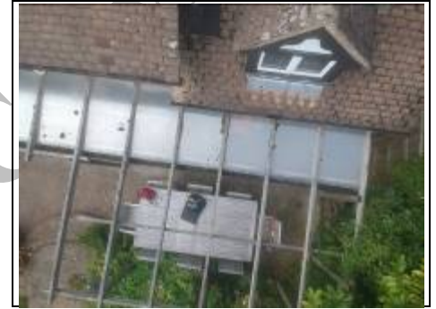
Rear canopy ~ Aerial View - 360 Photo ~
