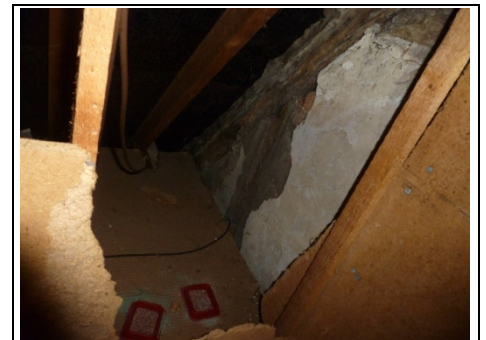
Old timbers in roof space
