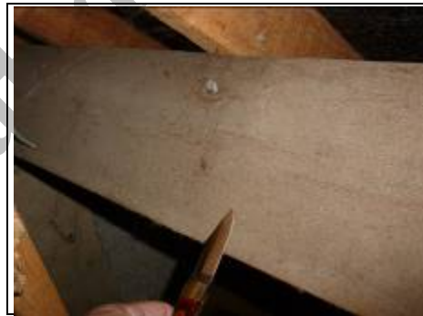
Knife test to purlin
