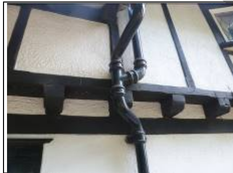
Cast iron gutters and downpipes
