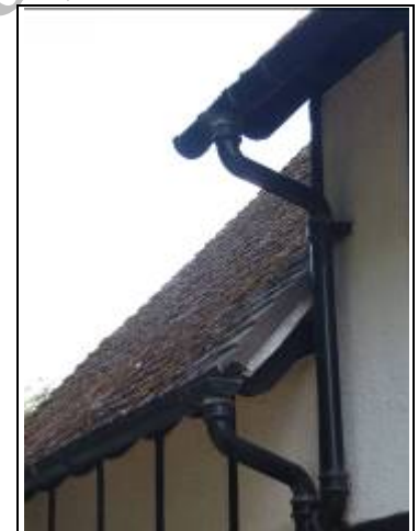
Cast iron and plastic gutters to front left
