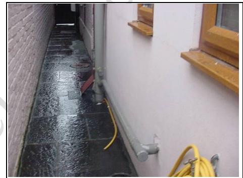
Right hand side is too high and needs the ground level lowering
