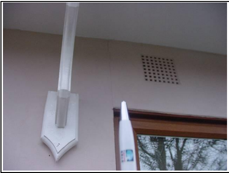
Crack in the render to the rear
