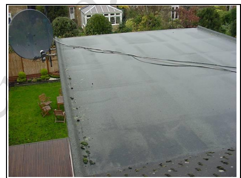
Flat roof to rear of property
