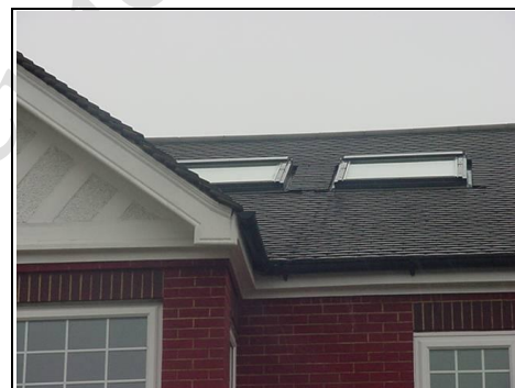
Fascias and soffits
