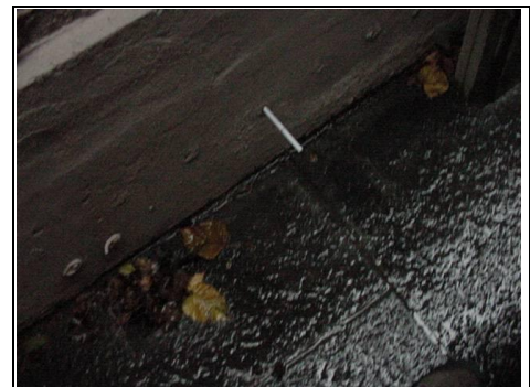
Damp proofing on right hand side
