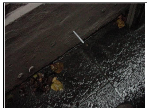
Damp proofing on right hand side
