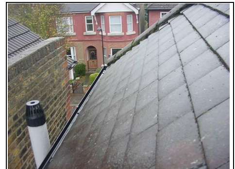
Close up of roof tiles
