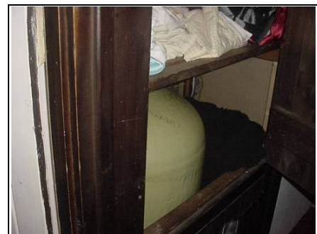
Hot water cylinder which is factory lagged
