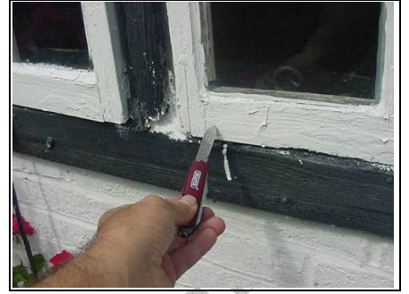
Knife testing the window
