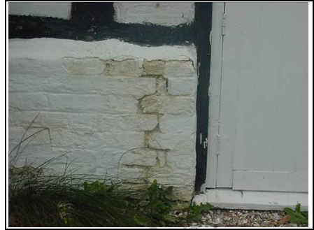
Brick plinth underneath the timber frame
