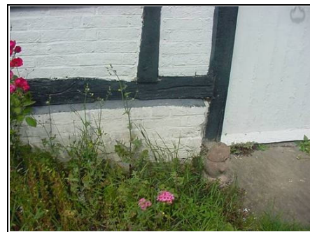
External timber frame with brick infill panel
