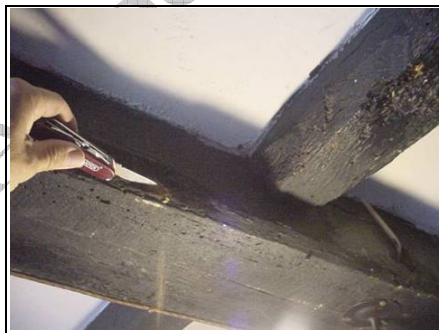
Internal spine beam with newish frass
