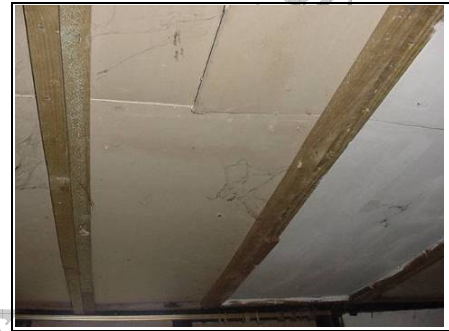
Infill to the ceiling
