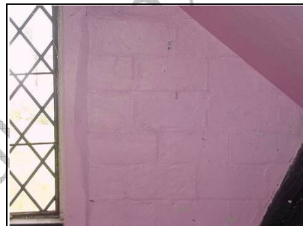
Within the corner of the rear right hand bedroom we can see brick on edge sometimes known as rat trap bond
