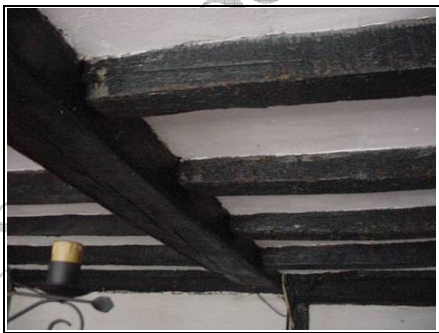
This shows the spine beams in the lounge
