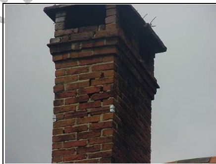
Close up of chimney one
