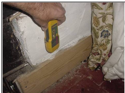
Checking for rising damp
