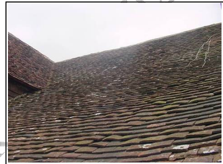
Mixture of hand made tiles and machine cut tiles
