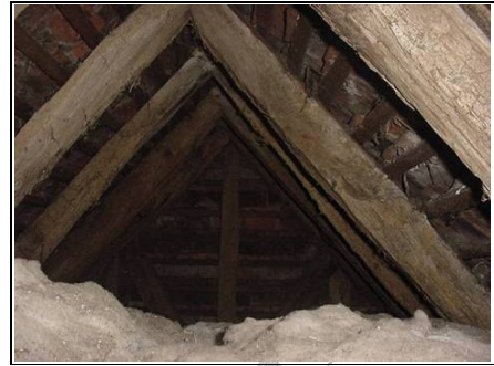
General view of roof
