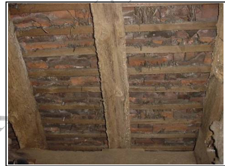
No protective underlayer (no sarking felt)
