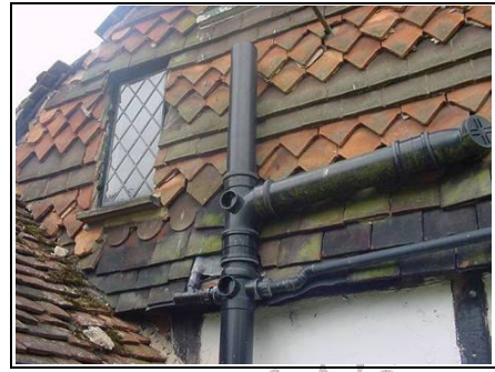
Plastic soil and vent pipe to the rear
