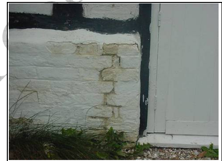
Close up of base of wall
