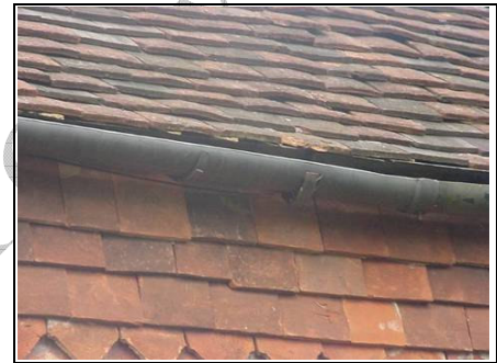
Plastic guttering
