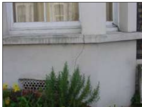
Cracking to next door neighbour's bay window (Right hand side neighbour), all directions as you face the property Cracking to the end gable of the end property
