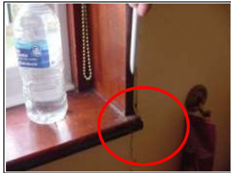
Crack to left hand side of window
