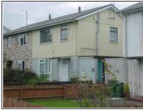
BISF property with metal profile sheet roof (has asbestos roof been removed or has it been overclad?) and metal profile sheet at first floor level and render at ground floor level and older style double glazed windows. .
