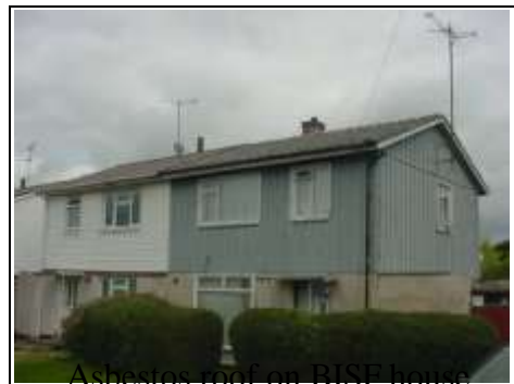
Asbestos roof on BISF house
