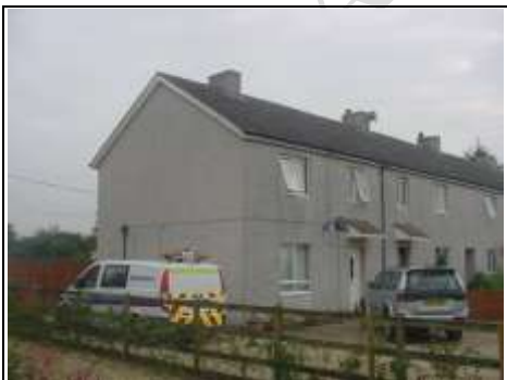
Large panel concrete non-traditional house
