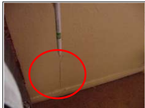
Crack on right hand side to base of wall near window
