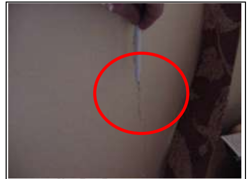
Close up of crack, approx half a metre to a metre in length
