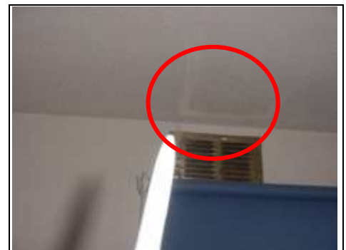
Crack around air vent
