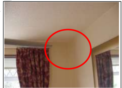
Wall to ceiling crack
