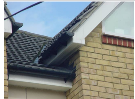
Awkward valley gutter detail
