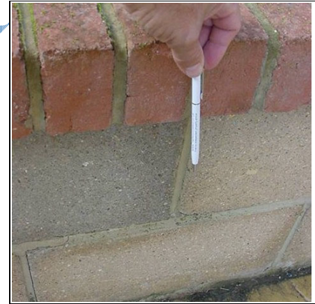
No weep holes to retaining wall
