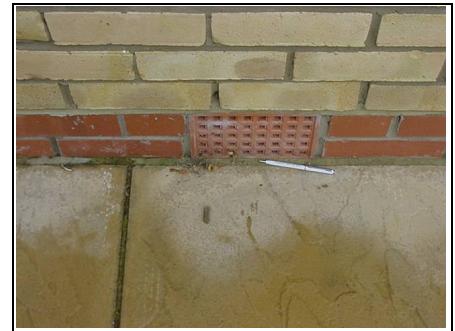
Airbricks acting as gutters
