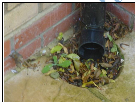
Blocked downpipes
