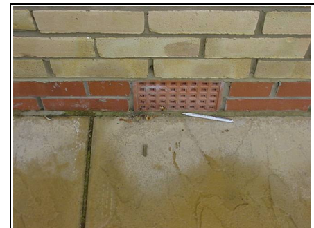
Air bricks acting as gutters
