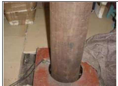
Central chimney which can rust
