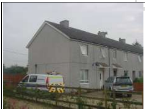
Large panel concrete non-traditional house
