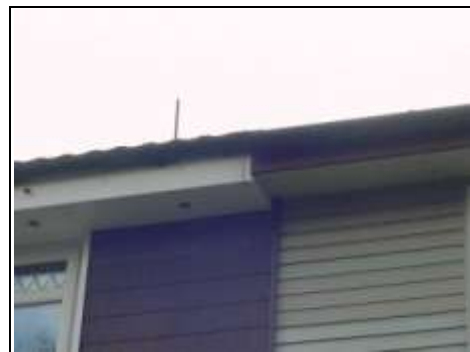
Example of plastic overcladding
