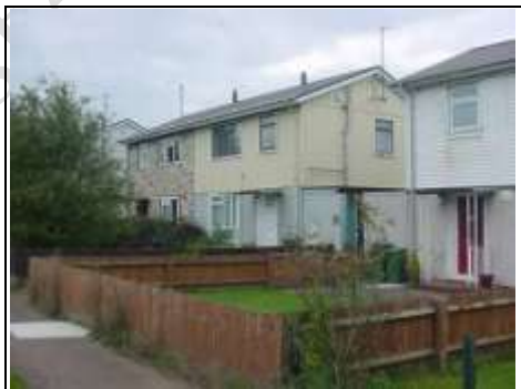
British Iron and Steel Federation House (BISF)
