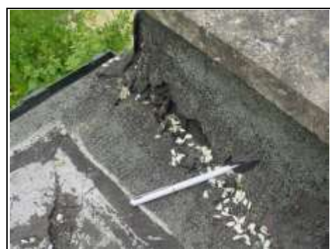
Felt has deteriorated to parapet wall
