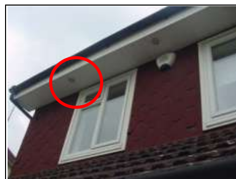
Lights in soffit board to front and rear of property are difficult to access to replace
