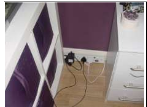
Overloading of electric points
