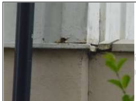
Rusting to profile metal cladding
