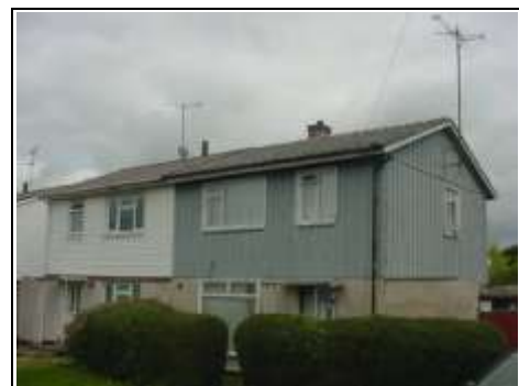
Asbestos roof on BISF house
