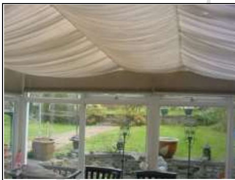
Linen ceiling in conservatory to limit heat loss and solar gain
