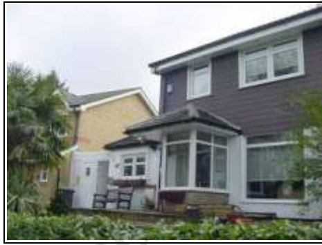
How vertical tiling and new windows can considerably change the look of a property but underneath it is still a metal framed building
