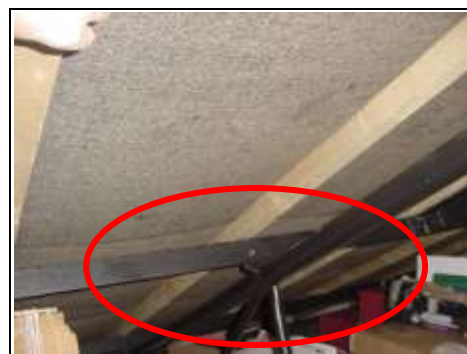
Metal frame, purlin and metal truss
