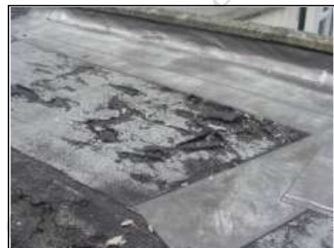
Deterioration to flat roof repaired with flashband
