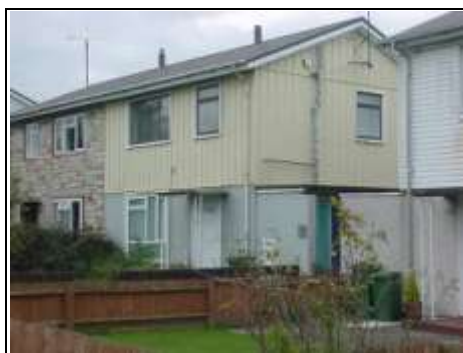
Marketing by: BISF property with metal profile sheet roof (has asbestos roof been removed or has it been overclad?) and the 1st floor sheet at first floor level and render at ground floor level and modern styled double glazed windows.
