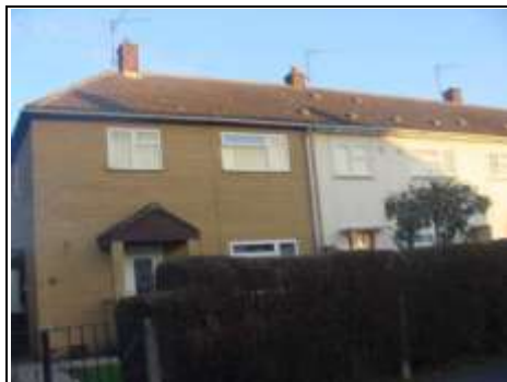
Brick clad modified non traditional house
