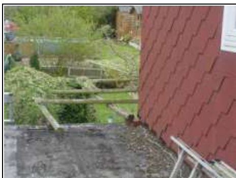
Wooden trellis to front is not secure and is balanced in place by a brick and is only held by luck and gravity as far as we can see
