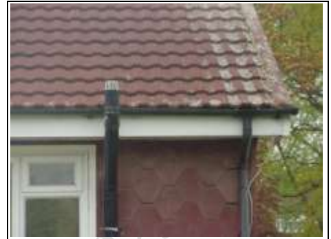
Soil and vent pipe
