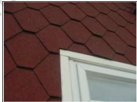
How vertical tiles sit around the windows
