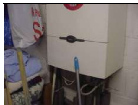
Wall mounted Baxi boiler
