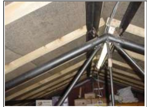
Top of metal truss and roof timbers
