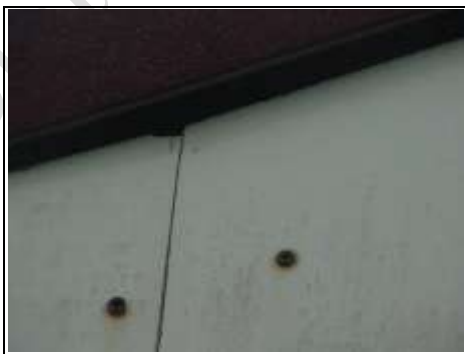
Rusting screws to fascia board
