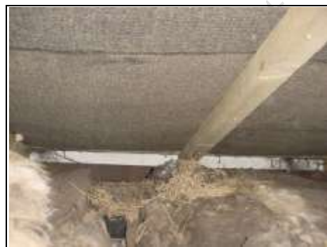
Insulation with building paper underneath and a birds nest
