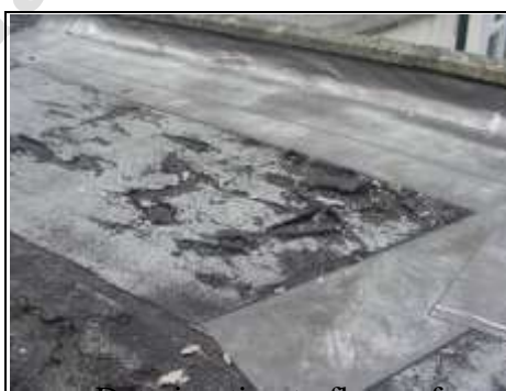
Deterioration to flat roof repaired with flashband
