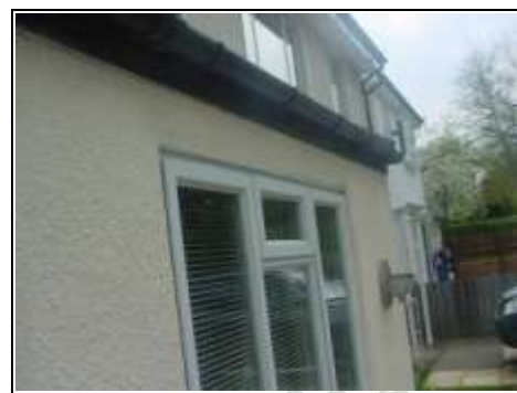
Plastic double glazed windows without trickle vents
