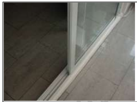
Inside and outside floor levels almost the same
