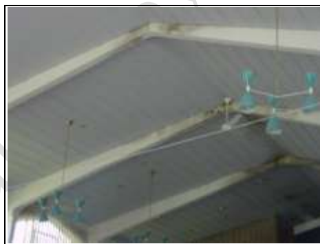
Cold Bridging in a commercial property with a concrete frame.
