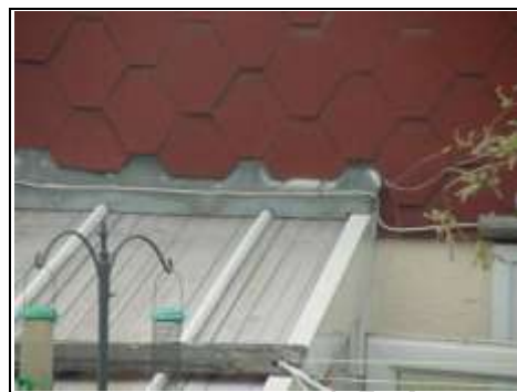
Conservatory roof links into vertical felt tiles
