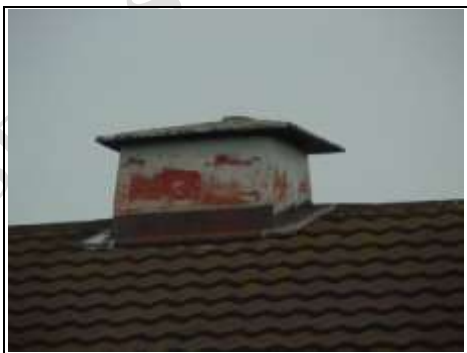
Asbestos original chimney non traditional house
