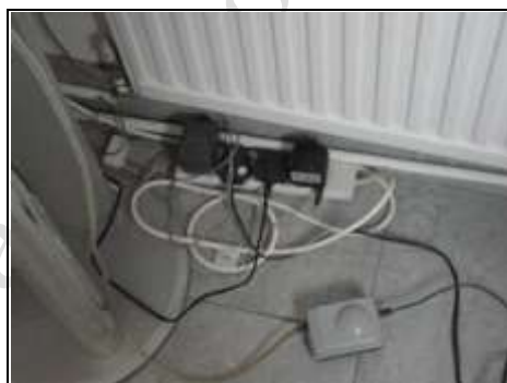
Cable extensions being used
