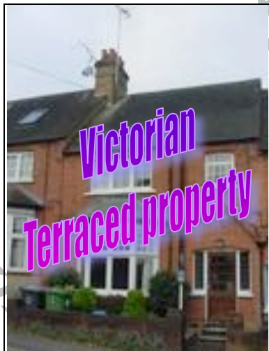
Front left chimney
