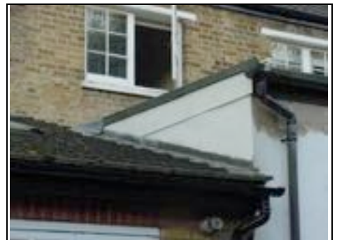
Flat roof meeting next door's low level pitched roof
