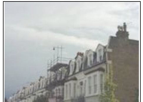
Loft conversion and dormer windows
