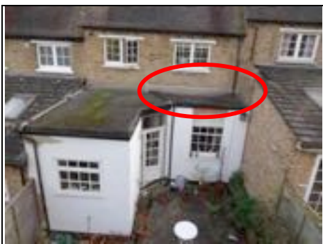
Rear right flat roof Aerial view – 360 photo
