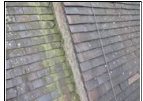
Step in roof And moss on tiles Aerial view – 360 photo
