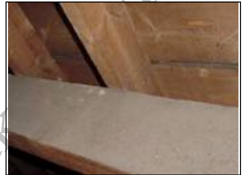
Purlin, common rafter and close boarding
