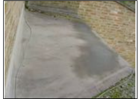
Rear right flat roof
