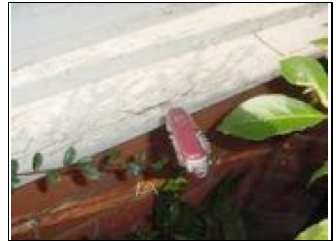
Knife test of timber windows
