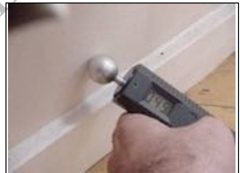
Testing for rising damp in front bay
