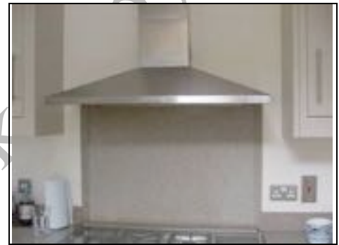
Filter over cooker – not an extract fan
