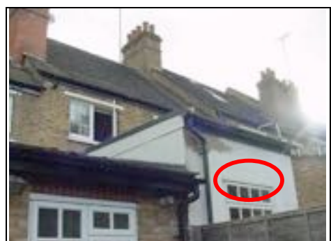
No drip detail above window
