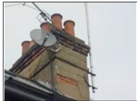
Render deteriorating
