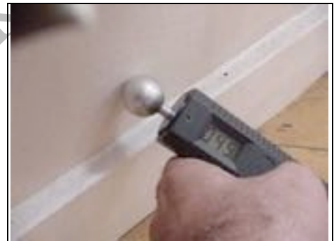
Checking for rising damp
