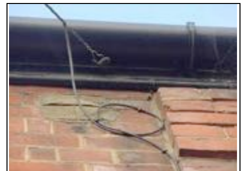
Blocked up air vent from bathroom
