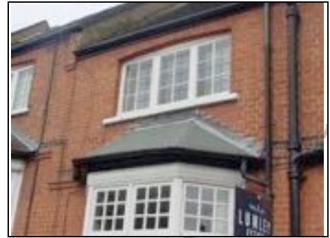
Front bay window roof
