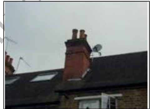
Rear right chimney
