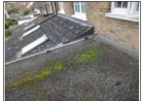
Rear left flat roof
