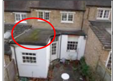
Rear left flat roof Aerial view – 360 photo
