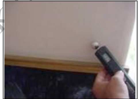
Testing for lateral dampness
