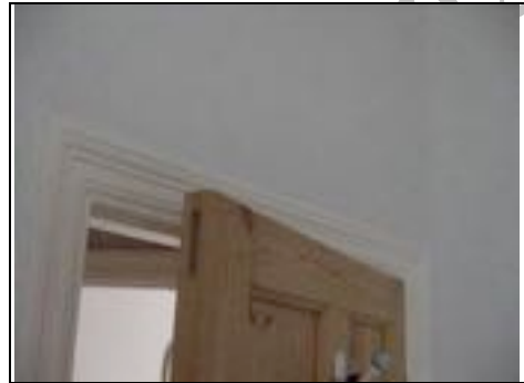
Checking doors for movement
