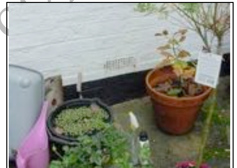
Air brick to rear
