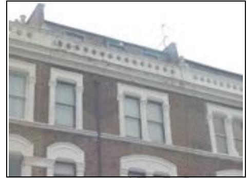
Classic Victorian Sliding sash windows where they have managed to put in one pane of glass
