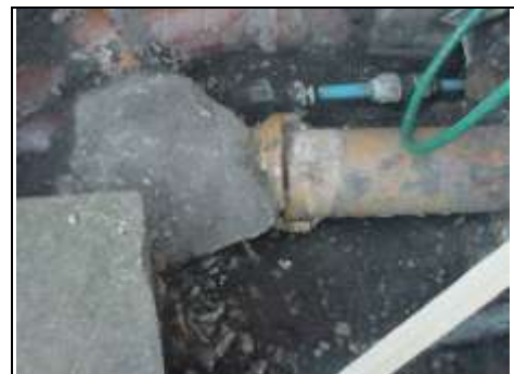
Redundant soil and vent pipe that needs to be checked
