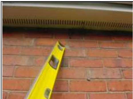
High level drill holes to left side where insulation has been added
