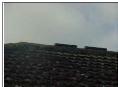
Vents have been added in the roof. These work in conjunction with the soffit vents so you may have to move the insulation back in the roof space
