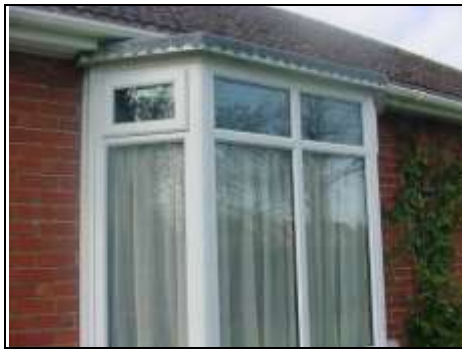
Front bay without trickle vents
