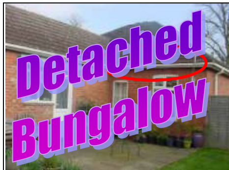
Interlocking concrete tiles to rear of roof, with lighter coloured tiles being replacement tiles that were broken
