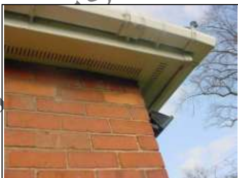
Fascias and soffits with vents. Are they being blocked by the insulation in the roof?
