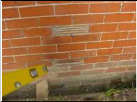
Vent under floor needs checking to see if it is blocked by insulation, particularly if there is a defective DPC. Check with a long screwdriver that it is working
