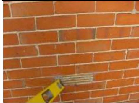
Blocked air brick which leads us to believe there is no longer a through flow of air at low level
