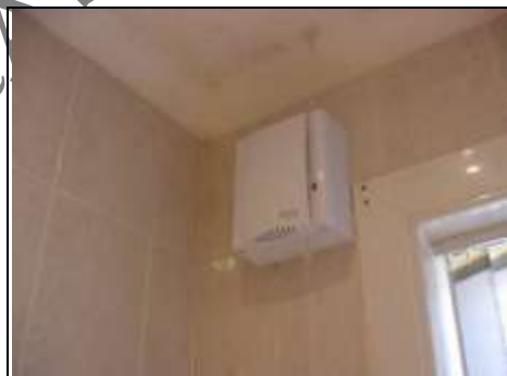
Humidity controlled extract
