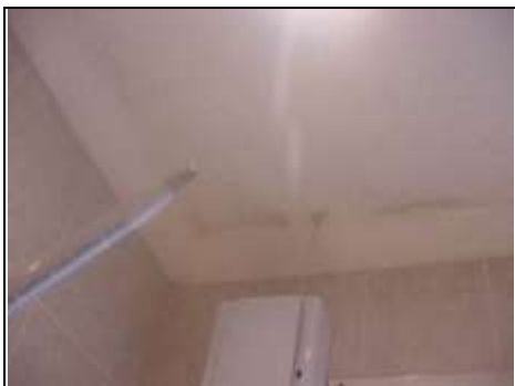
Black mould in bathroom
