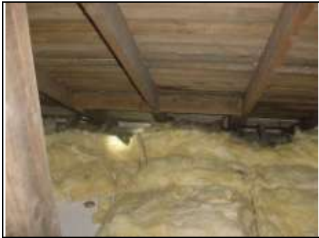
Insulation may be blocking air ventilations although can't be certain
