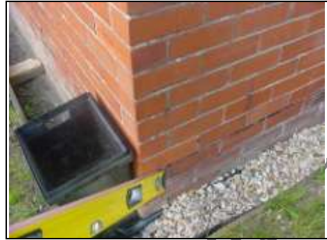
Basic French drain to front. It should really have a perforated drain on it to allow water to get away from the building, albeit you have more than two bricks between the DPC and the ground level
