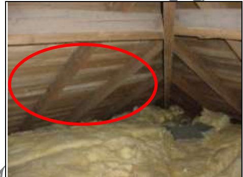
Efflorescence on timbers to rear left side
