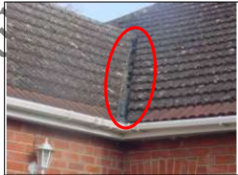
Valley gutter looks to have been tarred. Double check to make sure it is watertight
