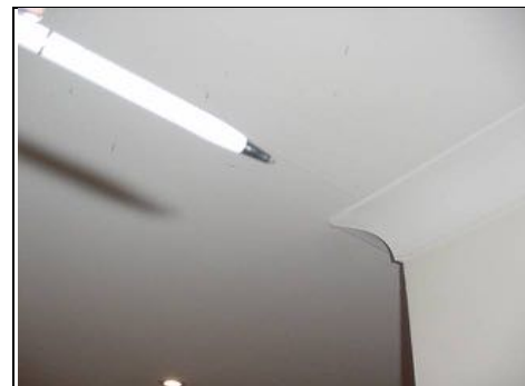
Ceiling hairline cracking
