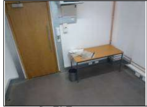
Room One showing exposed pipes
