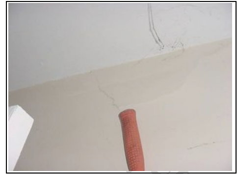
Internal cracking in toilets
