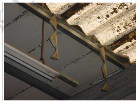
Ceiling tiles in place, note the water damage around the suspended ceiling units
