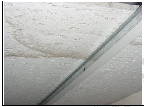
Staining to ceiling tiles
