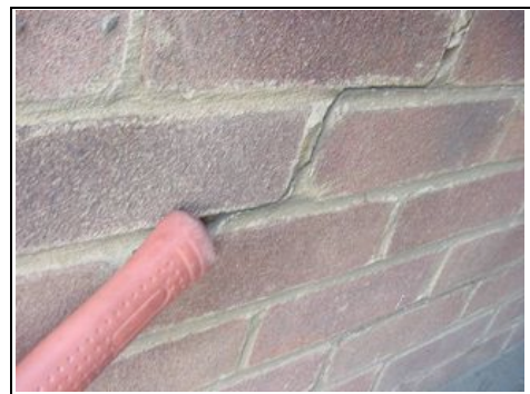
Cracking to brickwork
