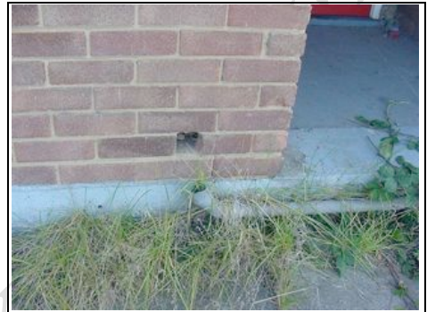
Drainpipe not connected
