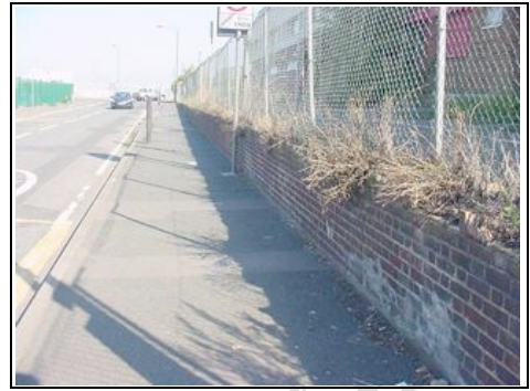
Retaining wall indicates that built up land has been used in this area
