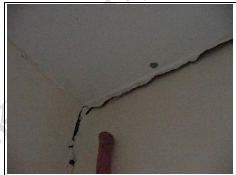
Cracking between wall and ceiling in hallway
