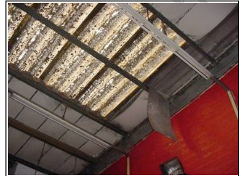
Asbestos roof taken from internally
