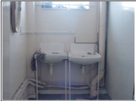
Ladies toilets internal soil and vent pipe
