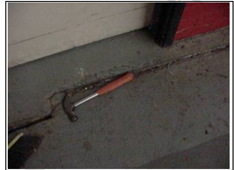
Floor subsidence to the front toilets
