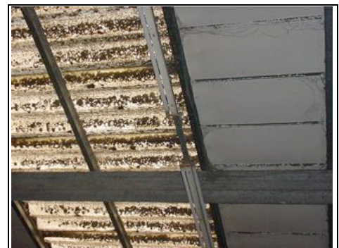
GRP roof light in need of cleaning
