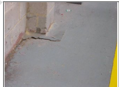
Post Office warehouse subsidence to the rear
