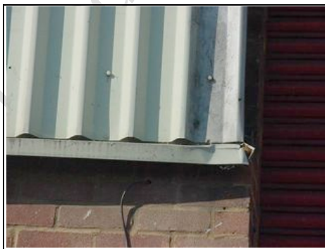
Impact damaged profile sheeting
