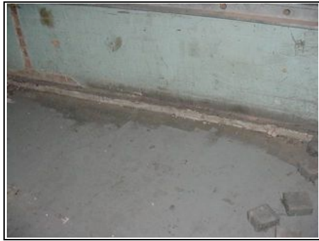
Floor subsidence to the rear of the warehouse
