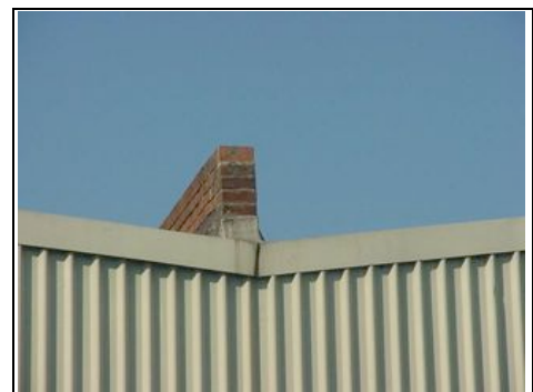
Parapet wall which is weathered and looks to have had a repair to the flashing and needs new flashing and coping stone
