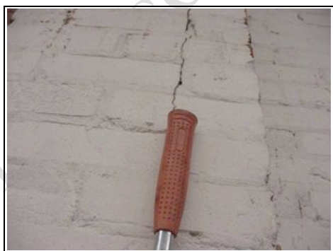
The hammer handle indicates where the cracked line is to the pier
