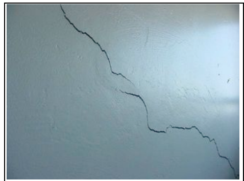
Cracks ground floor partition
