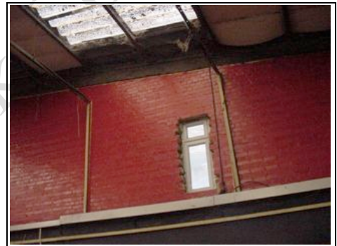
Block broken through to form window not been made good
