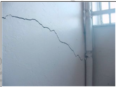
Cracks ground floor partition
