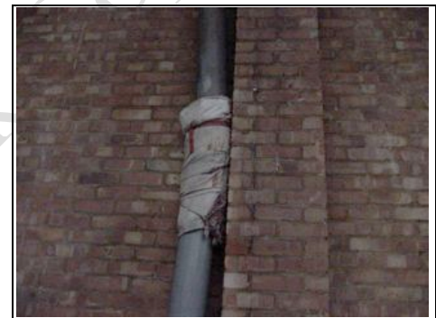
Cracking around columns in warehouse
