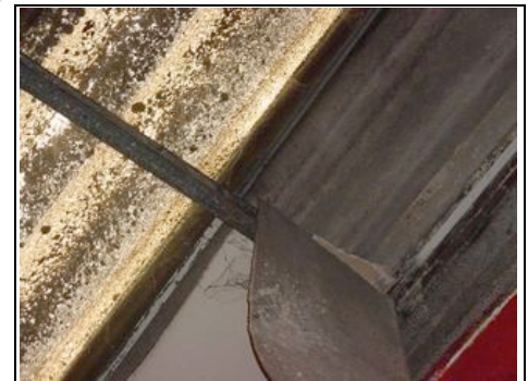
Close up of asbestos sheet on roof
