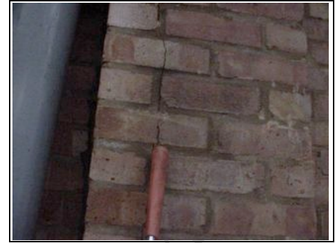
Cracking in warehouse
