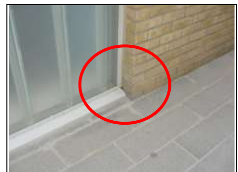
Opening in sill detail
