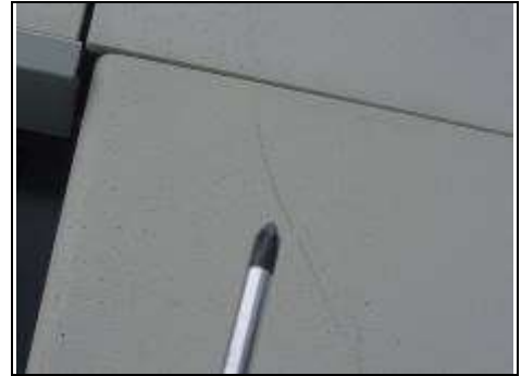
Mark to rain cladding
