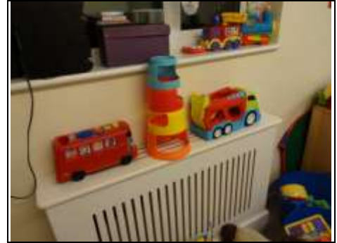
Example of covered radiator
