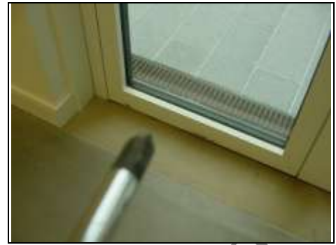
Running gulley protects left door
