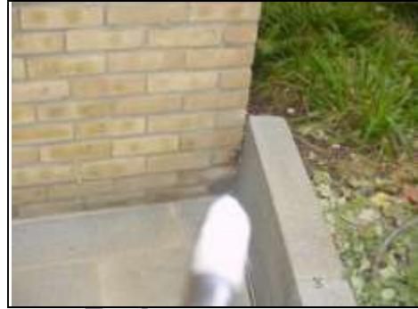
Close up of where high ground level starts
