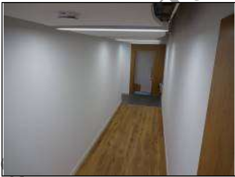
Link corridor Two to open plan room (Access to courtyard two)
