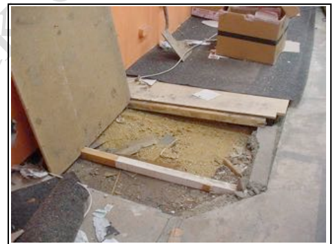
Wood flooring to side
