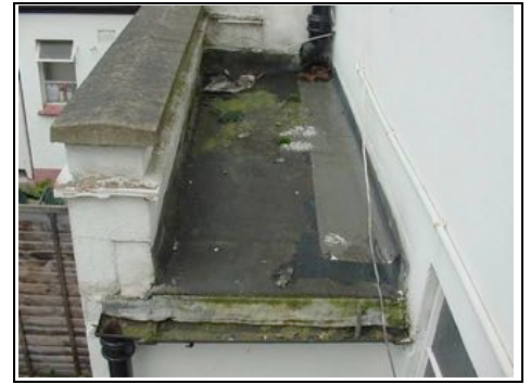
Roof over the entrance, patch repaired in Flashband
