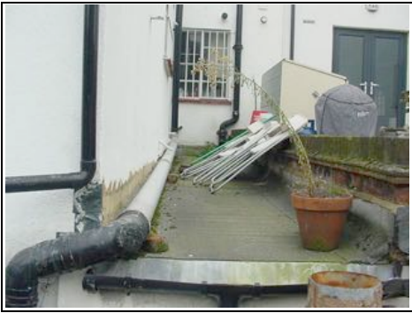
Flat roof over the shop
