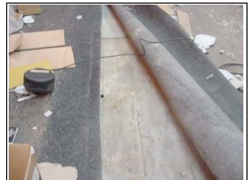
Concrete floor to centre
