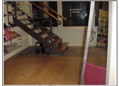
Customer's stairs to first floor
