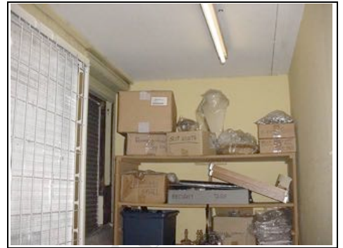
Ceiling in plant room
