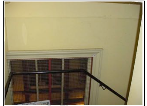
Window within staff staircase area
