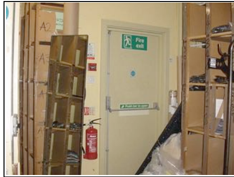
Fire exit to spiral staircase
