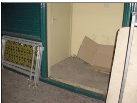
Lobby area giving access to basement via a ladder
