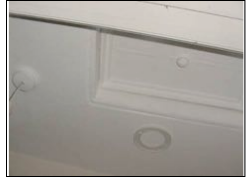
Loft hatch to roof space
