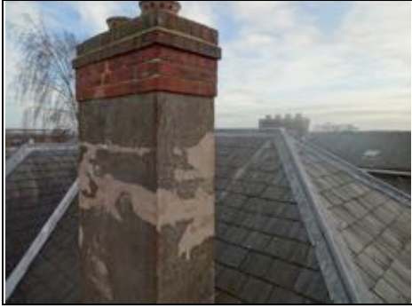
Rear right chimney Aerial view – 360 photo
