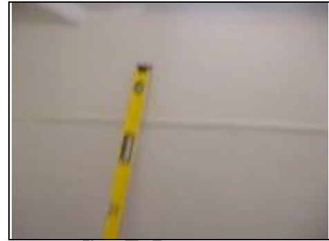
Hairline cracking
