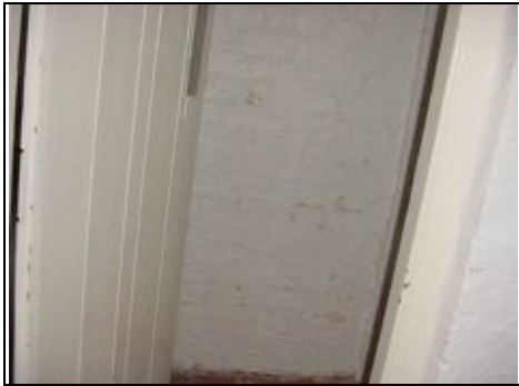
Painted brick walls
