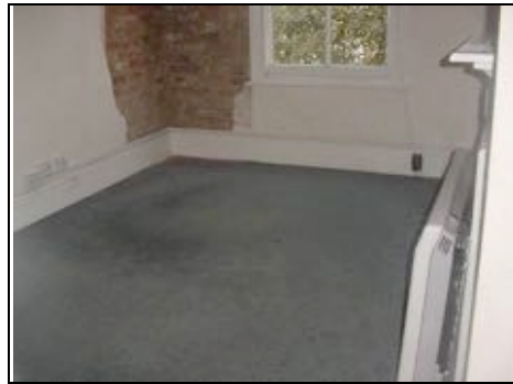
Front right office
