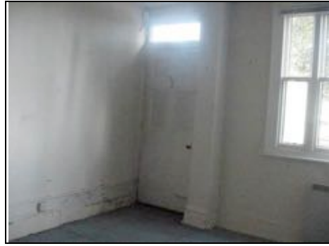
Front right office
