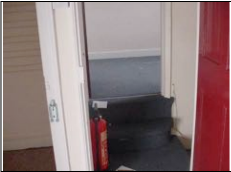
Steps up to front office
