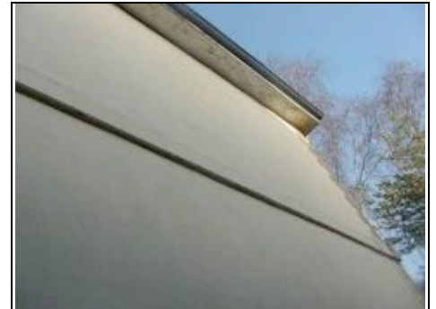
Modern plaster to left side
