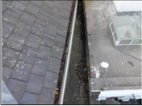
Close up box gutter Aerial view – 360 photo
