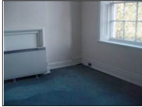
Front middle board room
