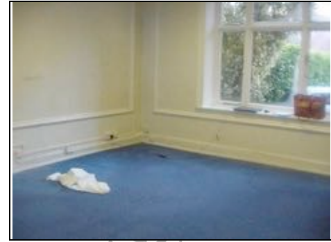
Rear left through office
