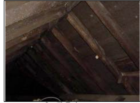
Mould to timbers
