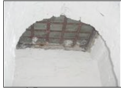
Glazed ceiling light to unknown area
