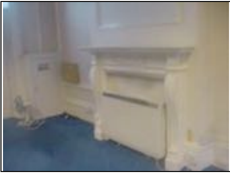
Electric fire in front of fireplace
