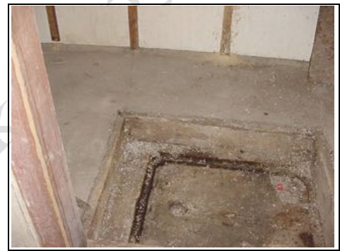
Drain within basement
