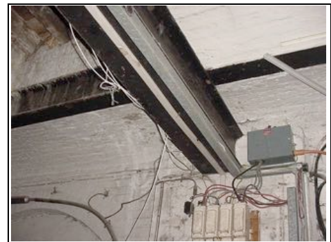
New steels added in basement 12
