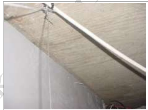
Concrete on the first floor
