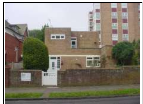
1960's concrete frame
