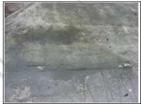
Close up view of entrance area roof
