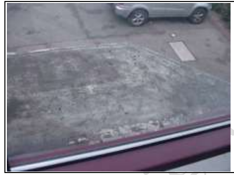
Entrance area roof, we recommend guttering is added
