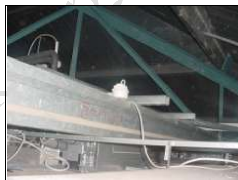
Steel frame forming roof structure
