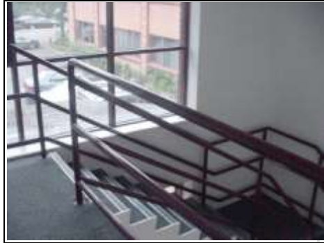
Landing and stairway area
