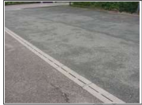
Central running gully to car park area
