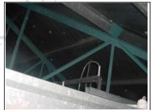
Void above roof – you will be heating Basildon!
