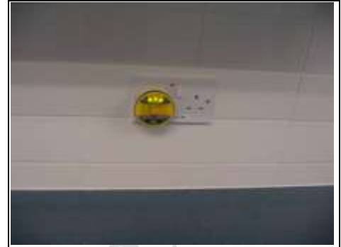
Earth Test ground floor kitchen
