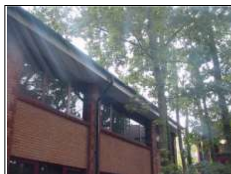
Restricted view on left hand side and rear main roof
