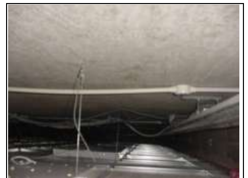
Ceiling ground floor
