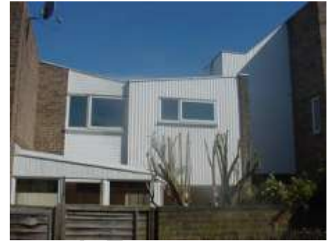
Typical 1970's house
