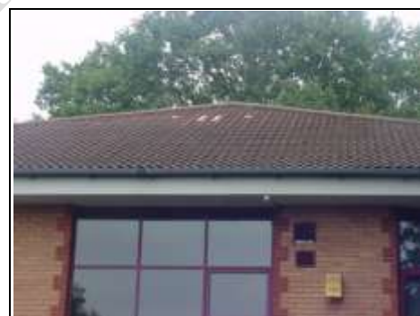
Main roof with mushroom vents
