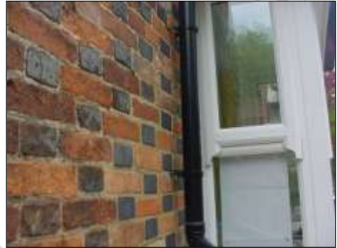
Replacement repaired brickwork at front of main building
