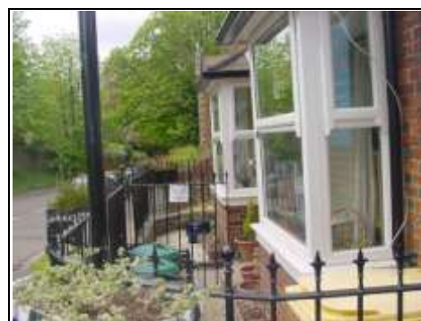
Plastic windows to front of main building
