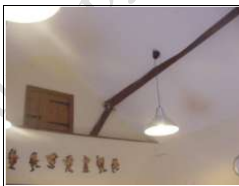
Lath and plaster ceiling
