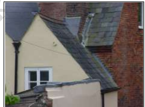
Lead tingles to rear of main roof
