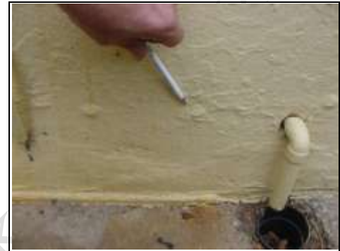
Old inserted damp proof course to right hand side main building
