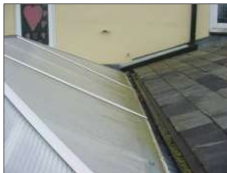
Valley gutter between conservatory and kitchen area
