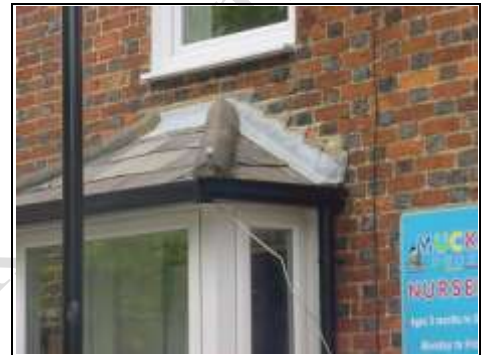
Front main building bay window roof
