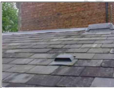
Rear slate roof in average condition
