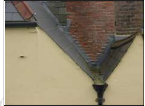
Valley gutter to rear of property at high level
