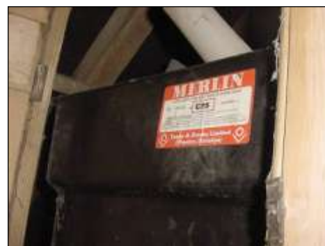
Disused water tank
