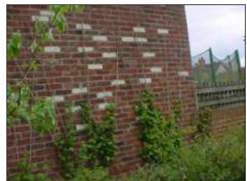
Plants on the brickwork
