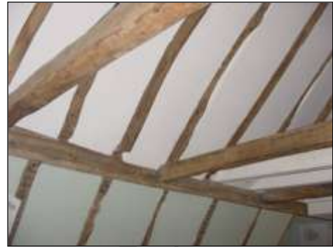
Timber frame structure.
