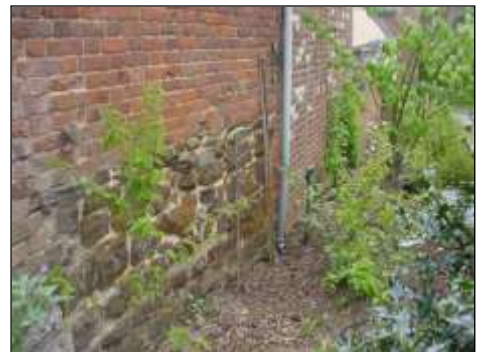
Rear of main building left hand side original sandstone
