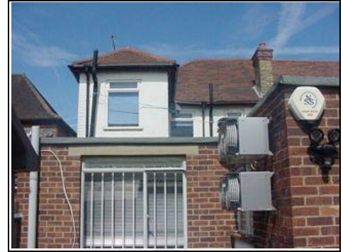
First floor level plastic window Ground floor level metal window
