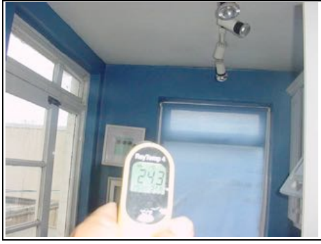
Surface temperature testing for condensation
