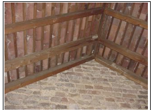
Underside of the roof tiles
