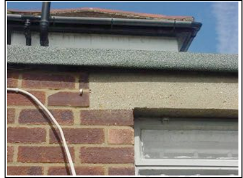
Concrete lintel to the rear
