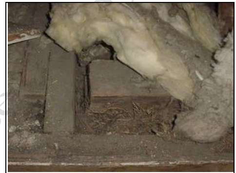
Insulation in roof
