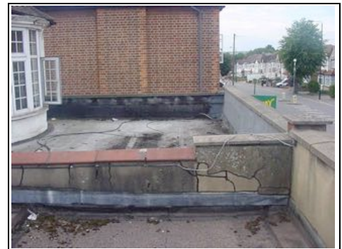
Flat roof to the front of the property
