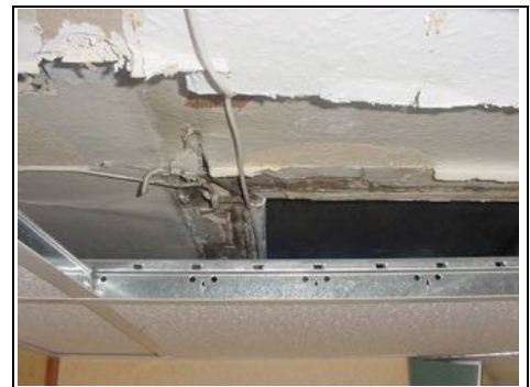
Close up of ceiling
