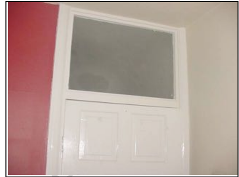
Door with glazing above on first floor
