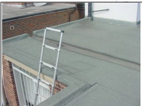
Left hand side view of rear flat roof
