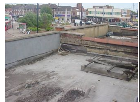
Front flat roof
