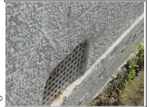
Render which is to ground level
