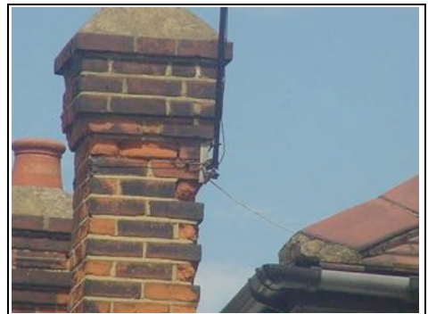
Close up of Chimney One
