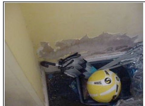
Skim coat over original lime plaster behind entrance door
