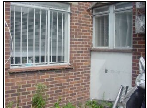
Bars to windows at ground level at the rear
