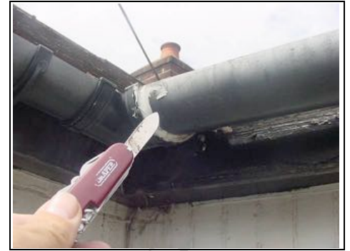
Close up of mastic repair
