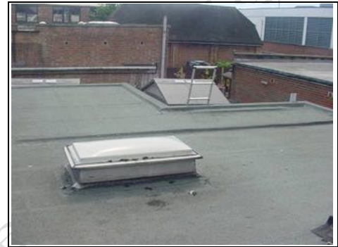
Rear flat roof
