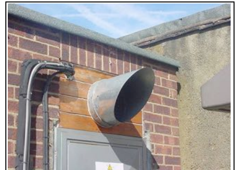
Flue at rear
