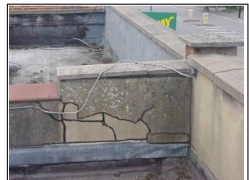
Rendering to parapet wall on neighbouring side
