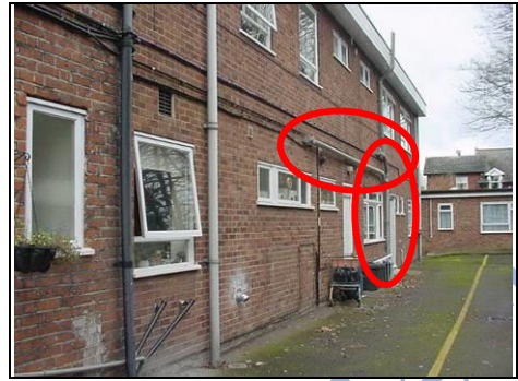
Long run to soil and vent pipes
