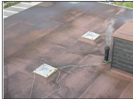
Middle of rear single storey flat roof Aerial view – 360 photo
