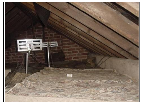
Hessian based bitumen membrane within rear roof
