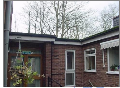
Stretcher bond brickwork to rear extension
