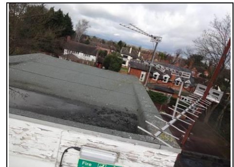
Roof over lift area Aerial view – 360 photo
