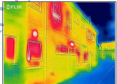
Heat coming through windows on right side of property
