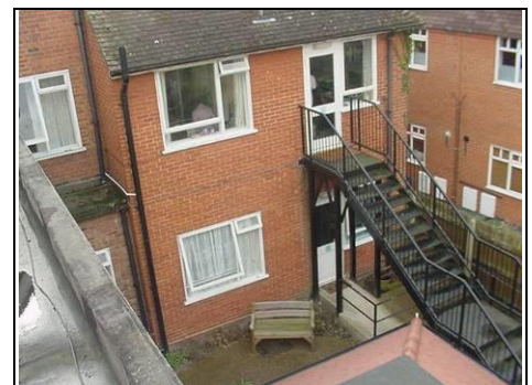
Rooms to the rear with a variety of different windows
