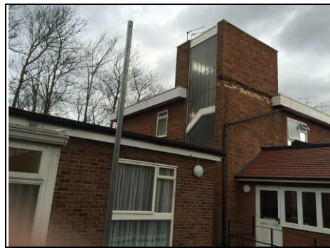
Lift tower and rear of two storey extension Aerial view – 360 photo
