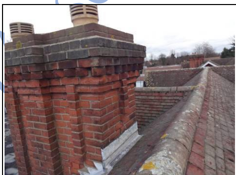
Trap behind rear left chimney Aerial view – 360 photo
