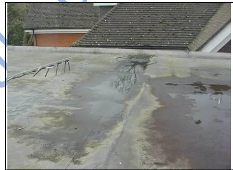
Two storey flat roof to left side
