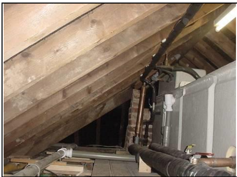
General view of left of rear roof
