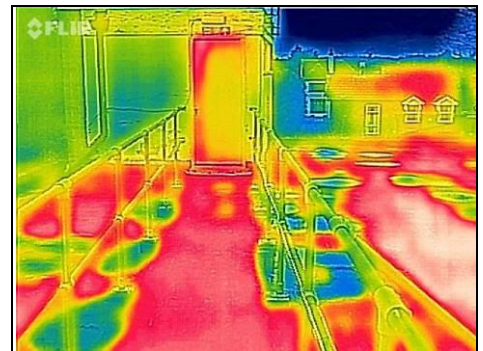
Thermal imaging looking towards lift area.
