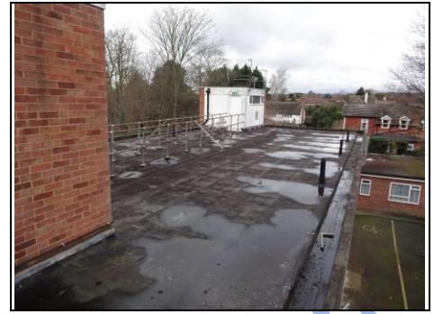
Two storey flat roof Aerial view – 360 photo
