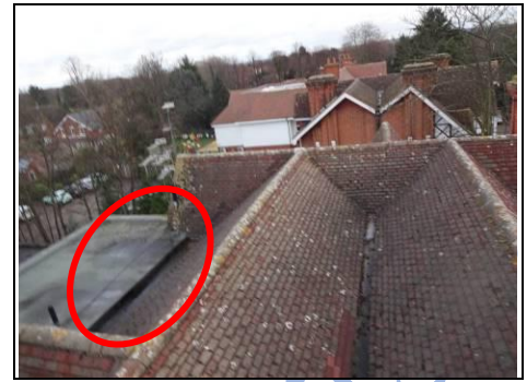
Rear box gutter Aerial view – 360 photo
