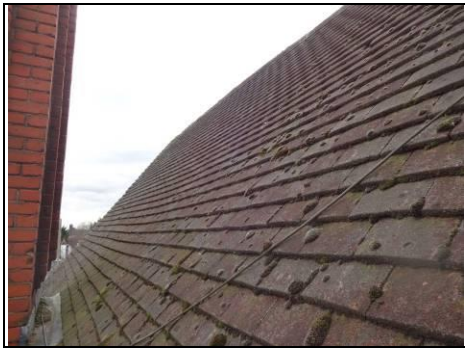
Close up of main roof tiles to right side
