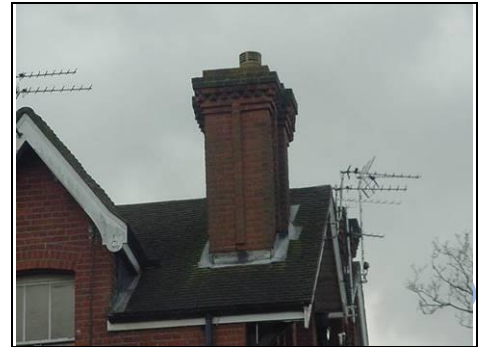
Rear left chimney
