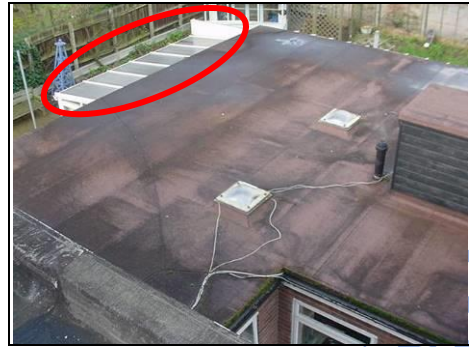
Rear glazed lean-to roof Aerial view – 360 photo
