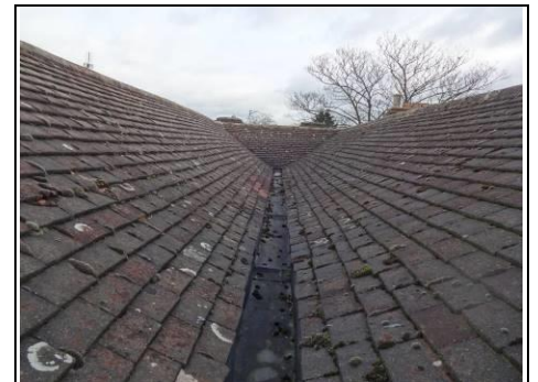
Hidden valley gutter on main roof Aerial view – 360 photo
