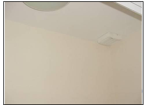
Small extract in one of the en-suite facilities
