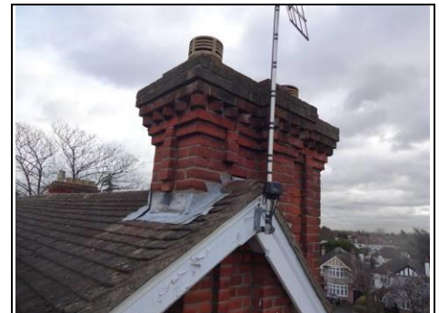
Front left chimney
