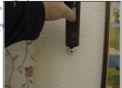
Dry lined walls in Room 20
