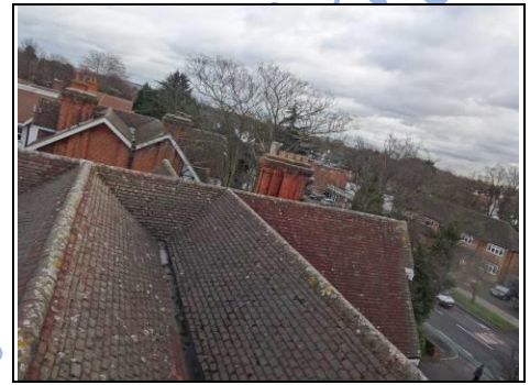
Main roof with hidden valley gutter
