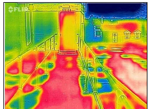
Thermal imaging looking towards lift area.
