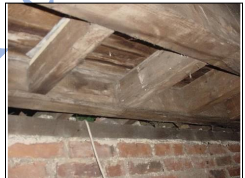
Timbers in front roof
