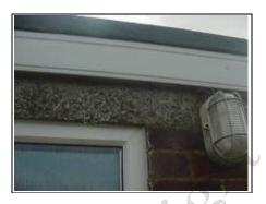
A close up view showing there is a concrete lintel over the door and window. This is where the cold bridging occurs causing condensation inside
