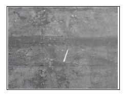
Cracking and crazing to the felt roof over the kitchen
