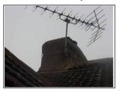
Chimney - left The cement flashing needs to be changed to lead flashing
