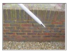
Step cracking in wall will need repairs.
