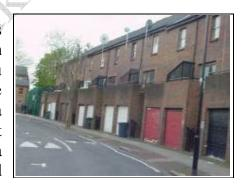
1960's properties built with concrete lintels that can cause **Cold Bridging**
