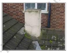
The rear chimney has a part lead flashing but needs to be all lead.
