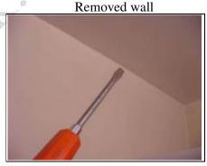
Cracking where the studwork wall in utility room meets the solid wall
