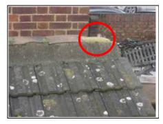
Missing tile on single pitch roof
