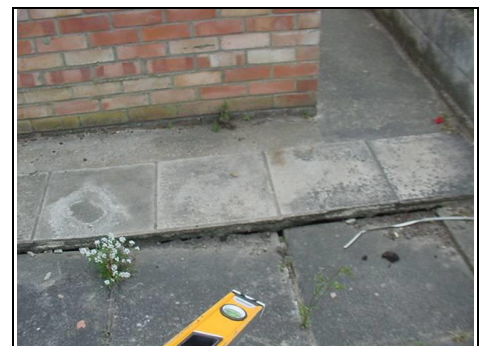
Movement to rear of property adjacent to boundary wall
