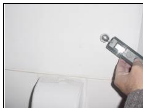
Testing for lateral dampness
