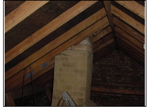
Timbers in main roof
