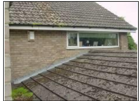
Concrete tiles to single storey pitched roof
