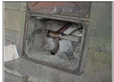
Manhole two middle left
