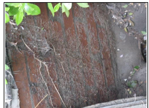
Manhole three front left
