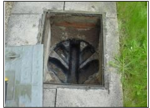
Manhole four front middle
