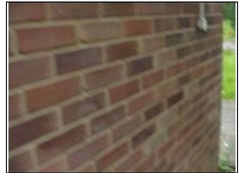
Stretcher bond brickwork
