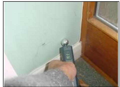
Testing for rising damp
