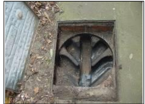
Manhole one rear left
