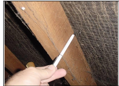
Close up of timbers
