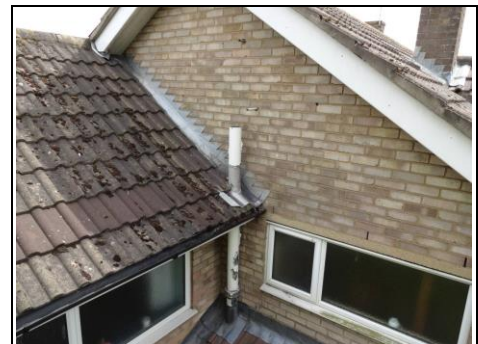
It may be an optical illusion but it does look like there has been some movement to the left gable.
