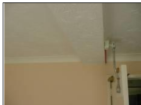
Chimney breast in bedroom six
