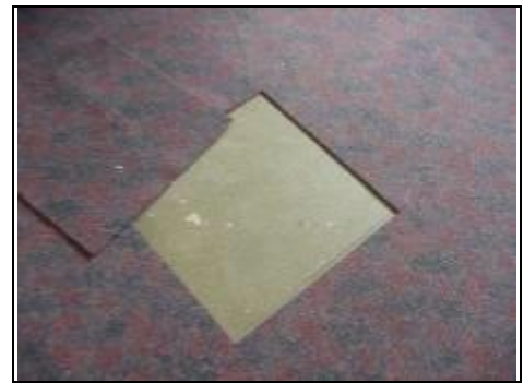
Timber decking indicating a suspended timber floor
