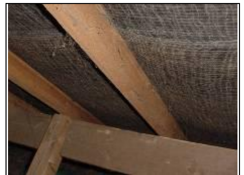
This photo shows the common rafters (the ones that form the pitch of the roof) and the dark area between is the underlayer.
