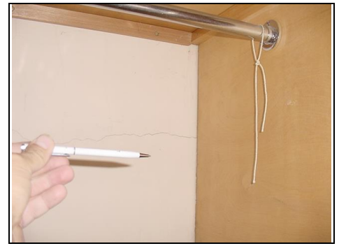
Hairline cracking
