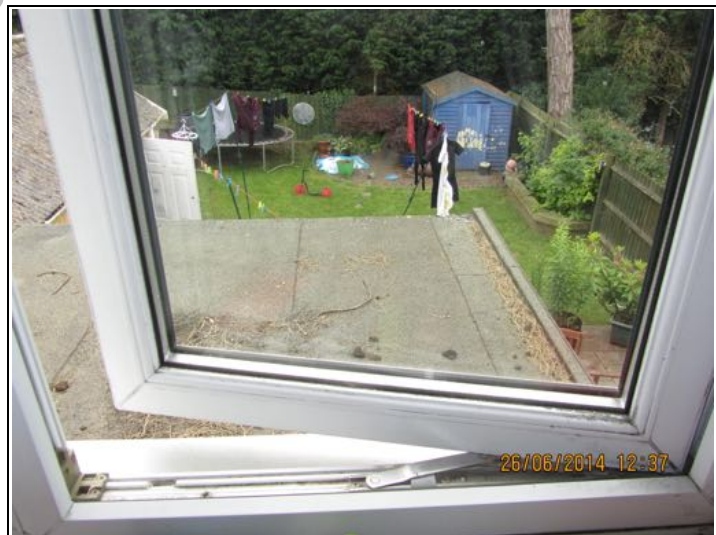
Rear Flat Roof over the Kitchen
