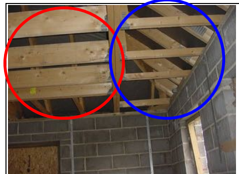
Example loft conversion Left side (red circle) floor rafters and right side (blue circle)
