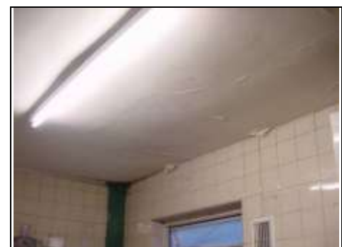
Dampness coming through from above in wash up area
