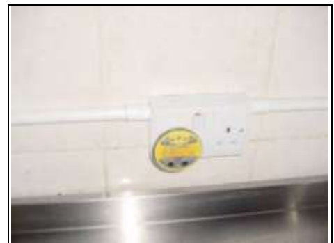
Earth test tripped both fuseboards
