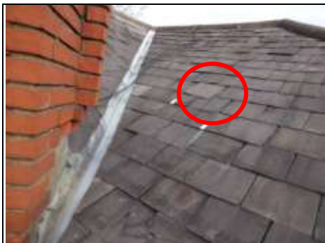
Slipped tiles on roof Aerial view -360 photo
