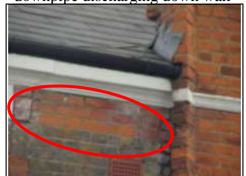
Dampness in the form of efflorescence on brickwork from overflowing gutter
