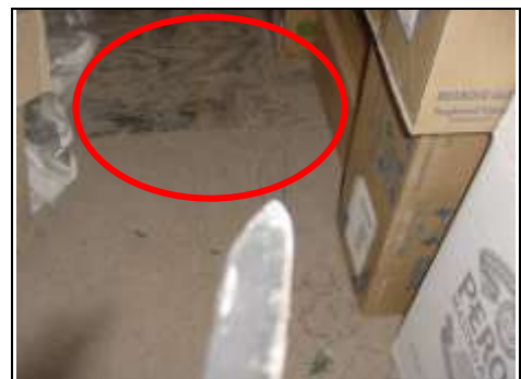
Staining to floor indicating rainwater coming in
