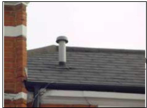
Soil and vent pipe
