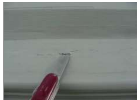
Signs of wet rot in timber windows
