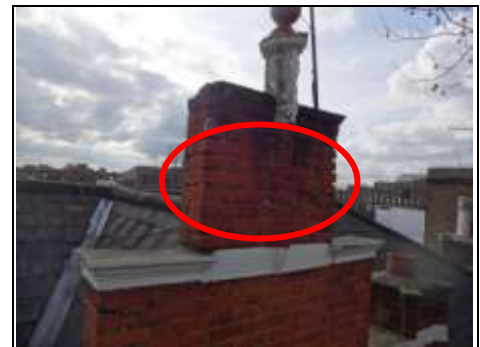
Deteriorating brickwork on the chimney Aerial view -360 photo
