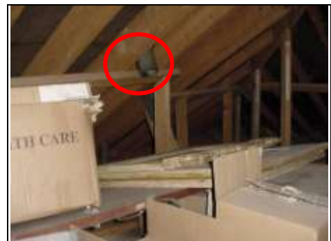
Vent not connected in roof space
