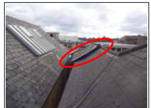
Flashband repairs on step in left side of roof
