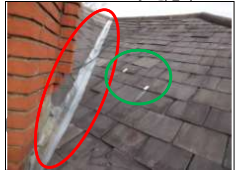
Rear valley gutter (red oval) and lead tingles (green oval) Aerial view – 360 photo
