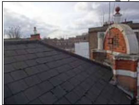
Back of corner chimney, Dutch gable and parapets Aerial view – 360 photo
