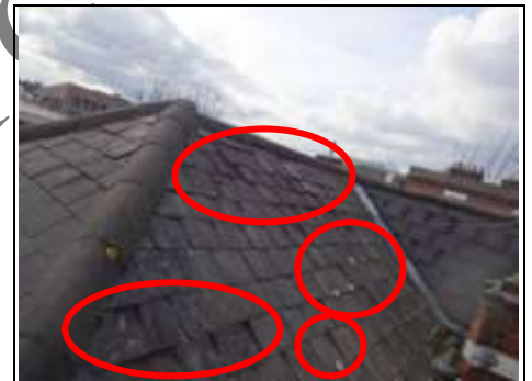
Slipped slates and lead tingles
