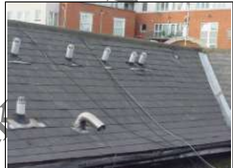
Numerous soil and vent pipes
