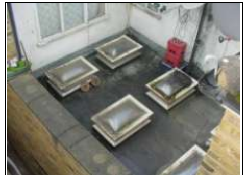
Flat roof with domed roof windows / sky lights, surrounded by parapet walls
