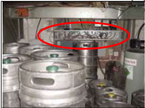
Cold store Wiring needs tidying up
