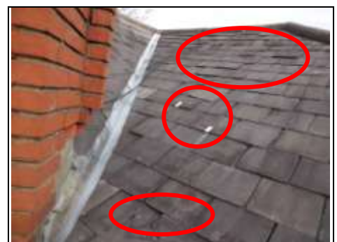
Old slates, with slipped, damaged slates and lead tingles Aerial view – 360 photo
