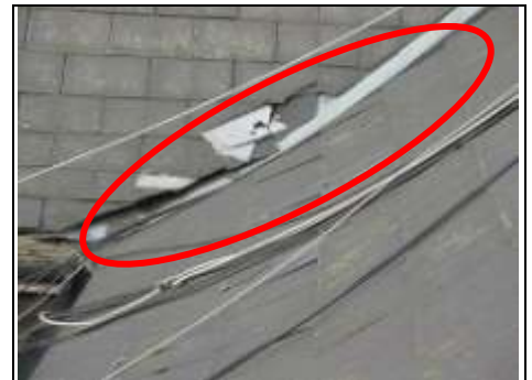
Rear valley gutter with damaged and slipped slates
