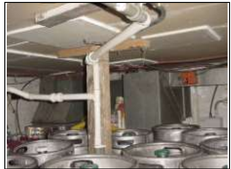
Drainage under bar needs supporting
