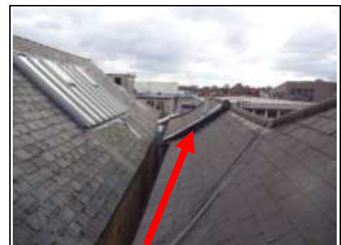
Flashband repairs on step in left side of roof Aerial view -360 photo
