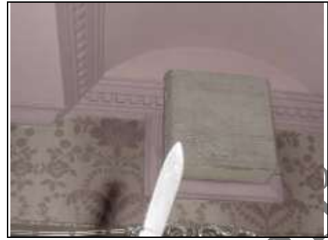
High level vent needs unblocking
