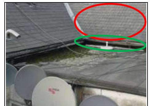
Dip in roof (red oval) with Flashband repairs below (green oval)
