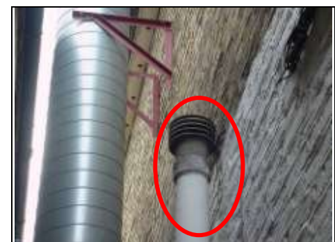
Flue may contain asbestos
