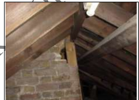
Chimney partially taken down visible within roof
