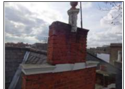
Chimney to right with soft red brick deteriorating and weathered pointing Aerial view – 360 photo
