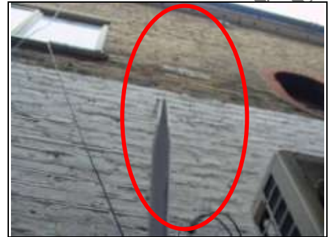
High level vertical cracking to left hand wall in passageway
