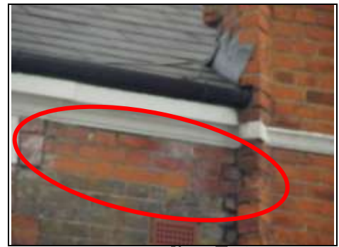
Dampness in the form of efflorescence on brickwork from overflowing gutter
