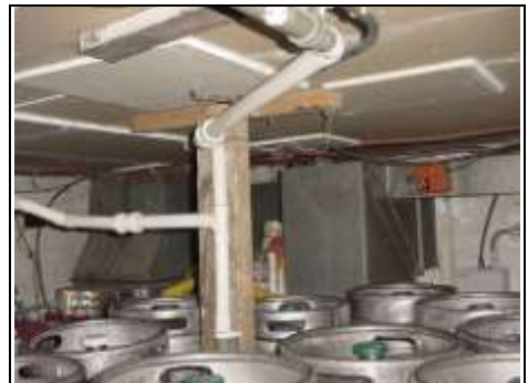
Drainage under bar needs supporting
