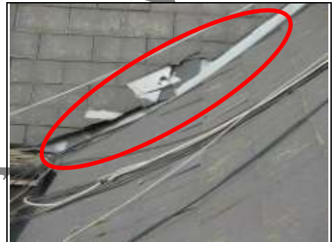
Problems with valley gutter
