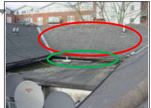
Dip in entire roof (red oval) with Flashband repairs below (green oval)
