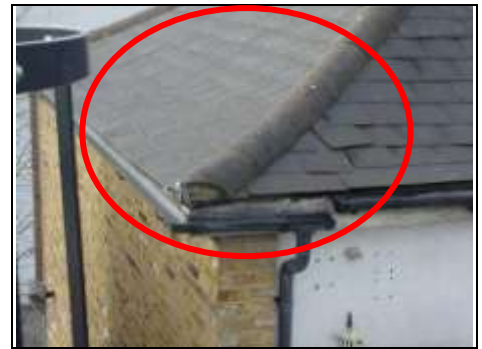
Rear right corner where there is some movement and whitening of slates
