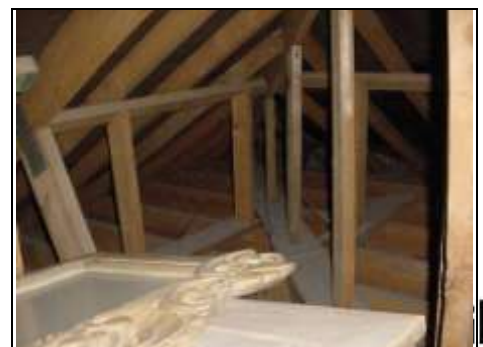
Props in roof space
