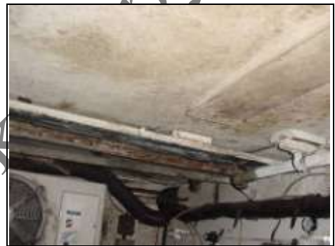
Mould to ceiling in cold store and rusting to supporting steels
