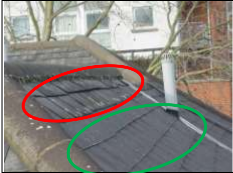
Original slate to top (red oval) Manmade slates below (green oval)
