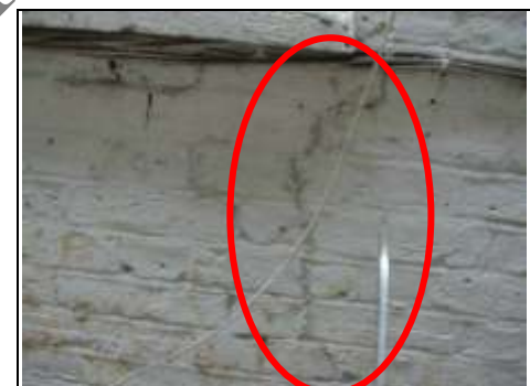
Vertical cracking to low level part of left hand wall
