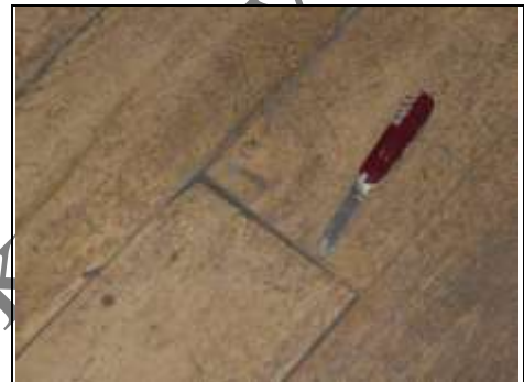
Bar boards screwed back down could relate to dampness and movement
