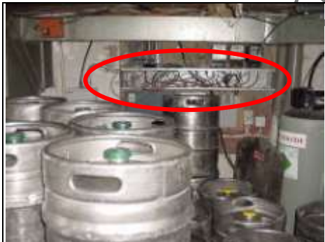
Cold store Wiring needs tidying up
