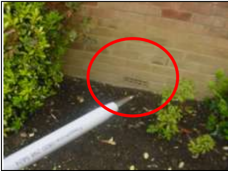
Airbrick acting as gutter
