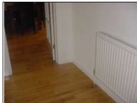
Unable to view floors
