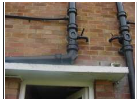
Soil and vent pipe to rear
