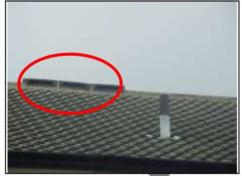
Vent to roof ridge
