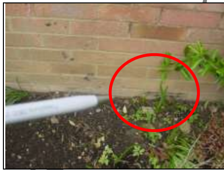
Airbricks acting as gutters
