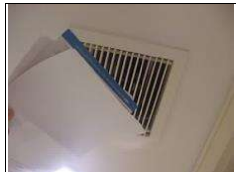
Poor extraction tested by using paper to see strength of extract fan
