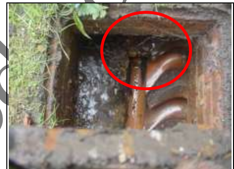
Roots in rear left manhole
