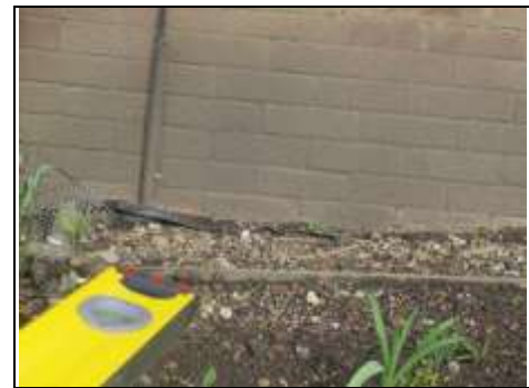
Rainwater hits the ground and bounces back onto the wall over the damp proof course
