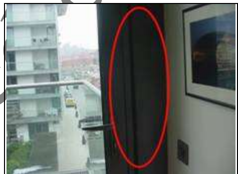
Flat with cold frame with condensation visible on the metal return
