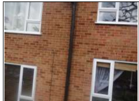
Stretcher bond brickwork
