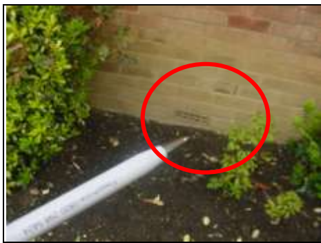
Airbrick acting as gutter
