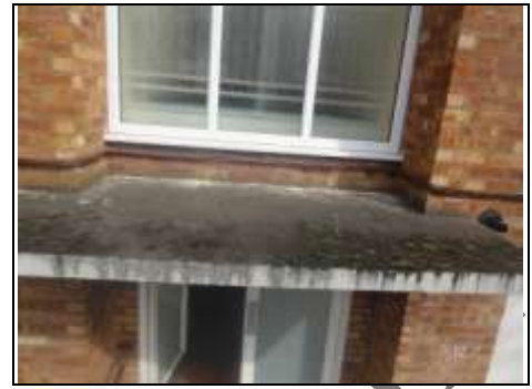
Moss to concrete roof of entrance canopy
