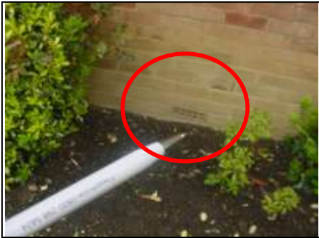
Airbrick acting as gutter
