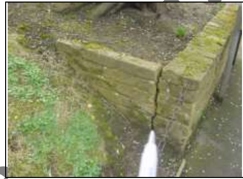
Tree causing damage to wall
