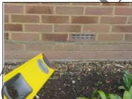
Damp proof course just below airbrick to front
