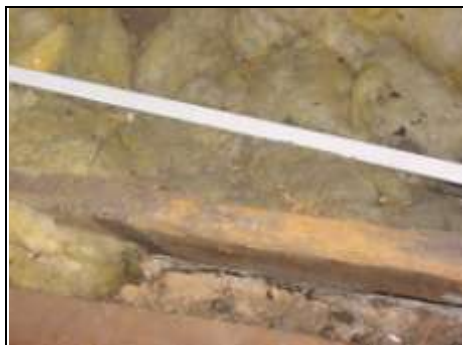
Woodworm in the roof
