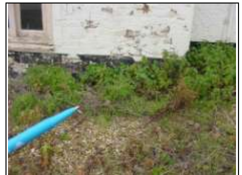
Ground level is high to front left
