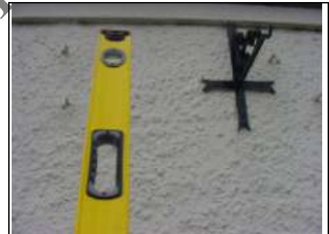
Crack and possible tie bar
