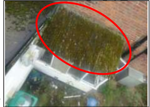
Asbestos roof to the rear entrance
