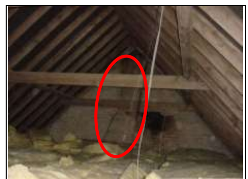
Crack on the front right, hidden within the function room roof
