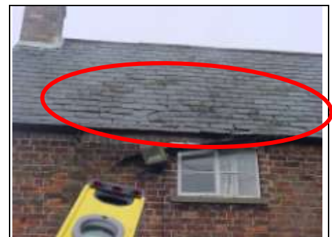
Slipped slates to the rear left
