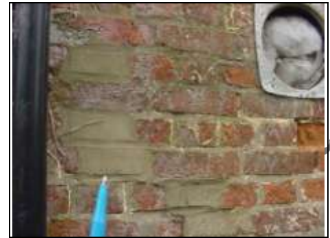
Ad-hoc pointing in cement mortar
