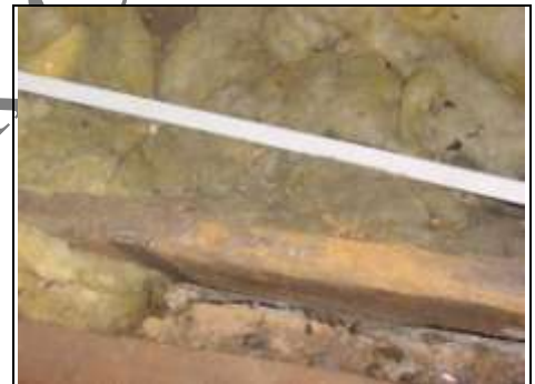
Woodworm in the roof
