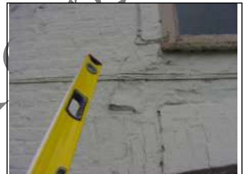
Cracking to the window
