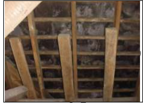
No protective underlayer to older style construction
