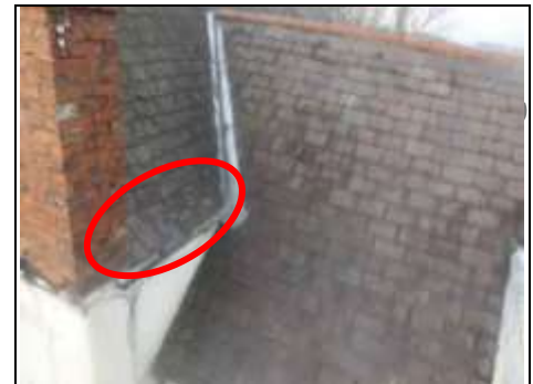
Slipped slates and lead tingles to the front right roof Aerial view – 360 photo
