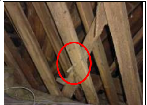
Peg fixings in the roof
