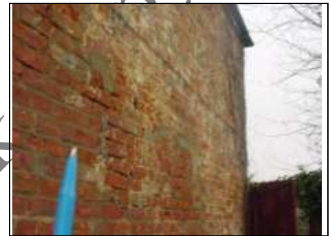
Whole bricks replaced with cement mortar
