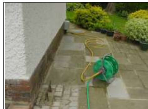
Weathering to brickwork
