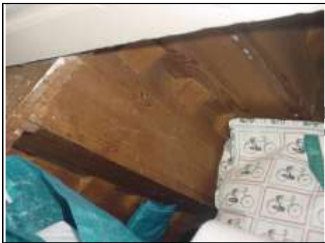
Underside of first floor to top floor staircase exposed
