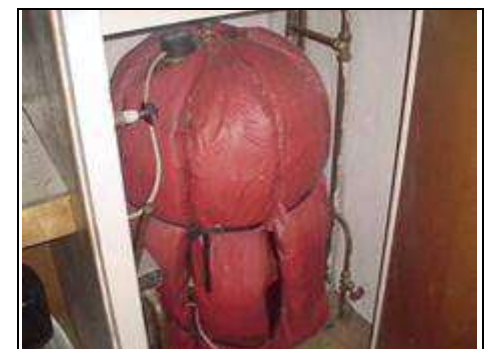
Older style cylinder with loose insulation jacket
