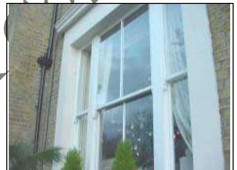
Sliding sash windows can swell in the winter months
