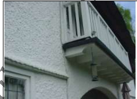
Close-up of drip detail above windows
