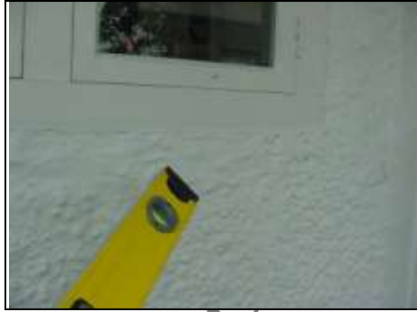
Undulations in the wall
