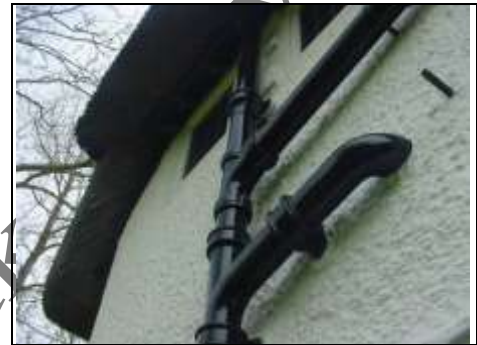
Soil and vent pipe
