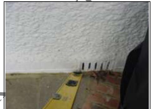
Airbrick acting as gutter
