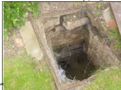
Tree roots in the manhole
