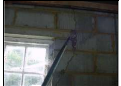
Cracking to rear wall
