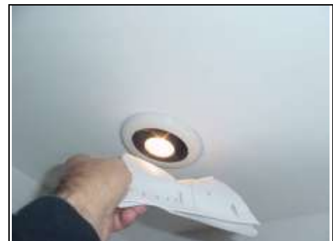
Checking the draw of the extract fan within the light
