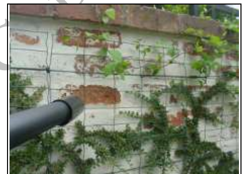
Spalling brickwork
