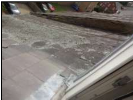
Deteriorating slates to right
