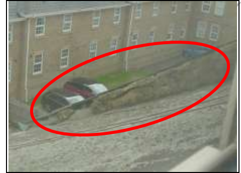
Step in roof viewed from rear window
