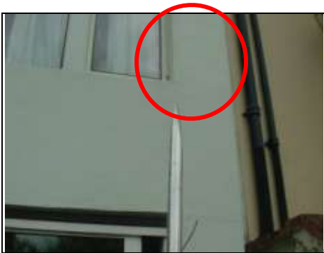
Vertical cracking
