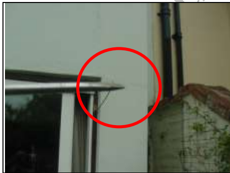
Horizontal cracking
