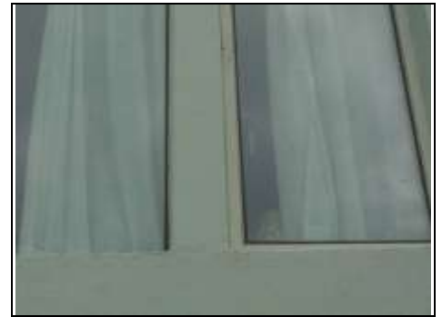
Repair around window area
