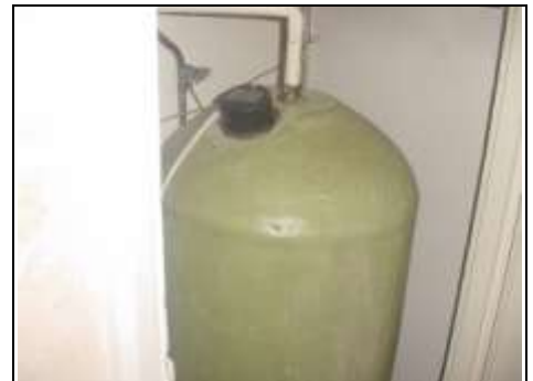
Modern items we often see in older properties factory insulated hot water cylinder
