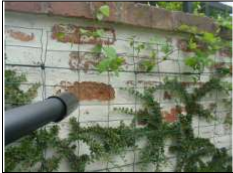
Spalling brickwork to rear garden wall
