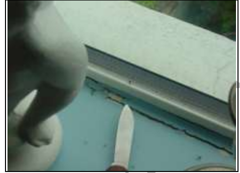
Cracking to box bay window sill on first floor rear window
