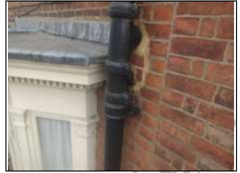
Cement mortar repairs
