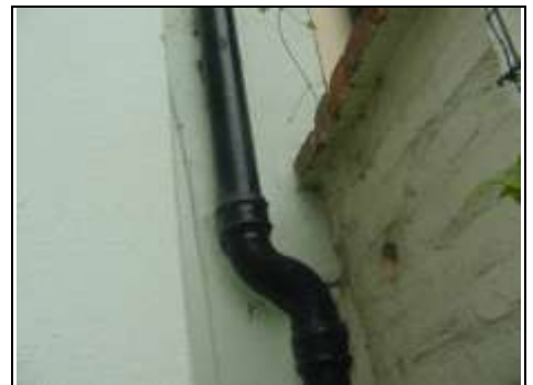
Possible rusting to cast iron
