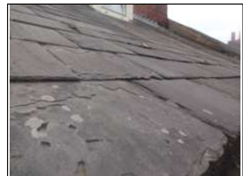
Deteriorating slates
