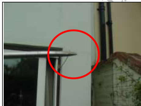
Horizontal cracking
