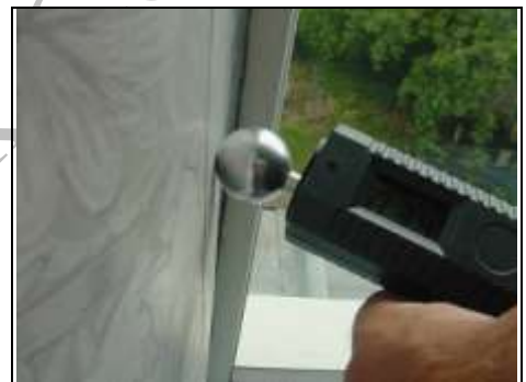
Lateral dampness in window reveal
