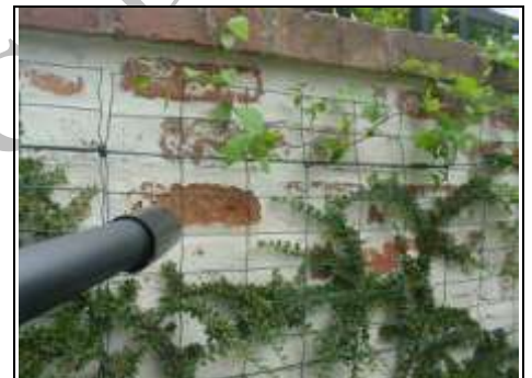
Spalling brickwork
