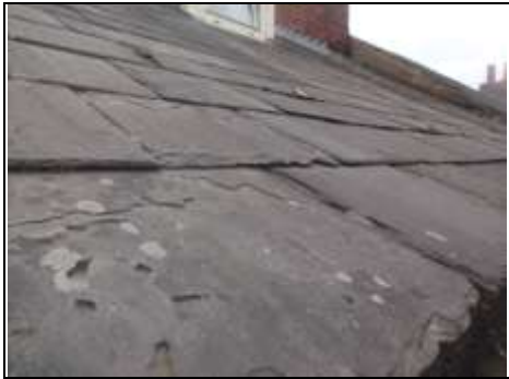
Deteriorating slates
