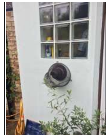
Flue for Baxi boiler
