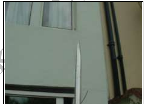
Hairline cracking to rear box bay indicating that render has got too high a cement content
