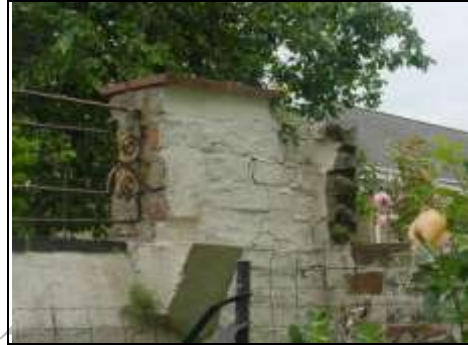
Rear right corner of garden wall needs repair
