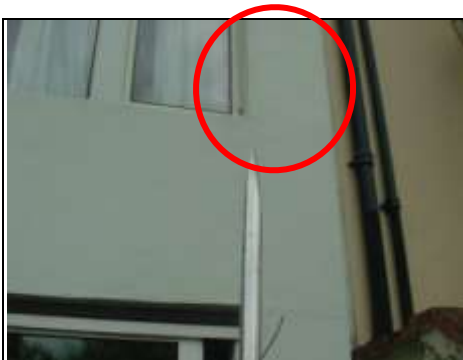
Vertical cracking
