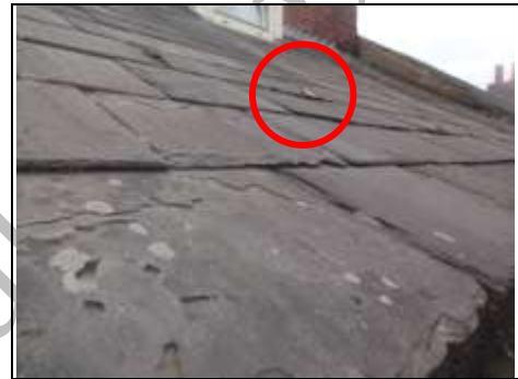
Deteriorating slates (tingle circled)
