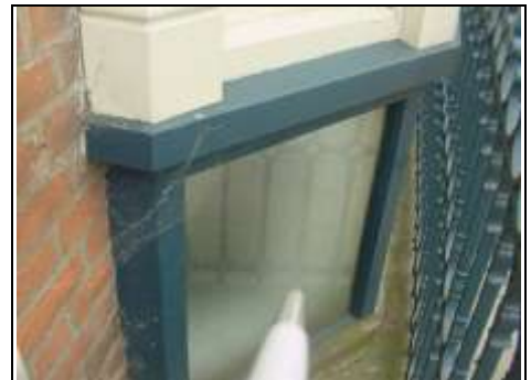
Glazed window to front not to listed building standard
