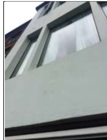
Repairs to render We would prefer a bell mouth detail here.
