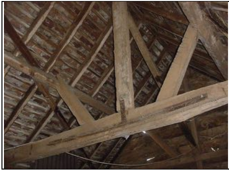
Kingpost truss roof of sorts stabilised with a metal brace
