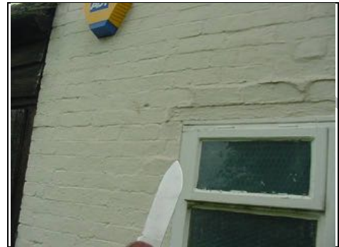
Window put in flush and timber lintel above
