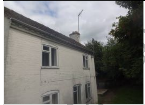
Rear of main house
