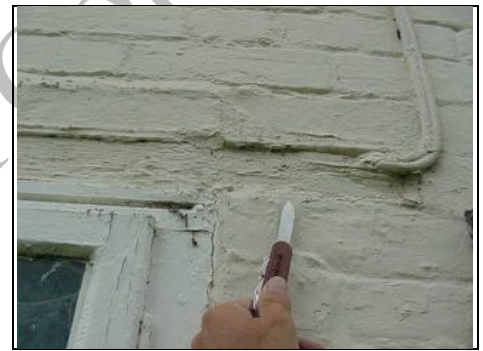
Timber lintel over front window
