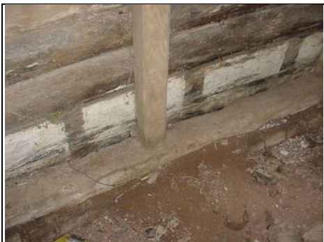
Sole plate and vertical timbers
