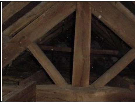
Kingpost truss roof
