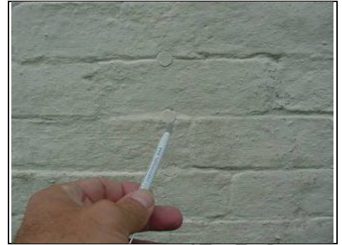
Chemical damp proofing
