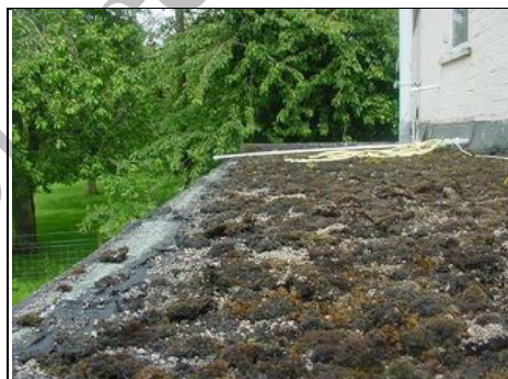
Moss to flat roof
