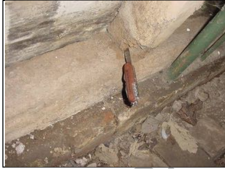
Base of vertical timbers
