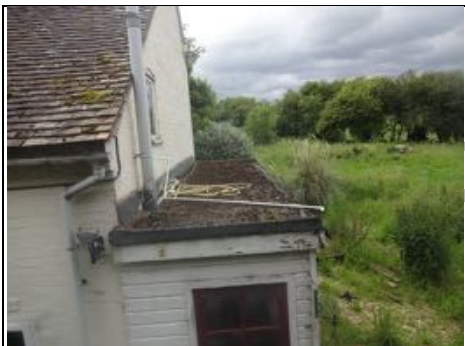
Flat roof to porch on right
