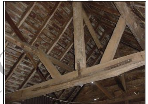
Barn has medieval style kingpost truss of sorts stabilised with a metal brace
