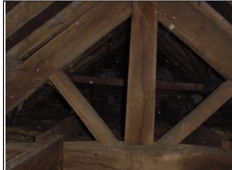
King post roof of main house
