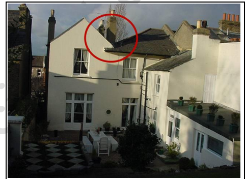
Circle shows where roofs meet and form valley gutter.
