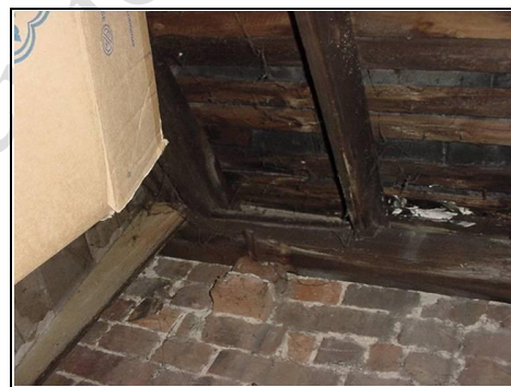
Rear Left hand side roof showing damp getting in.
