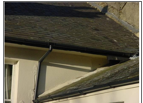
Main slate roof joining rear roof
