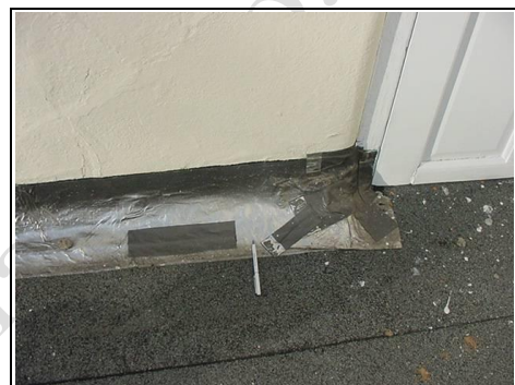
Close up Flashband repairs with concrete roof in view
