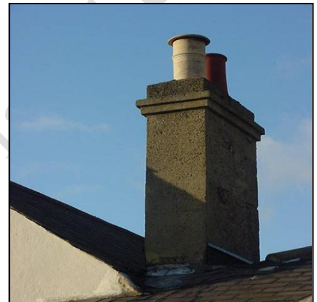
Weathered render on chimney
