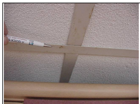
Dampness has come through as shown by the rust on the suspended ceiling system
