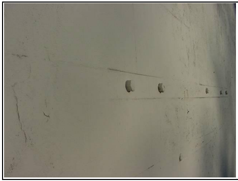
Strapping to rear parapet wall
