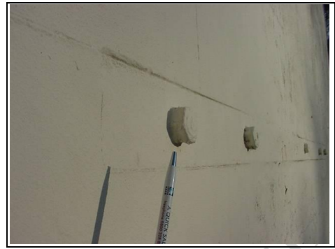
Strapping to parapet close up
