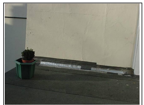
Repaired flashing
