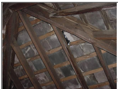
Front Left hand side roof showing dampness getting in.
