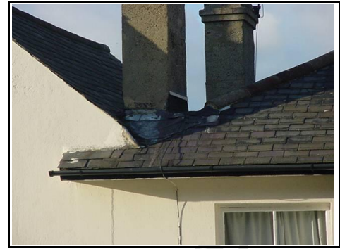
The two centre chimneys sitting in the valley gutter
