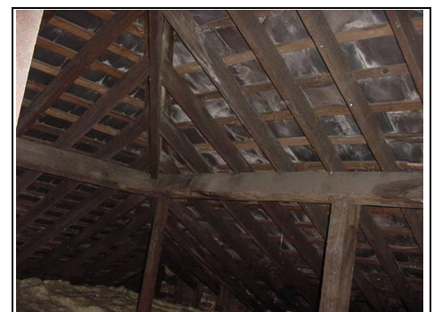
Dampness visible to the timbers. The darker areas are dampest.
