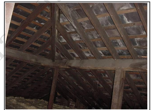
No protective underlayer and dampness getting in
