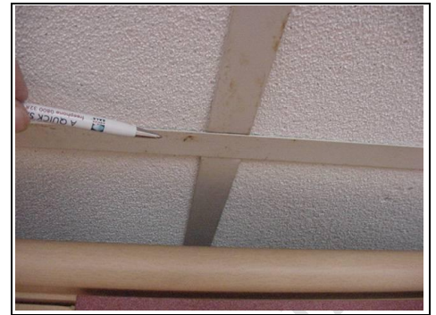
Rust on ceiling system
