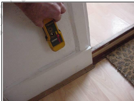
Dampness found in dining room due to the ground levels
