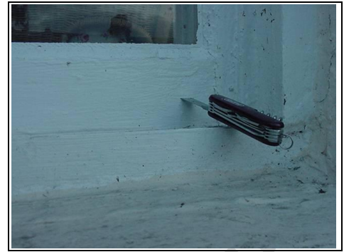
Rotten timber knife test
