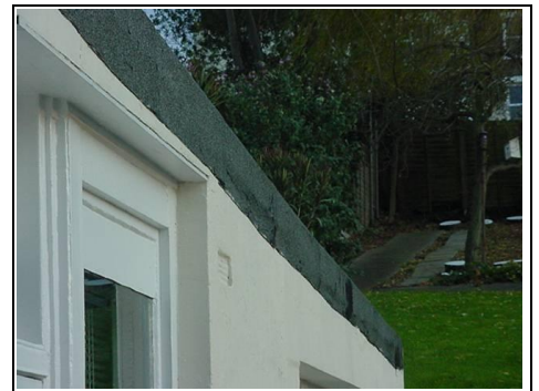
Flat roof with no gutter
