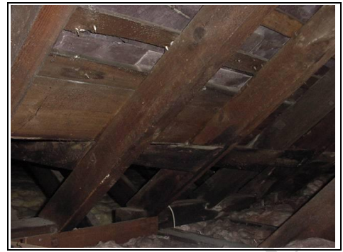
Close up of the valley gutter showing dampness in the timbers
