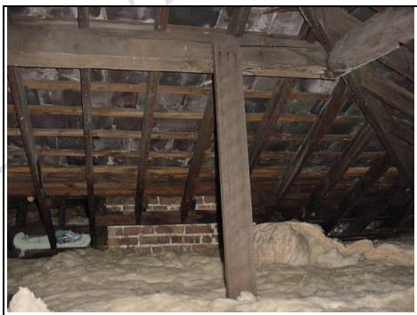
Dampness and condensation in the timbers
