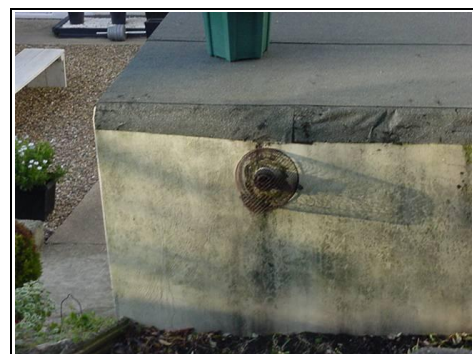
No guttering to the rear of the kitchen roof
