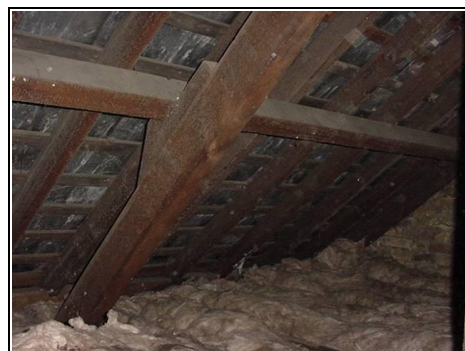
Looking at the roof to the right hand side with mould on the timbers.
