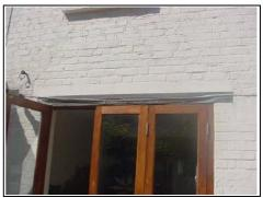
Movement visible above the door – stepped diagonal pattern from the lintels. Also drip detail needs to be improved and / or the doors set within the frame and a vertical damp proof membrane added.
