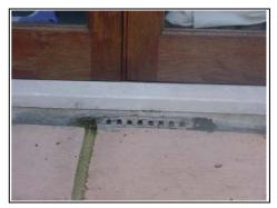
Blocked airbricks to suspended timber floor
