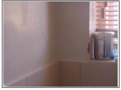
Diagonal cracking to bathroom wall
