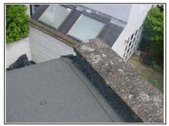
Small lip to the parapet wall at the end of the flat roof does not resolve the problem of rainwater discharging down the length of the left hand wall. A proper drip needs to be formed.
