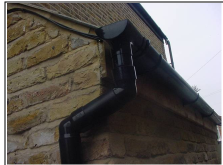
Fascias and soffits not painted to the left hand side
