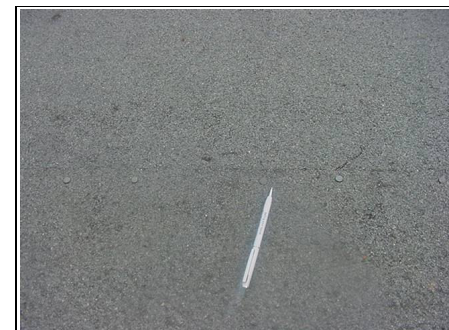
Nails to rear flat roof over kitchen
