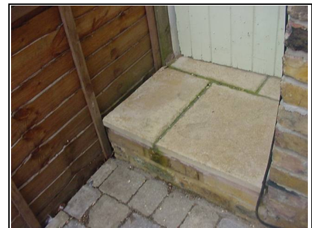
Water staining on the steps due to a leaking/surcharging gutter
