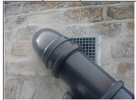
Extract from bathroom covered by seal and vent pipe
