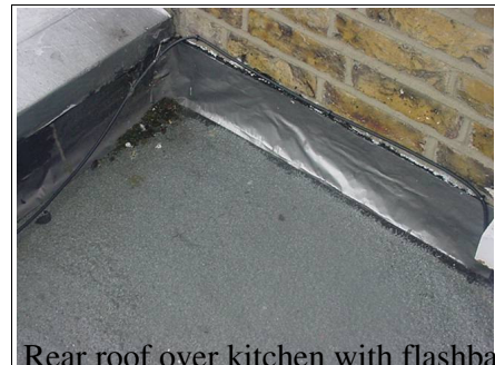
Rear roof over kitchen with flashband
