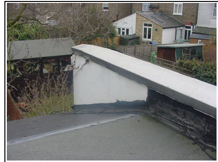
Flashband on parapet wall which is not ideal
