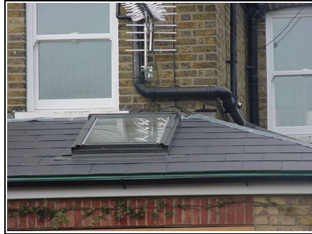
Awkward soil and vent pipe
