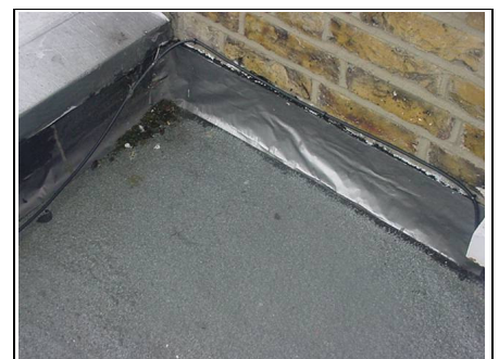
Flashband to rear flat roof
