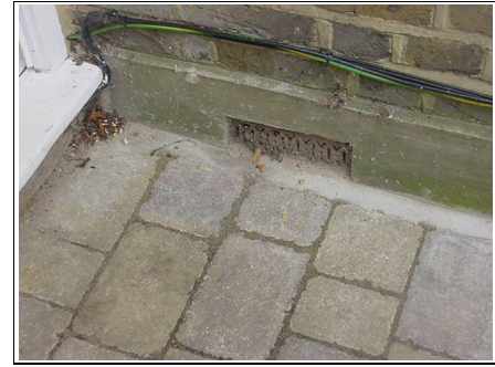
Airbrick acting as a gutter next to the door
