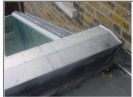
The original coping stone has been completely covered in a flashband.
