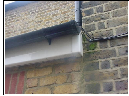
Overflowing gutter
