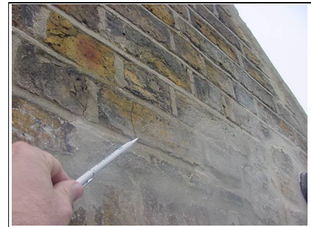
Hairline cracking to rear of prop above bathroom window
