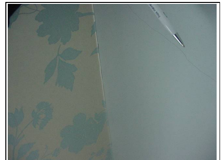
Hairline cracking to plaster
