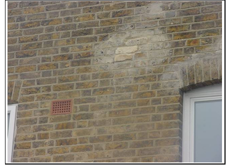
Next doors air vent and you air vent covered up
