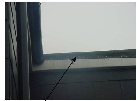
Nailing of main flat roof
