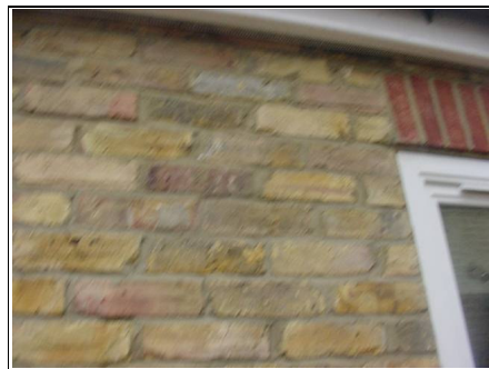
Stretcher bond brickwork to extensions
