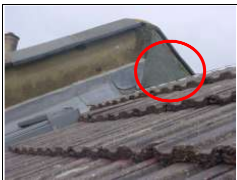
Felt flashing
