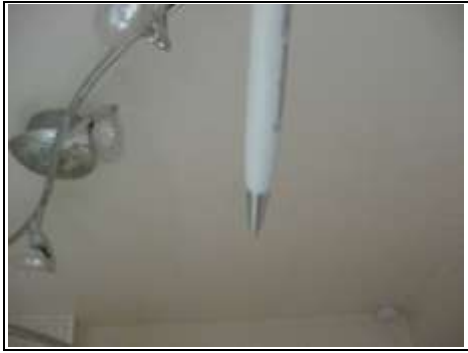
Straight line crack to bathroom ceiling
