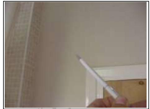
Diagonal crack in bathroom which is a structural crack
