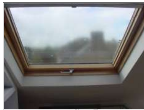
Misting of roof window
