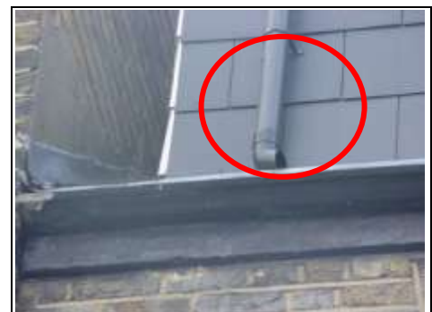
Downpipe causing overflow
