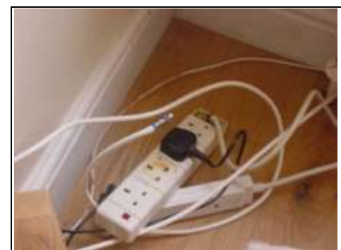
Extension leads were noted, more electric points required 25
