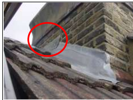
Felt flashing
