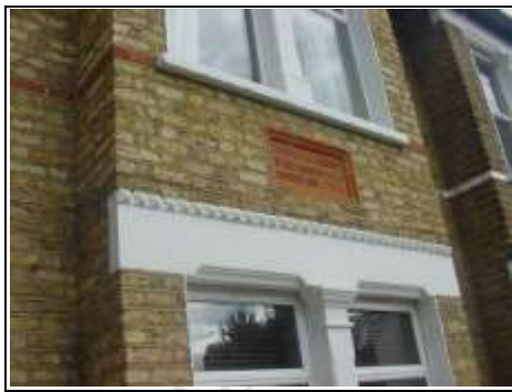
Brickwork to front was previously rendered
