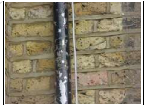
Surface of bricks sanded or sand blasted, possibly damaged when the render was taken off which means they will deteriorate more quickly
