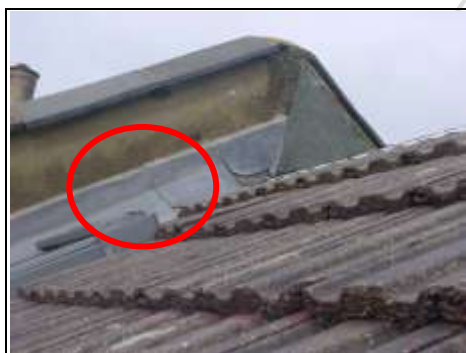
Close up of flashings (tile on edge with a covering of lead)
