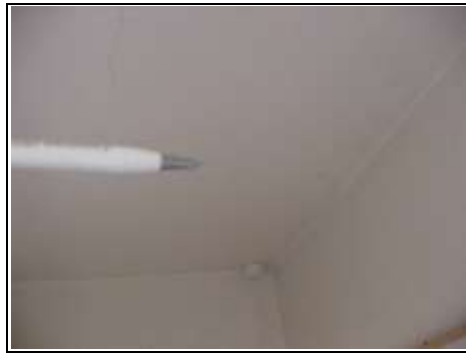
Other straight line crack to bathroom ceiling
