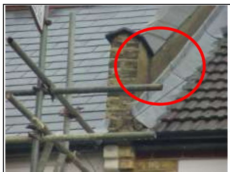
Left hand parapet wall with original tile on edge and then lead over the top
