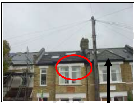
Flat roof to front box bay – you can see pitched roof to adjacent property
