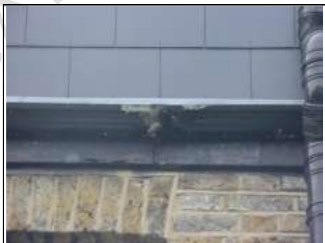
Gutter to rear which isn't coping, looks to be cast iron
