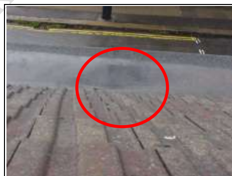
Ponding to bay window roof
